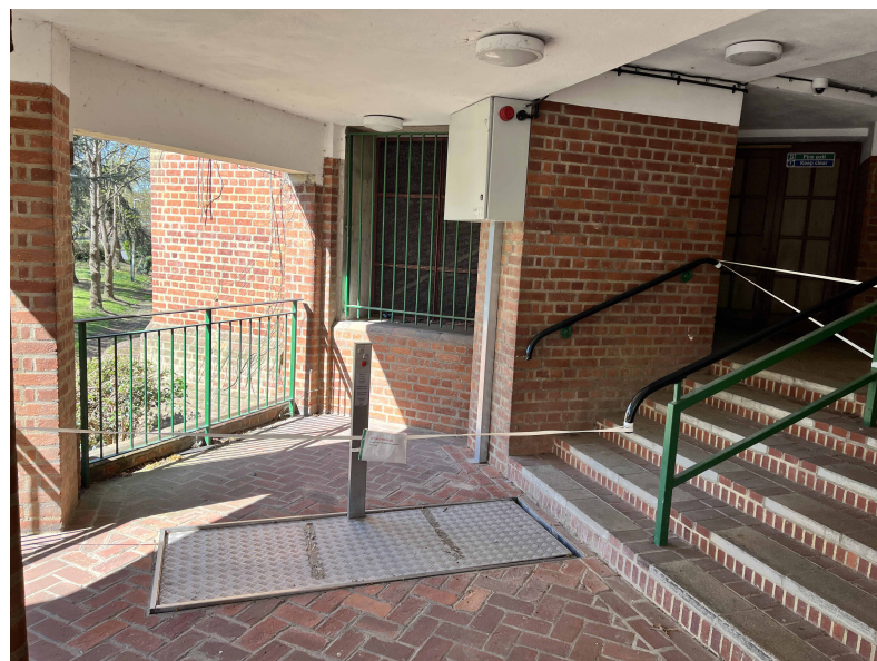
View of the existing platform lift (out of service).
