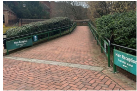
View of the existing Ramp
