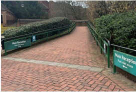
View of the existing Ramp
