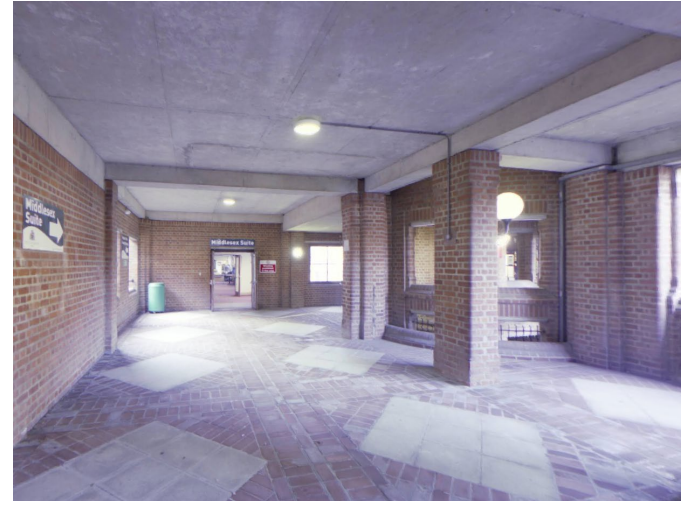
Covered walkway and Middlesex Suite entrance door
