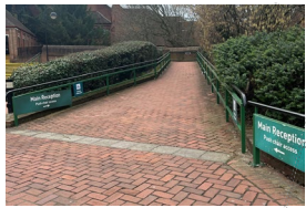
View of the existing Ramp
