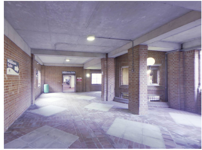
Covered walkway and Middlesex Suite entrance door
