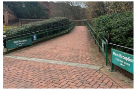
View of the existing Ramp
