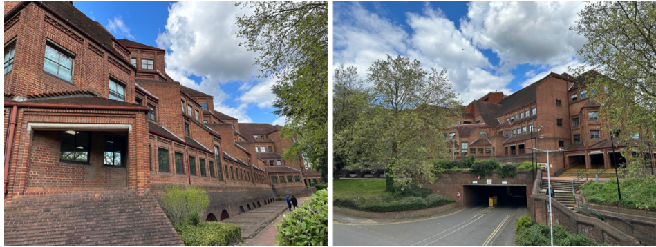
Figures 6&7: The semi-basement and cascading bays
