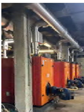
Figure 7. Existing gas fired boilers
