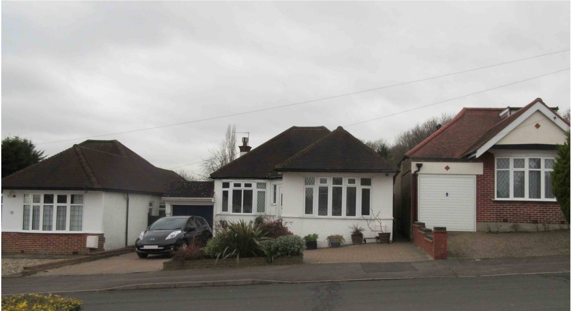
Front, 5 Hillside Crescent:
