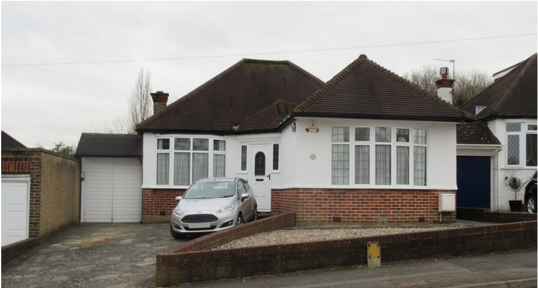
Front, 3 Hillside Crescent:
