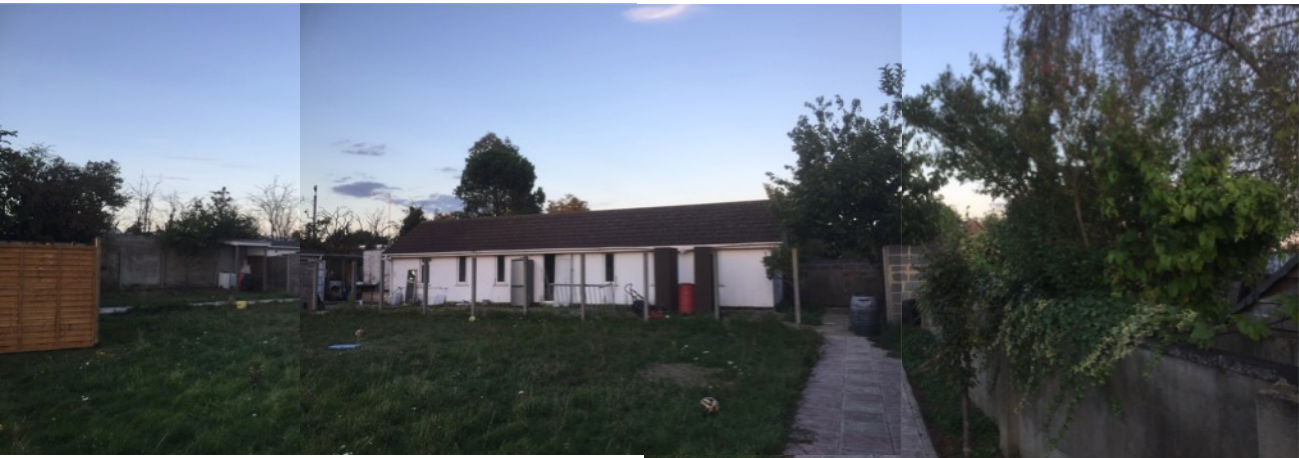
Views from rear garden looking towards the outbuilding and rear boundary
