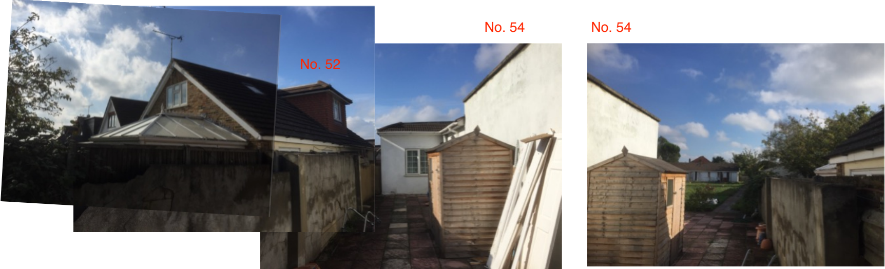
Views from the patio looking down the side of the property adjacent to no. 52
