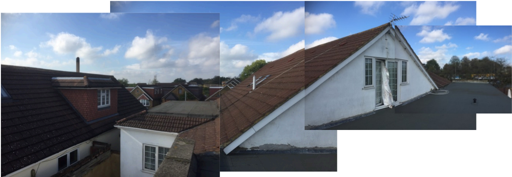
Views of the roof from the existing flat roof extension
