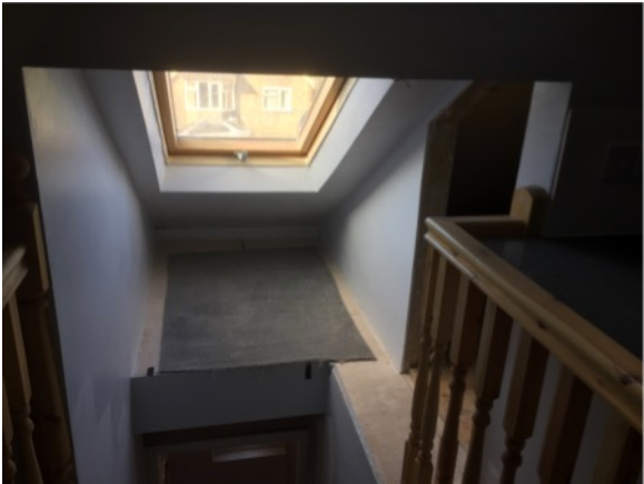
Area of storage and skylights above the staircase
