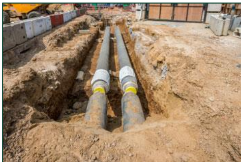
Figure 6. District heating pipework 3
