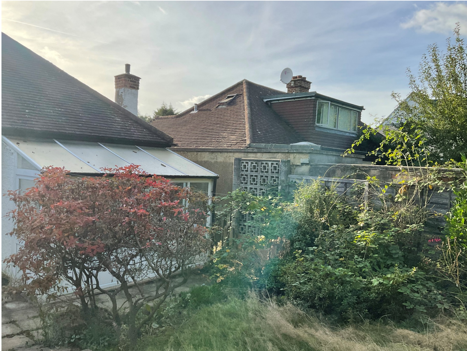
SITE PHOTOS: 75, Hillside Road, Northwood, HA6 1PZ
