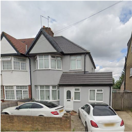
7. No.29 Dawley Avenue opposite No.28
