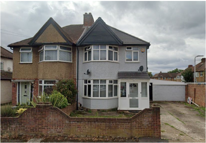
2. Front view of No. 30 and 28 Dawley Avenue
