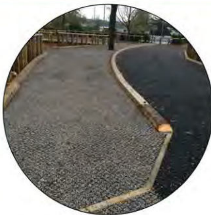
Backfilled with gravel
