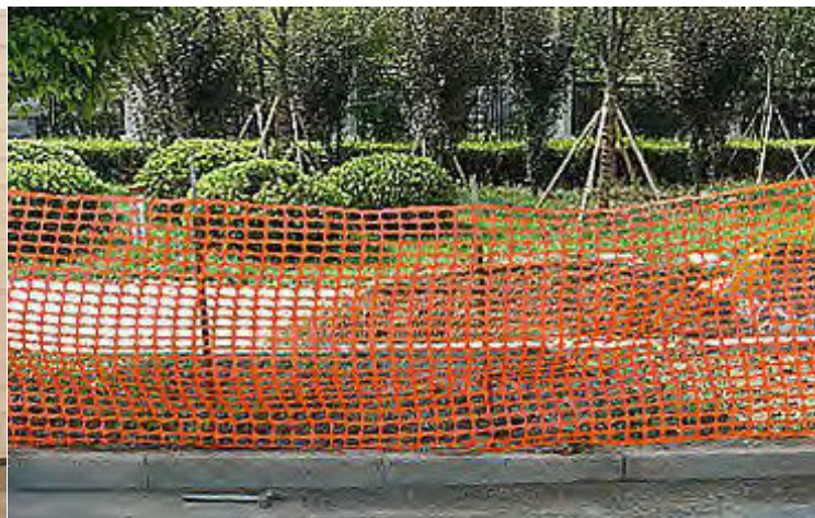
Plastic mesh fencing held in place with road pins.
