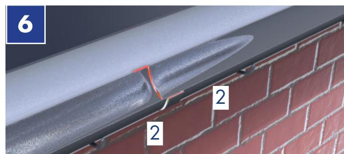
Finally, cone off the exposed bolt stud and nut inside the gutter with a generous application of silicone around the joint and from external surfaces.
