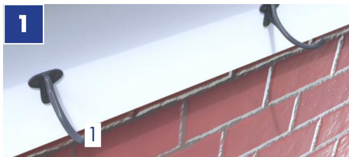
Using a straight edge or ruler, shim gutter brackets with 5mm clearance so that the last roof tile or slate will align with the midpoint of the gutter.
