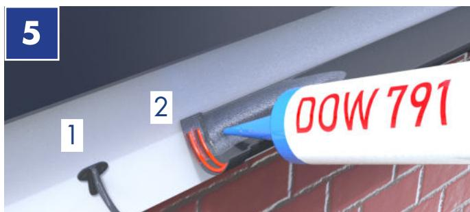
Apply two 6mm beads of DOW 791 silicone sealant either side of, and around the fixing hole.
