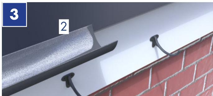
Lower the gutter onto the brackets ensuring sufficient clearance for the gutter joint. Clip gutter into bracket.
