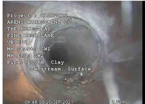
SW1X_a436c66e-90db-4588-be63-e4759c3dcd45_20210927_085154_178.jpg, 00:00:03, 0.93 m Junction at 9 o'clock, diameter: 100mm
