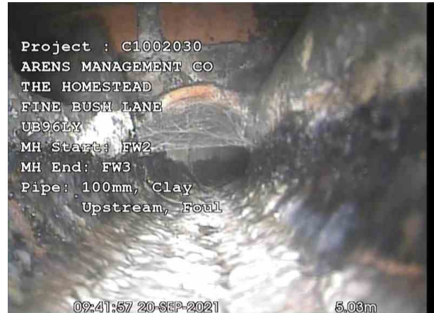
FW3X_81cebaaa-2ead-4f30-8e9a-0c4d51c9ed1c_20210927_083037_889.jpg, 00:00:18, 5.03 m Finish manhole, FW3, the pipe is flowing fine
