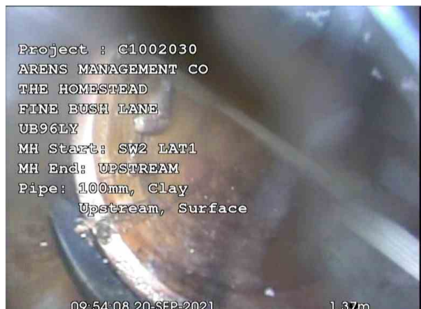
UPSTREAMX_ca45a53c-90f5-460b-8fe8-f028685f26c1_20210927_085334_124.jpg, 00:00:09, 1.37 m Finish connection without manhole, UPSTREAM, the pipe is flowing fine
