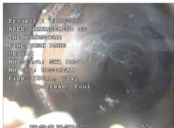
UPSTREAMX_47231b34-8d51-4185-992f-fbf23499fc12_2021 0927_083514_725.jpg, 00:00:06, 1.87 m Junction at 3 o'clock, diameter: 100mm
