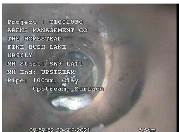
UPSTREAMX_b41d7a84-b3d3-48d2-8f29-3671441025e3_202 10927_085013_339.jpg, 00:00:13, 7.66 m Junction at 3 o'clock, diameter: 100mm
