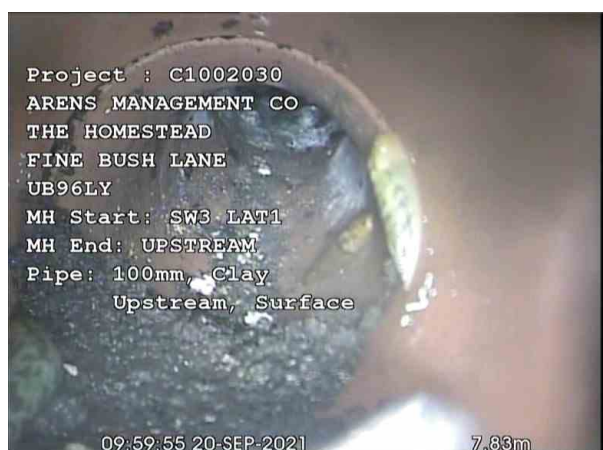
UPSTREAMX_54f6bd31-f753-4e34-9378-9c2c8bece954_202 10927_085033_624.jpg, 00:00:16, 7.83 m Finish connection without manhole, UPSTREAM, the pipe is flowing fine
