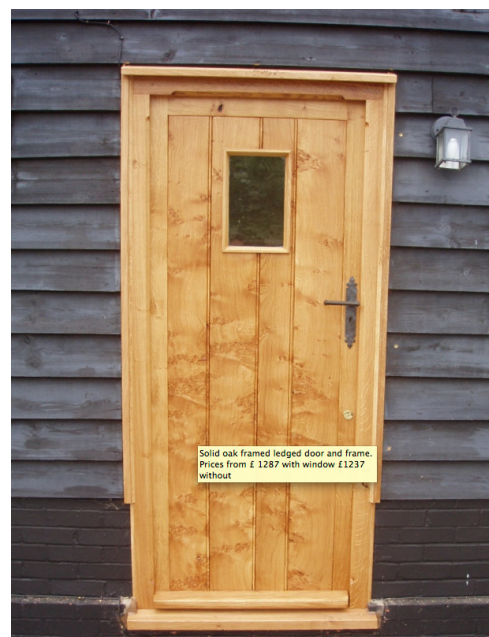
A typical door set within the feathered edge boarding
