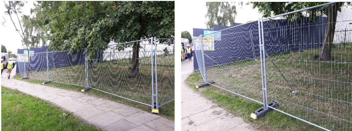
Photos above show protective fencing installed as per BS5837:Fig 3A with rubber feet and stabilizer struts.
