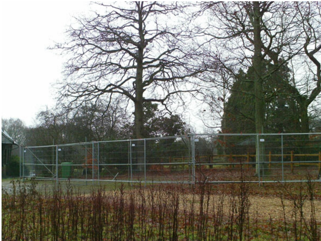
Protective fencing with stabilizers as per fig 3 (a).
