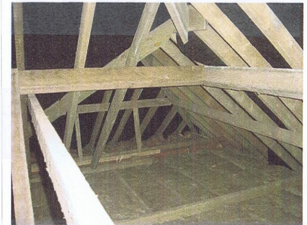
view into front bay (loft).
