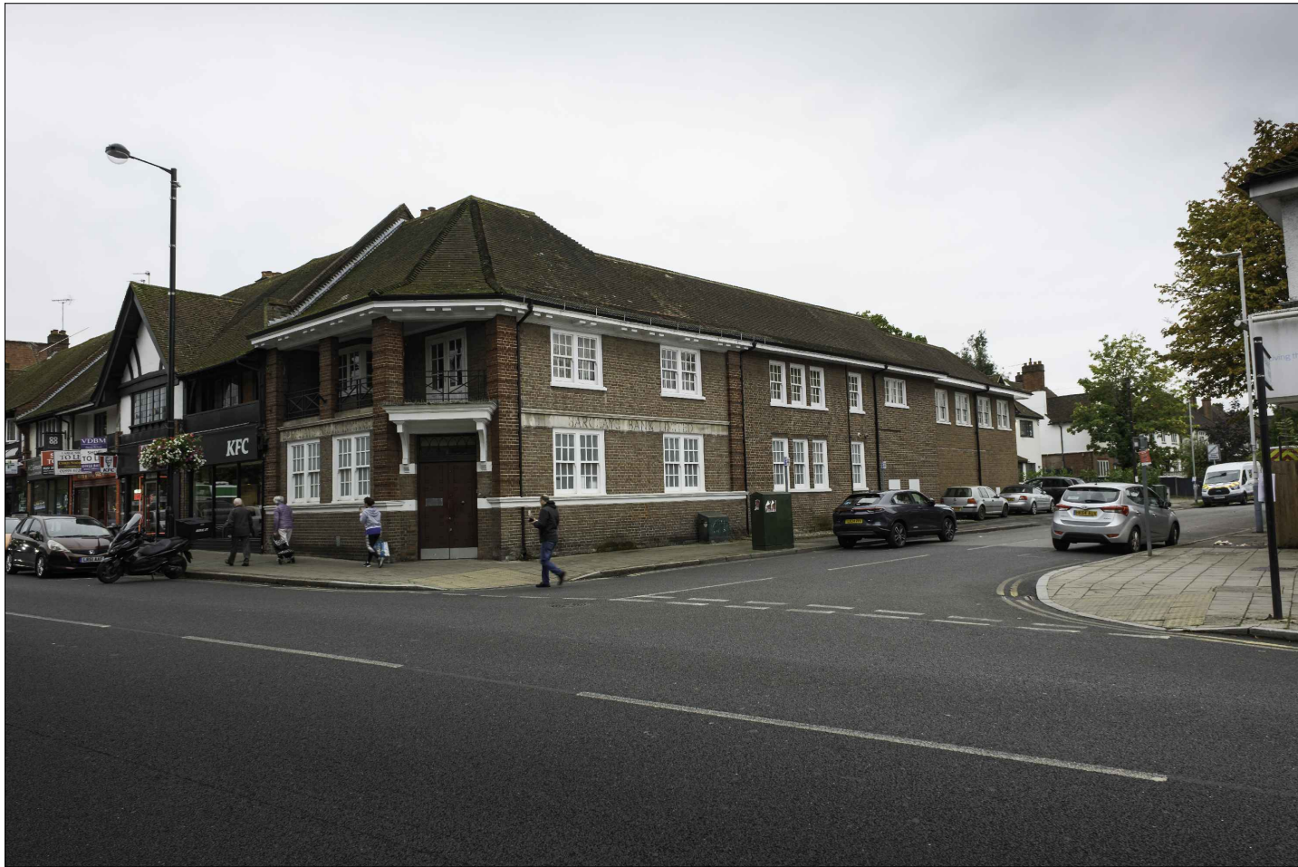
EXISTING VIEW FROM HIGH STREET
