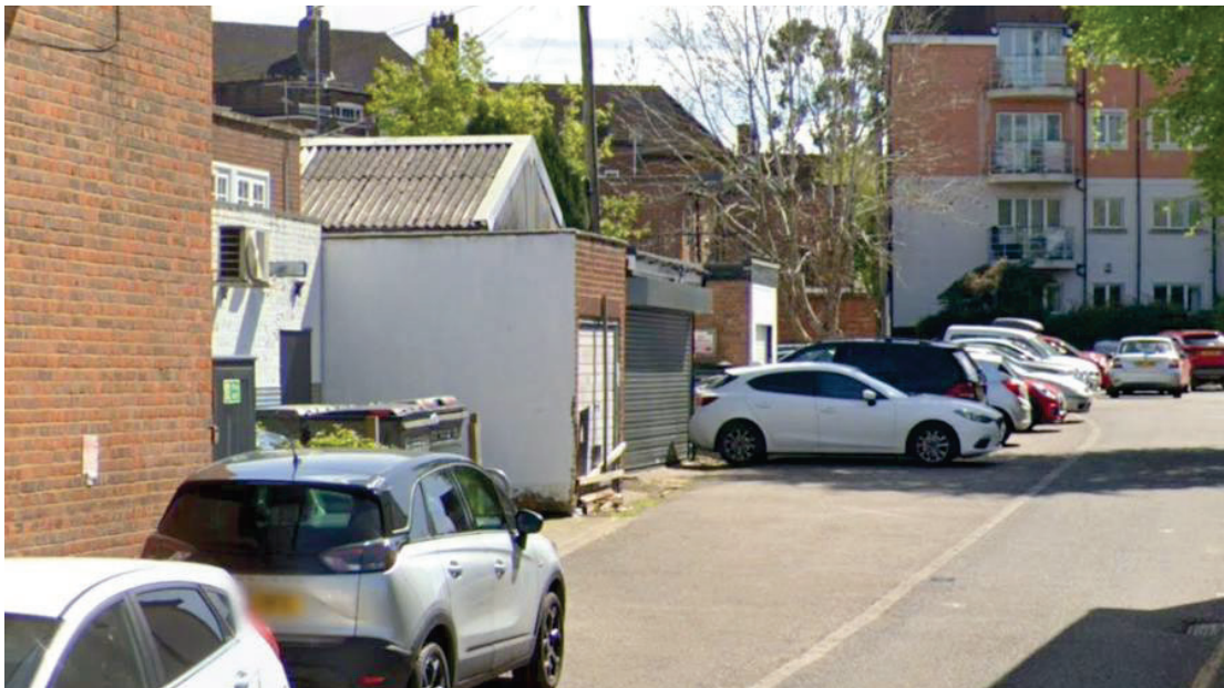
Figure 14: Rears of High Street Properties as Viewed from the Access Road
