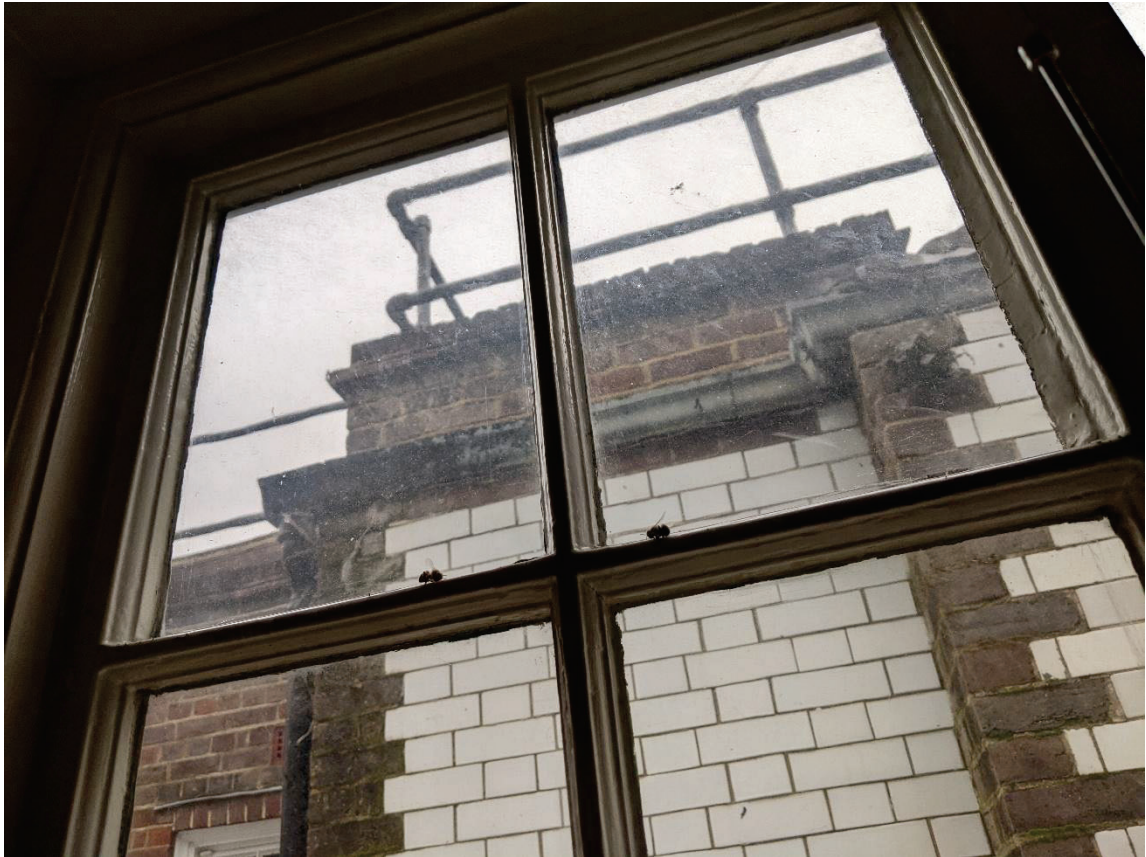
Figure 18: View Upwards from Inside no. 56a (Following amendments, the second floor balcony to Flat 5 would no longer be directly above this window)
