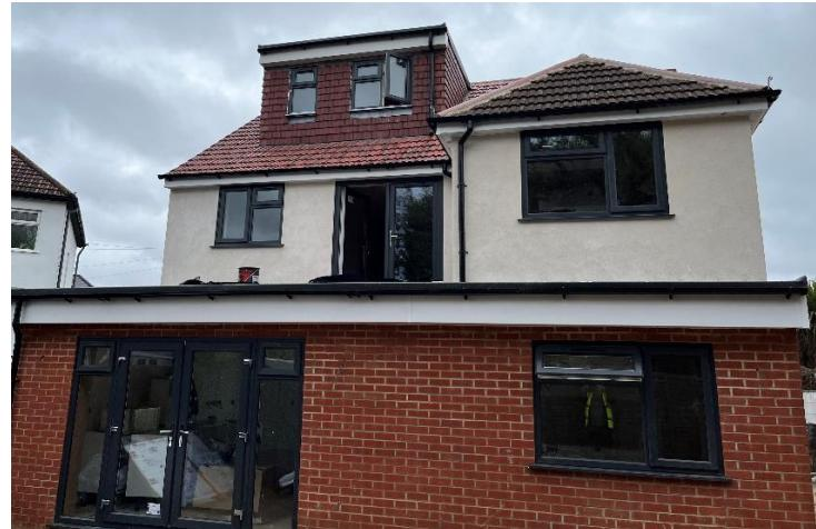
The reason of the small change is that the structural engineer placed the steel beam support for the floor, roof and dormer in a measured location and the contractor built off the beam resulting in the rear dormer wall being approx. 250mm closer to the rear of the building. This has enlarged the rear dormer wall downwards by approx. 200mm. and has not raised the dormer roof any higher than the Approved drawing, see detail photo below.
