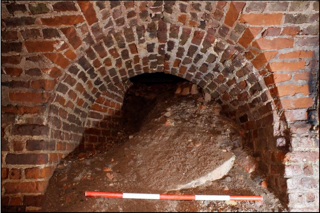
Plate 31: Room 12 looking East
