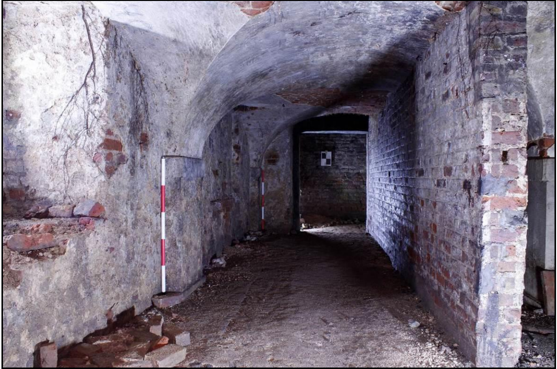
Plate 23: Room 2 looking north
