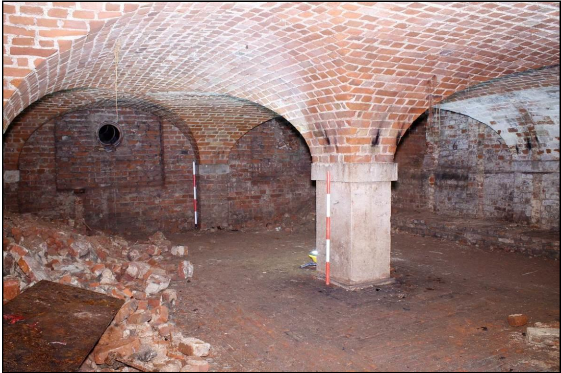
Plate 12: Room 6 Looking Southwest
