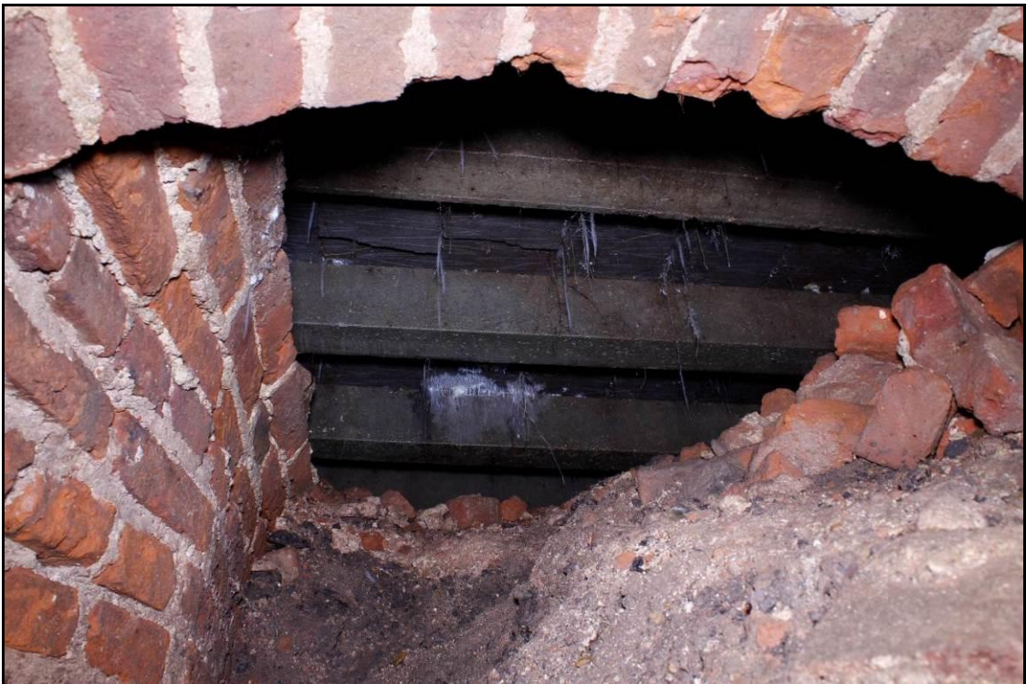
Plate 32: Room 12 Concrete beams
