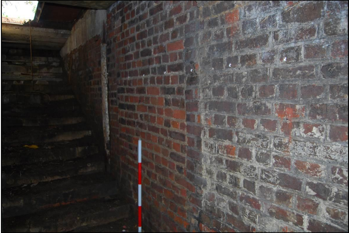
Plate 22: Entrance Area Room 1 Looking Southeast
