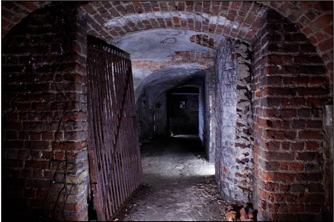
Plate 21: Iron door between Room 2 and 4
