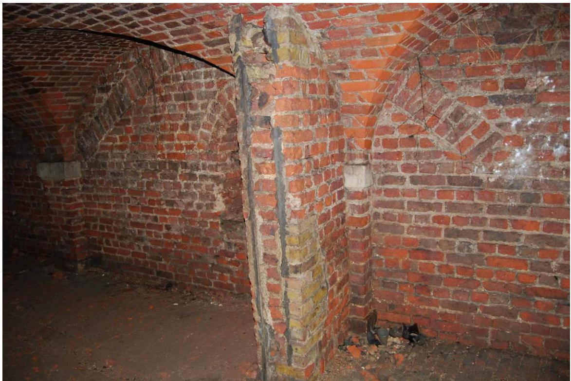
Plate 8: Relieving arch across Icehouse, Rooms 4 and 5, Looking Southwest
