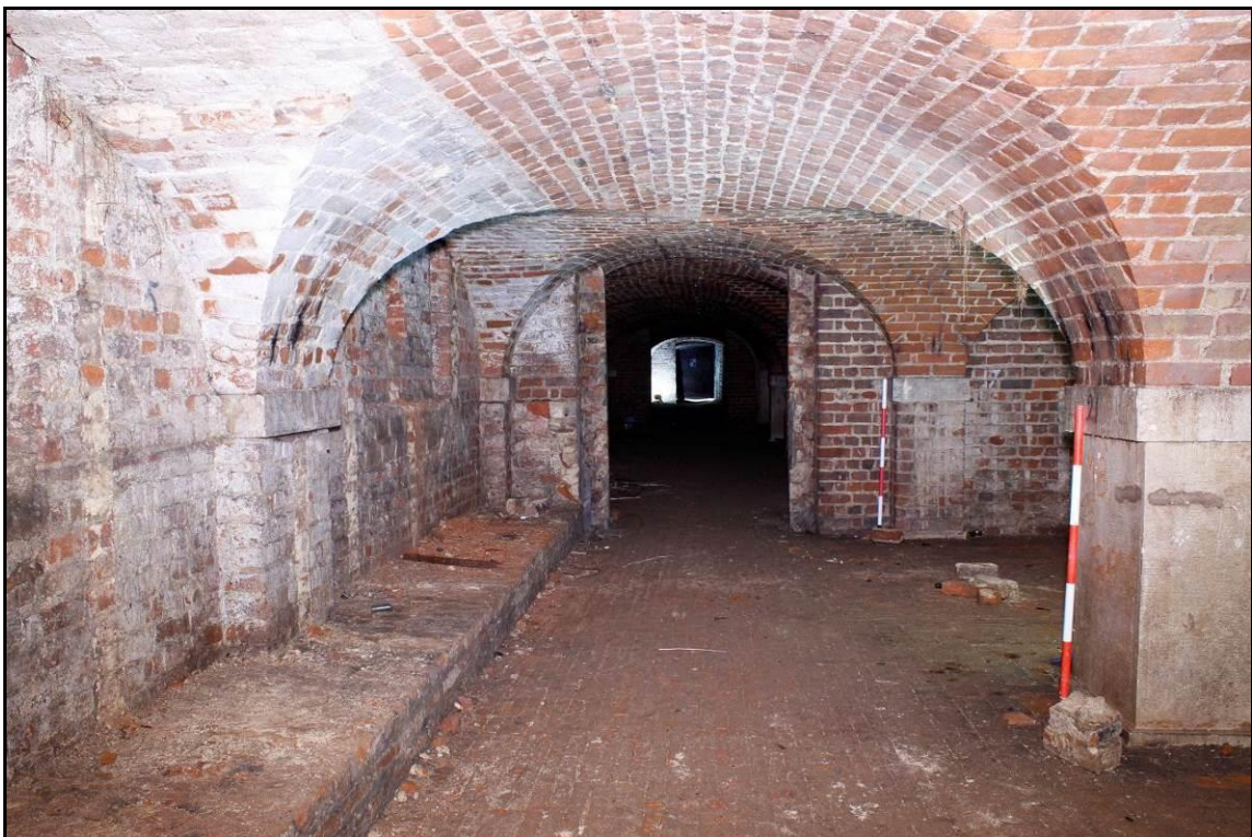
Plate 13: Room 6 looking towards door to Room 5
