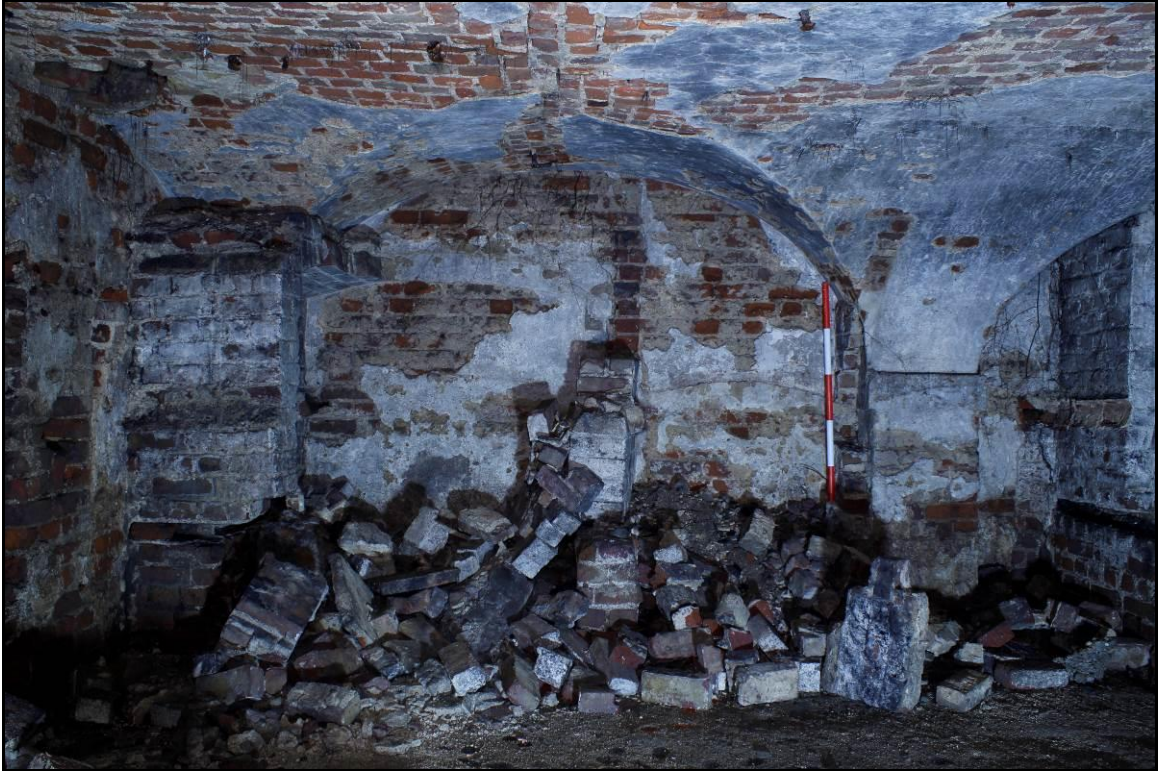
Plate 19: Room 3 demolished brickwork
