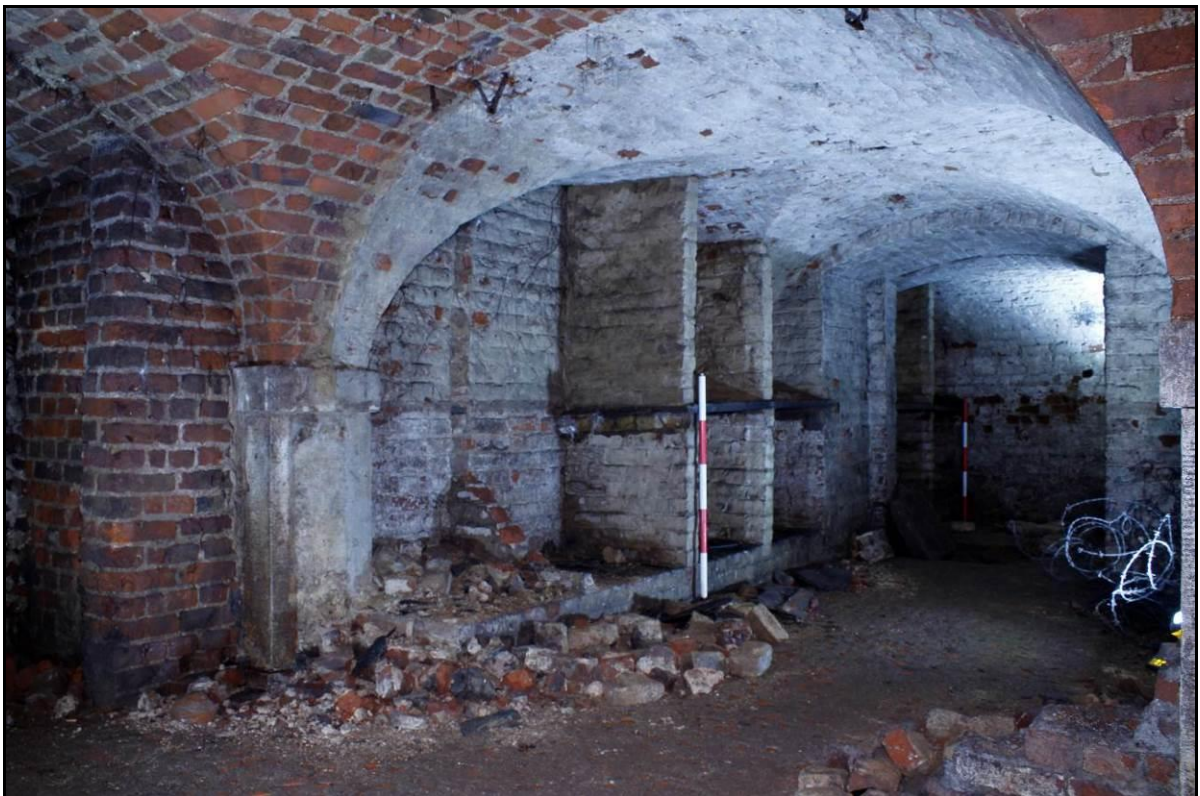
Plate 27: Room 7 to 8 Overview Looking Northwest
