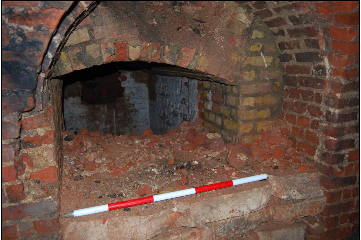
Plate 30: Room 11 Looking Southeast
