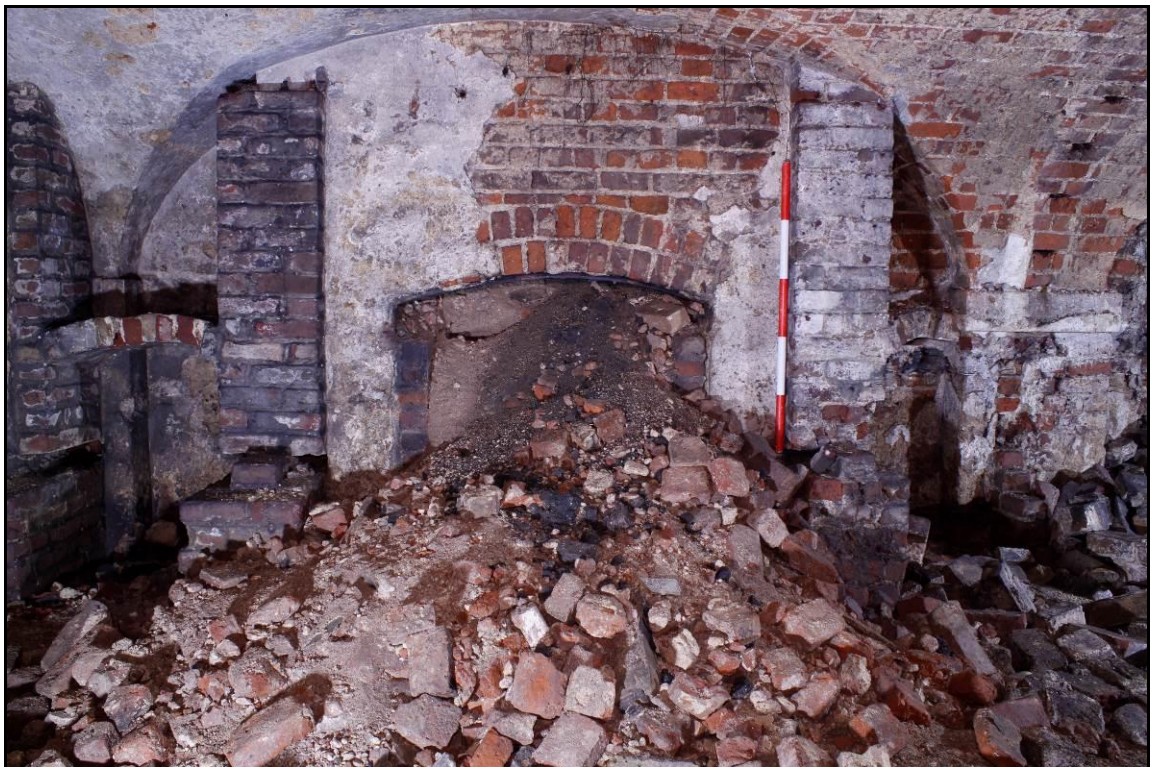
Plate 18: Fireplace in Room 3, looking East
