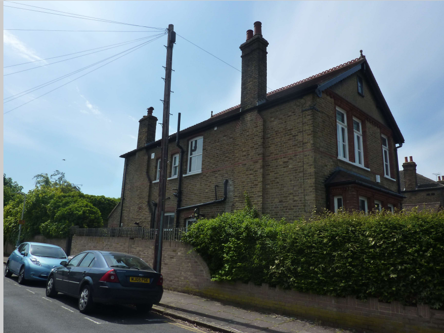
3.2 – Photograph of 13 Queens Road taken from the junction of Queens Road & Kings Road.
