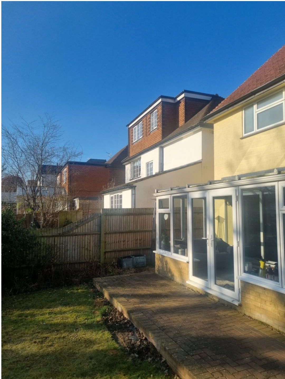
Rear / Side Elevation of Properties 30 & 36 Park Avenue (Showing two storey rear extension of No30 & 32)
