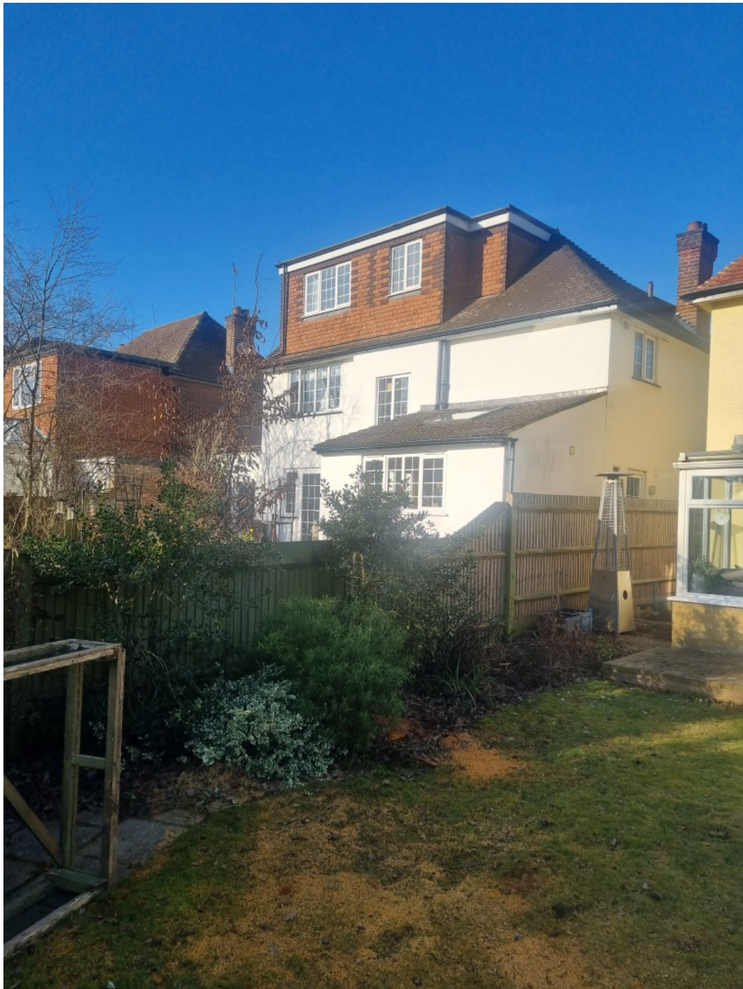
Rear Elevation of Properties 32 & 34 Park Avenue (Showing two storey rear extension of No32)
