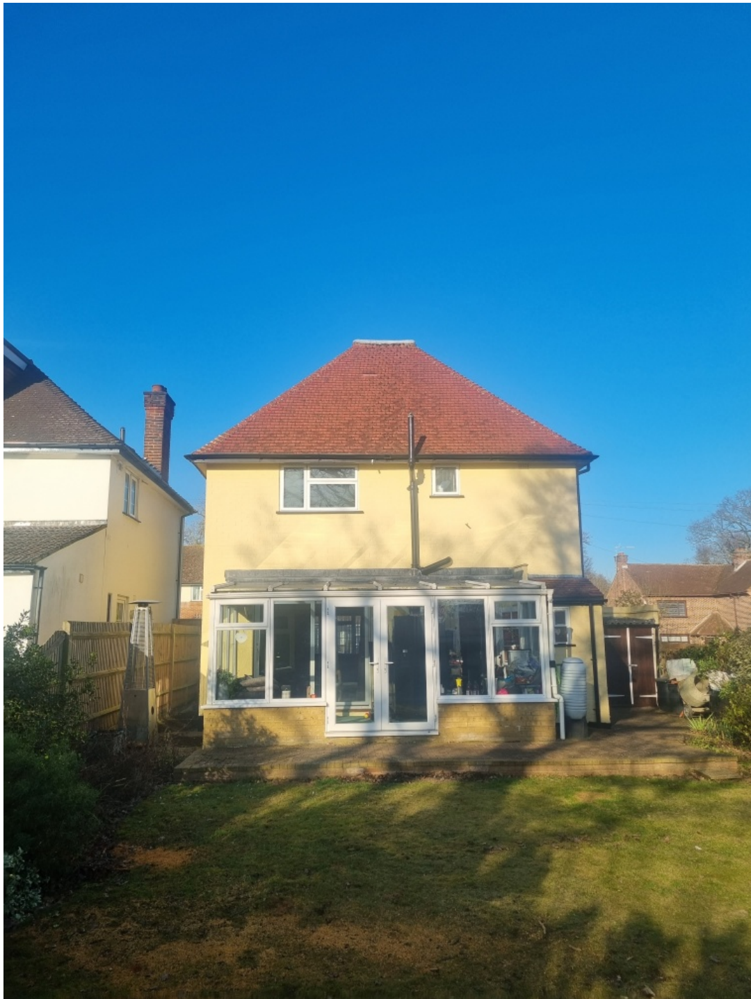
Rear Elevation of Property
