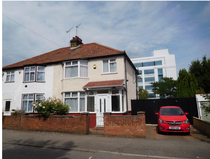
FRONT VIEW OF APPLICATION SITE
