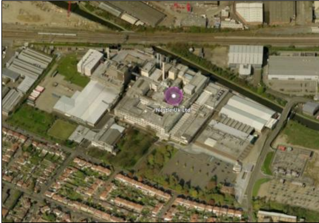
Figure 2.12: Aerial view of the former Nestlé Factory (2016, BING)
