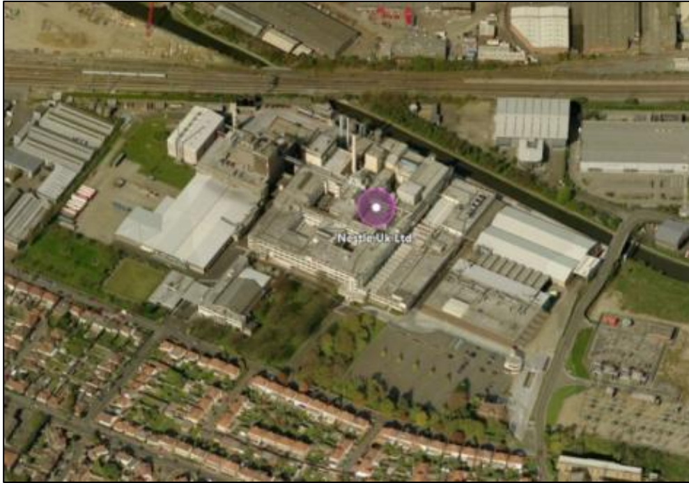
Figure 2.13: Aerial view of the former Nestlé Factory (2016, BING)
