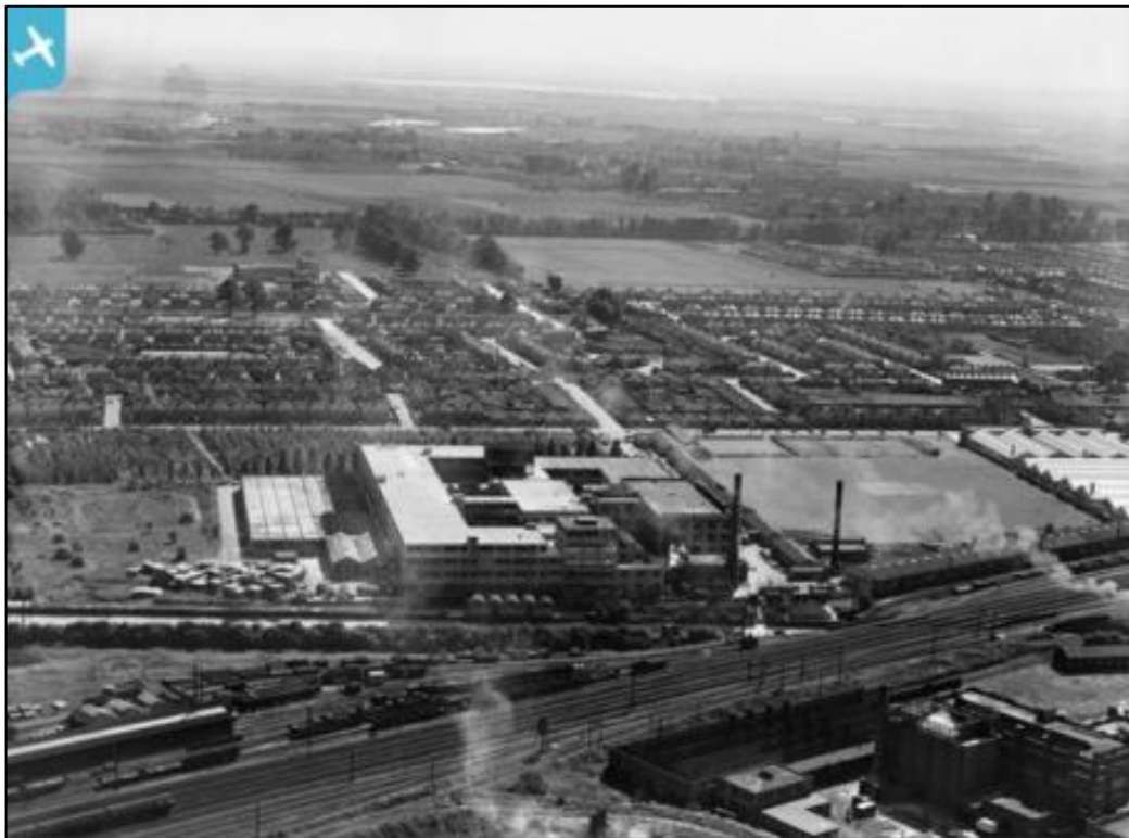
Figure 2.10: Aerial photograph of the Nestlé Factory at Hayes, taken 1939 (Britain from Above)
