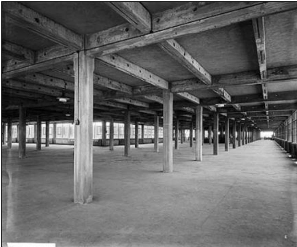
Figure 2.5: Image from 1921 showing the construction of the extension at Hayes Cocoa Factory with exposed concrete beams and posts (Historic England Archives)
