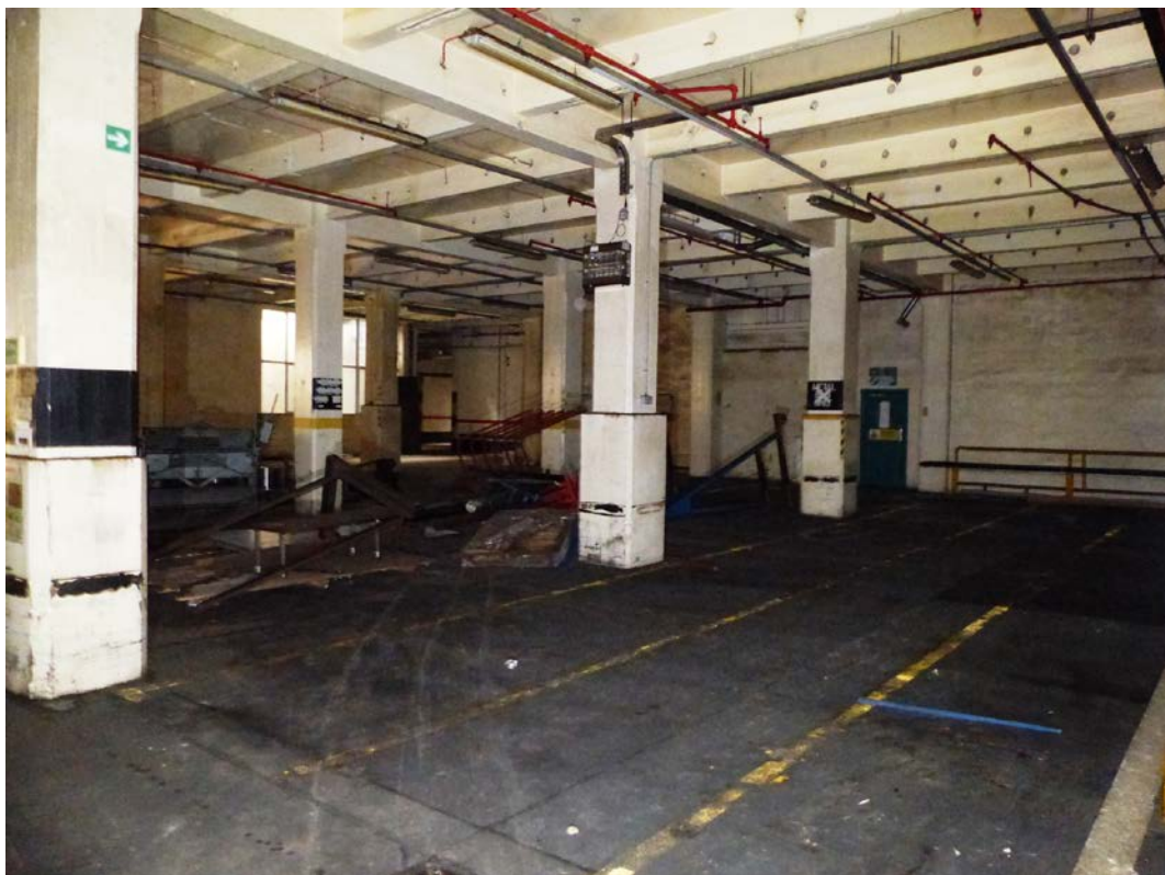
Fig 40 Tote Bin Store, GF22, looking north-west
