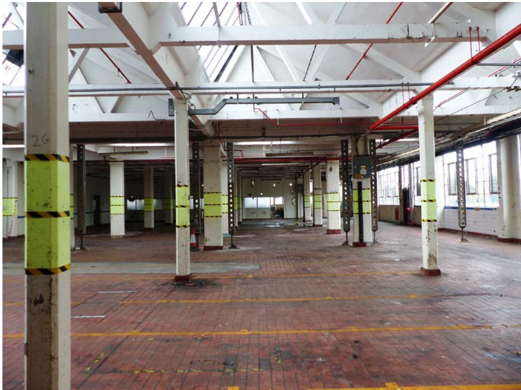
Fig 29 Ground floor storage area within the single storey east section, looking east
