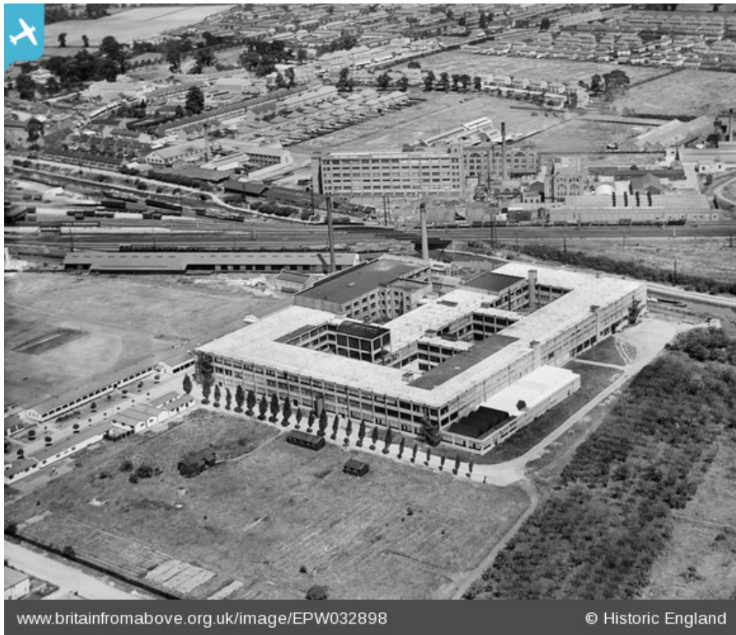
Fig 11 The Main factory building in the 1930s from the southeast (Britain from Above)
