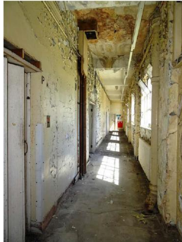
Fig 82 Northern end of the corridor on the first floor, looking north
