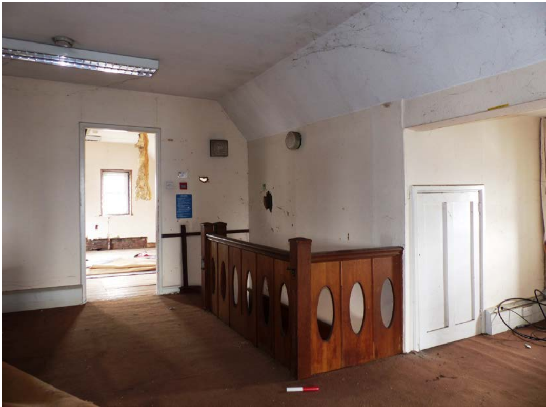
Fig 112 Second floor landing of the staircase, protected with timber panelled railing
