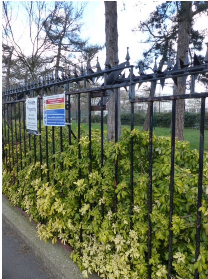
Fig 132 Railing Type D, looking north-west
