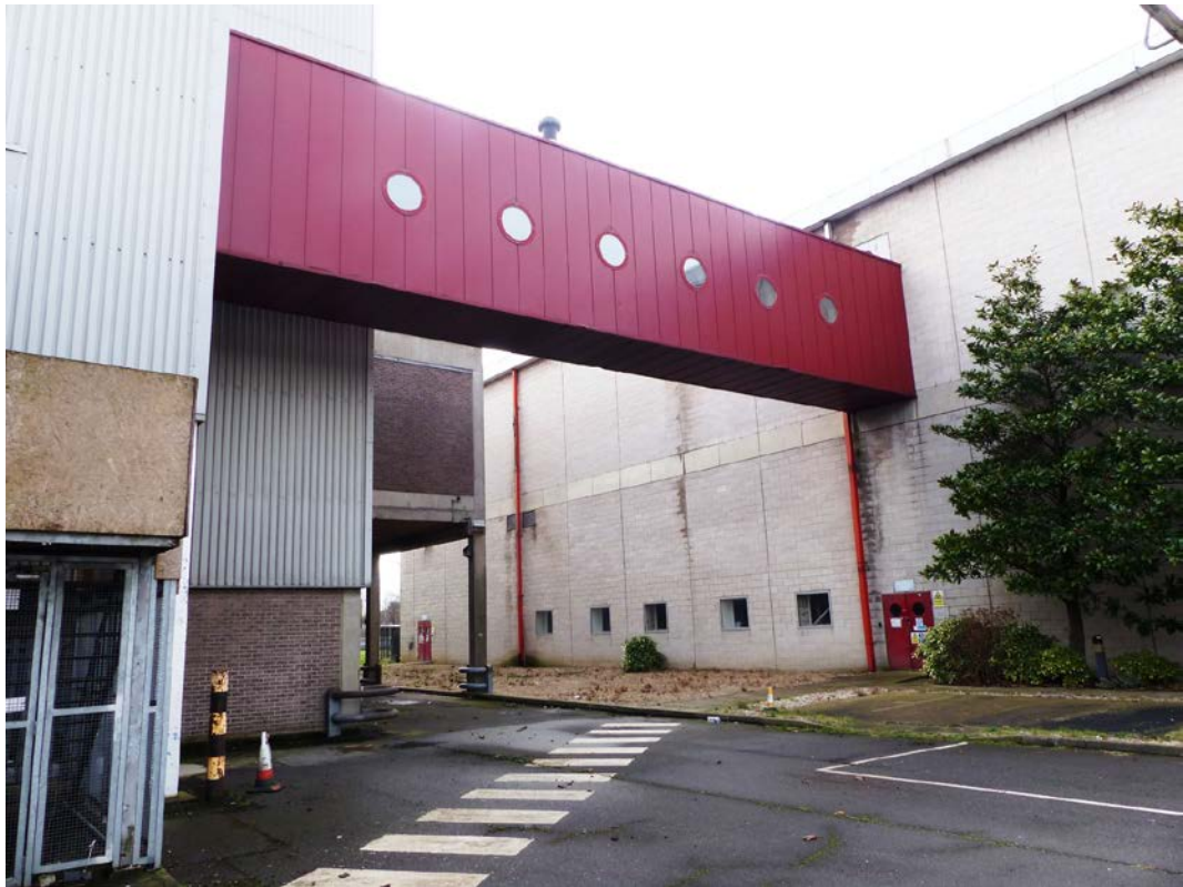
Fig 149 A modern high-level steel framed walkway connecting the two late 20th-century factory buildings at the north-west corner of the site.
