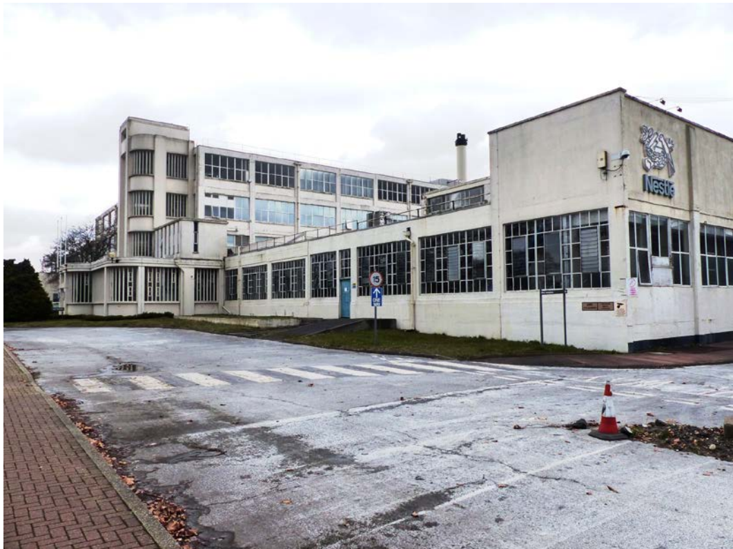
Fig 14 Main factory building, looking north-west
