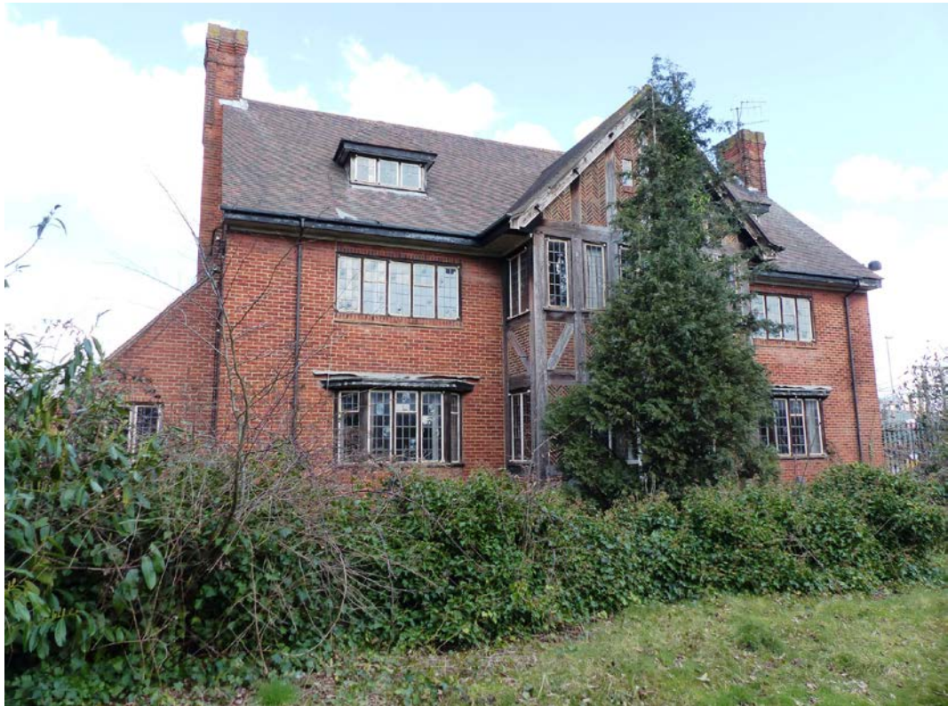
Fig 88 South elevation of the lodge, looking north-east
