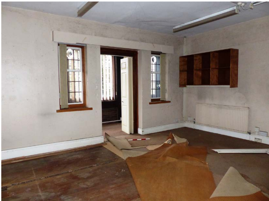
Fig 110 Room 1F4, looking south-west
