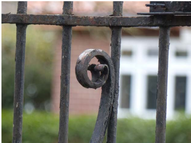
Fig 128 Scrolled outrigger detail, looking south
