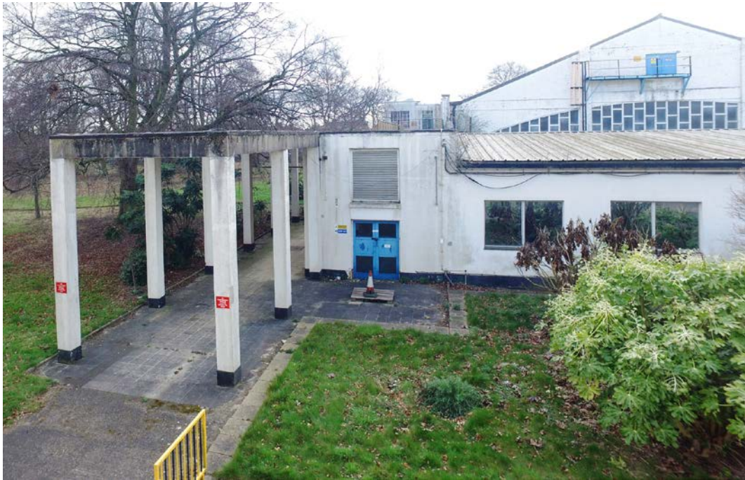
Fig 69 East end of the north elevation, looking south
