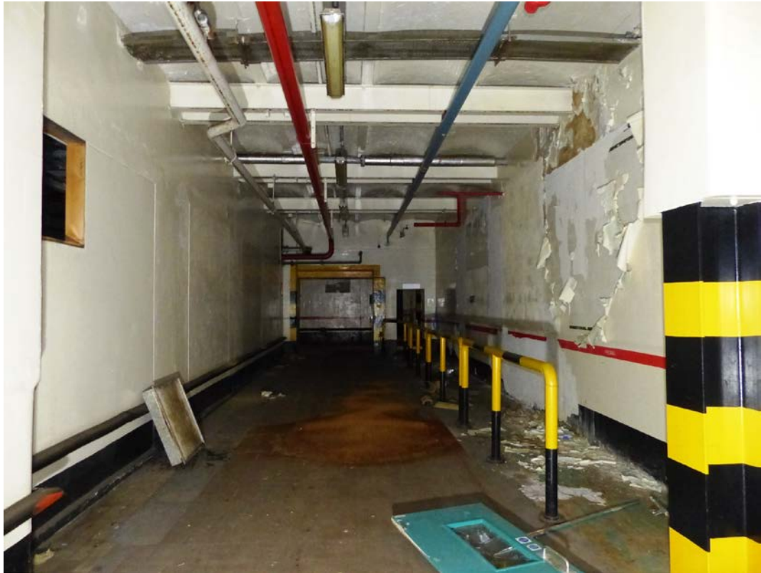
Fig 41 GF28, looking east
