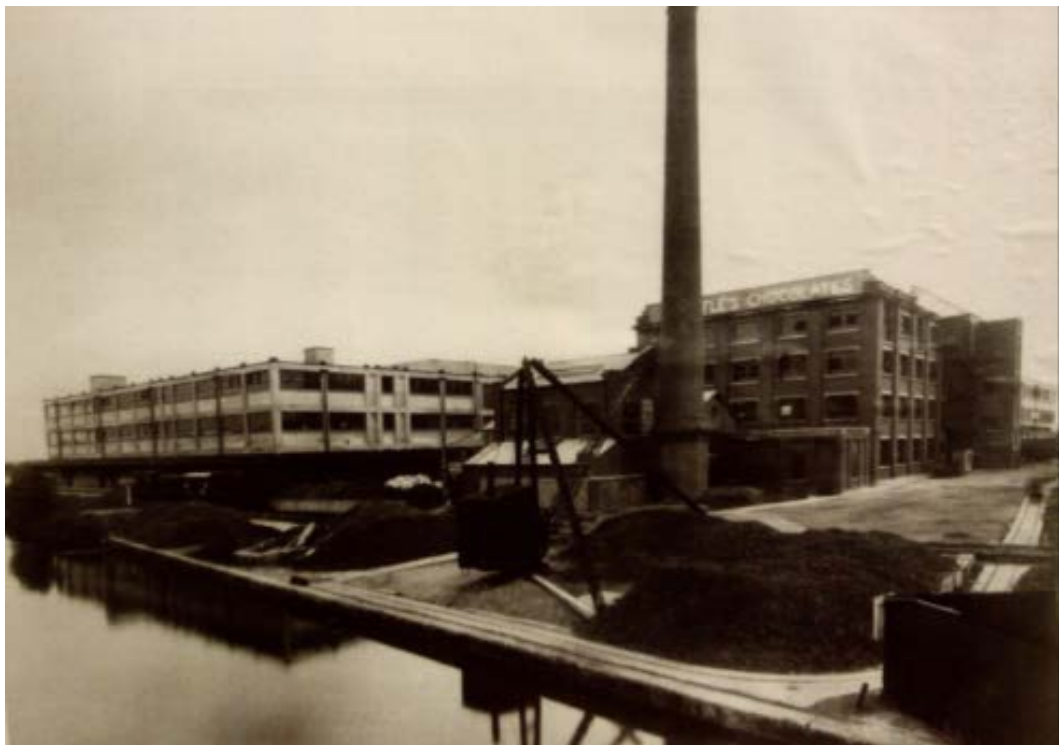
Fig 10 1930s view of the factory from the north-west with the extension (Turley Heritage 2017)
