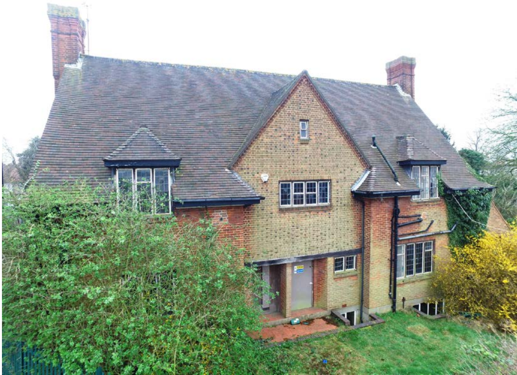
Fig 91 North elevation of the Lodge, looking south-west
