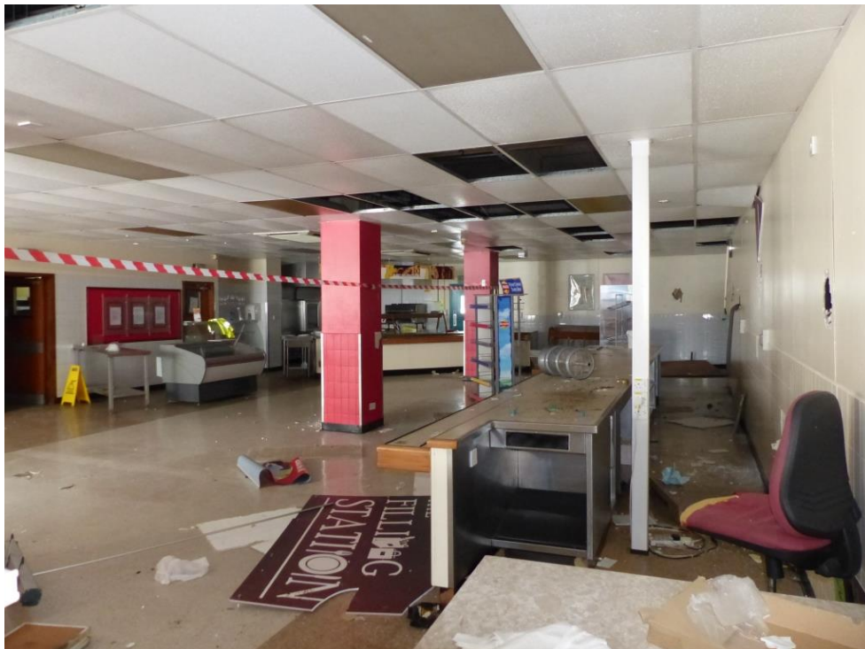
Fig 48 Staff shop and cafeteria, room 1F8 looking north-east.
