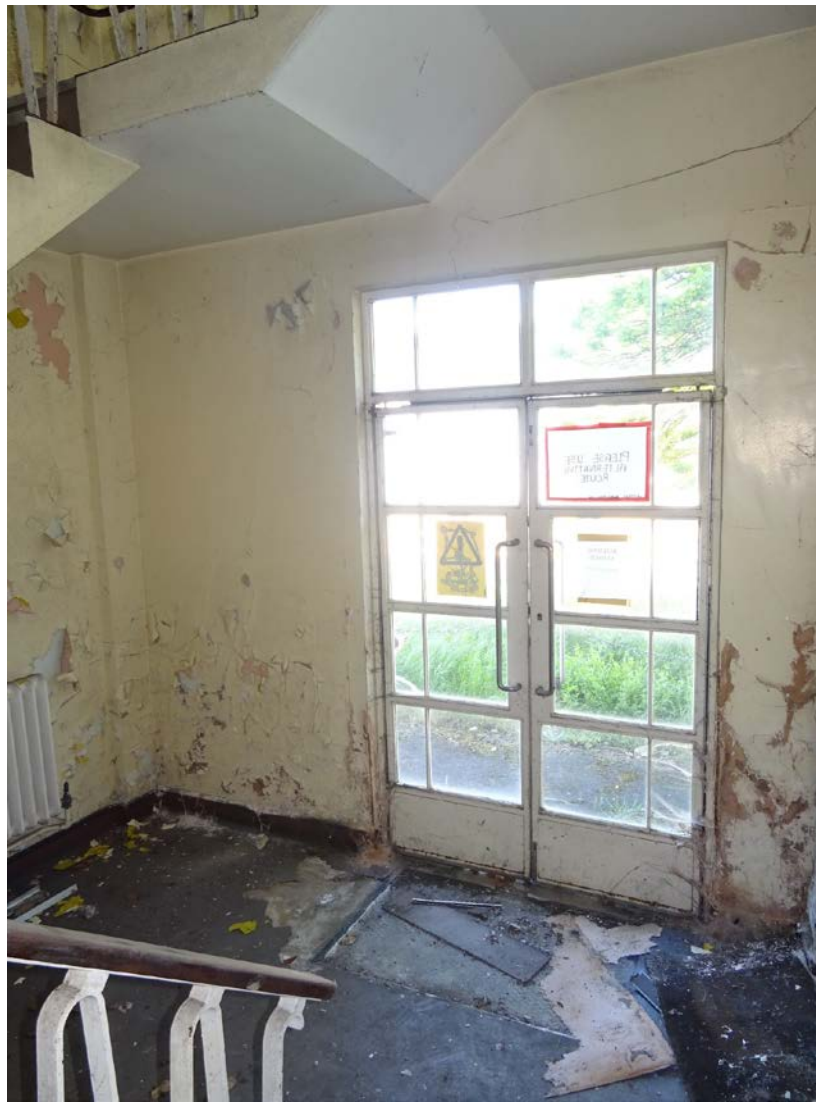
Fig 85 External door from the north-west stairwell
