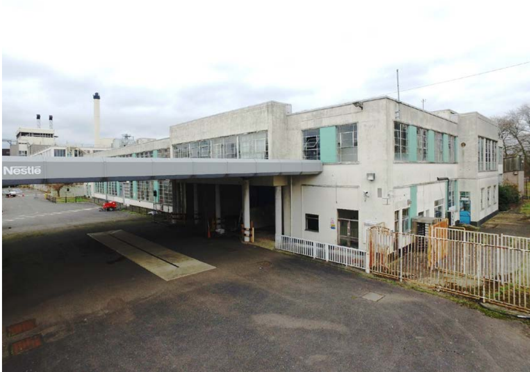
Fig 67 South end of the west elevation with a large steel canopy
