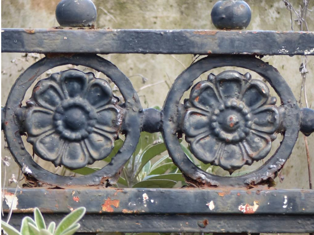
Fig 122 Main Gate rosette detail from the south
