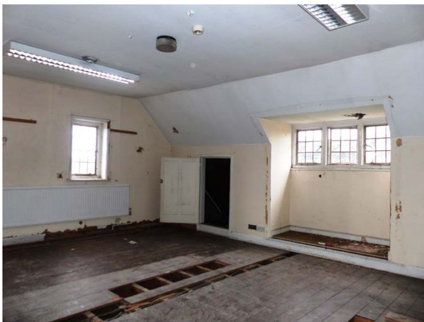
Fig 116 Dormer window recess to the south in room 2F3, looking south-east
