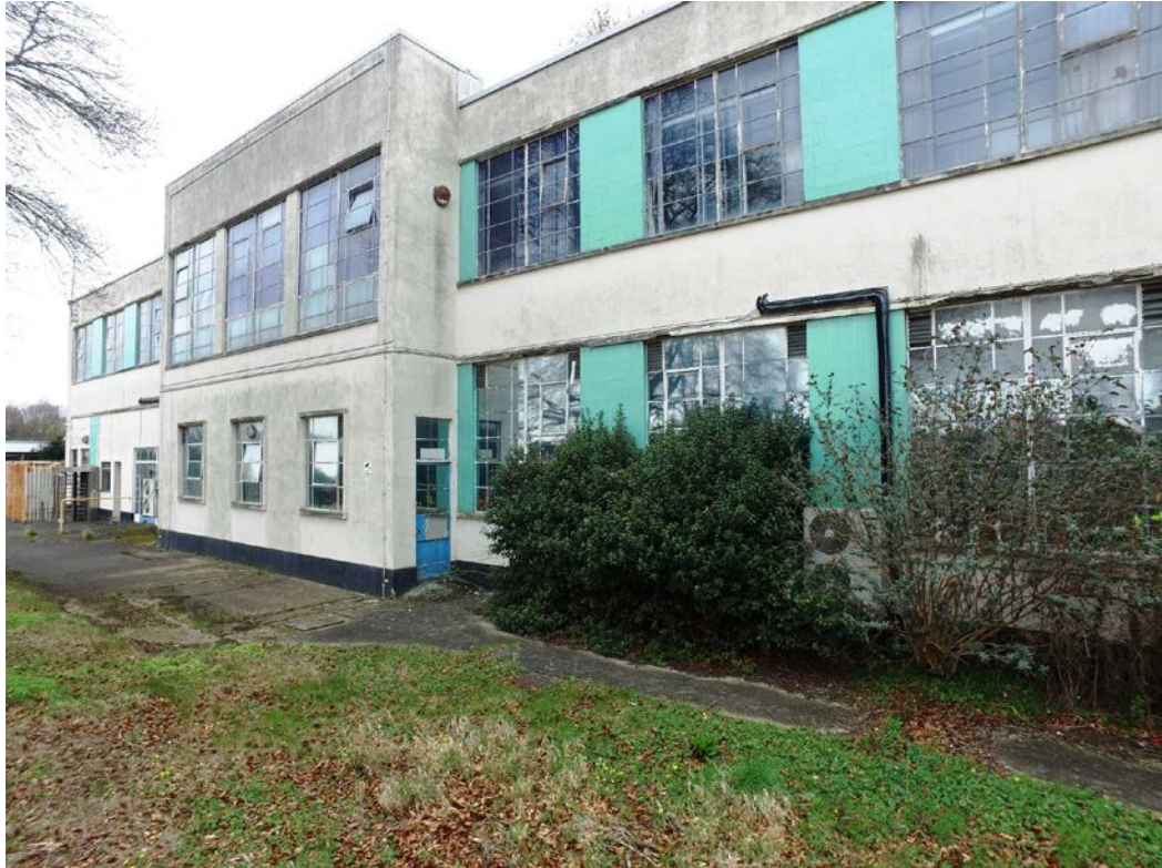
Fig 65 South facing elevation of the former canteen, looking north-west
