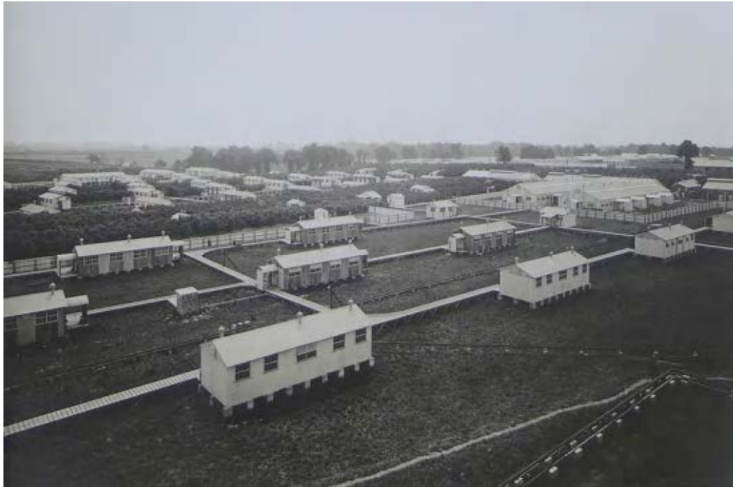
Fig 8 NFF No.7 sheds, cleanways and railway tracks (Collier 2014)
