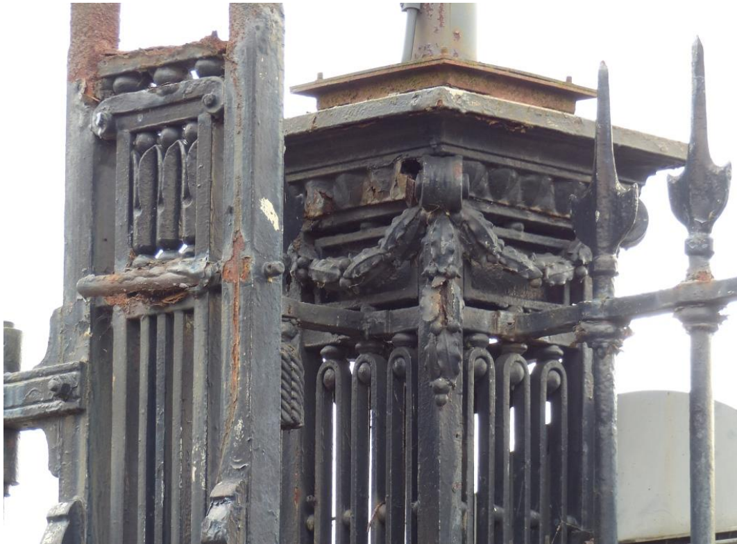
Fig 119 Beverage Gate pier detail seen from the northwest
