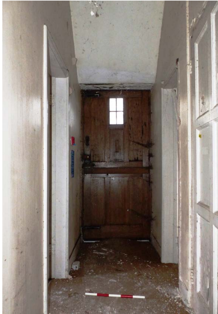
Fig 95 External door to the west from the ground floor hallway, looking west
