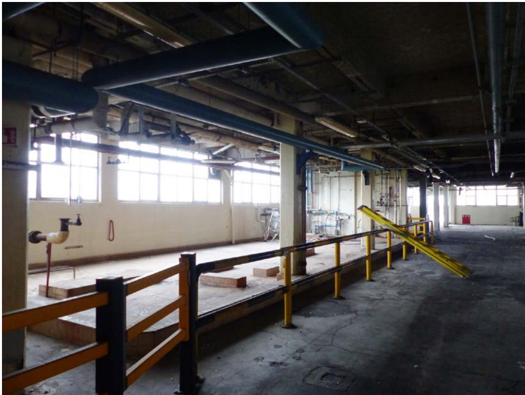
Fig 55 Processing areas along the fork-lift route on the second floor at the north end of the building
