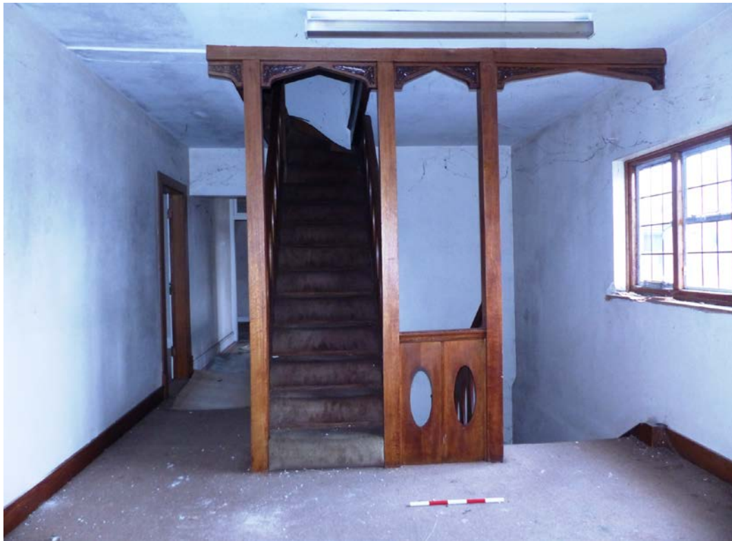
Fig 107 First floor landing, looking west
