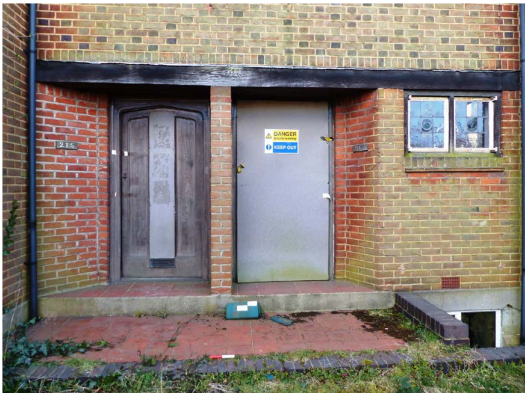
Fig 92 Entrance doorways from north
