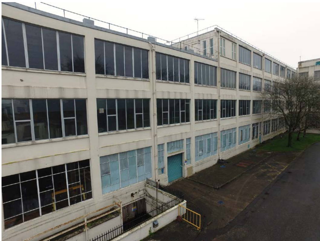
Fig 16 Central section of the south elevation of the main factory building
