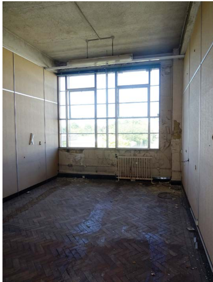
Fig 81 One of the first-floor office rooms in the west wing with herringbone wood parquet flooring
