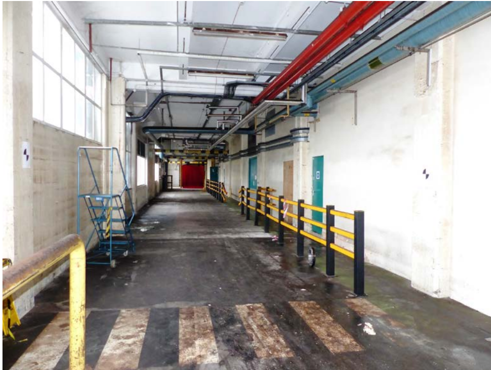
Fig 46 Fork-lift route along the north end of the ground floor, looking east
