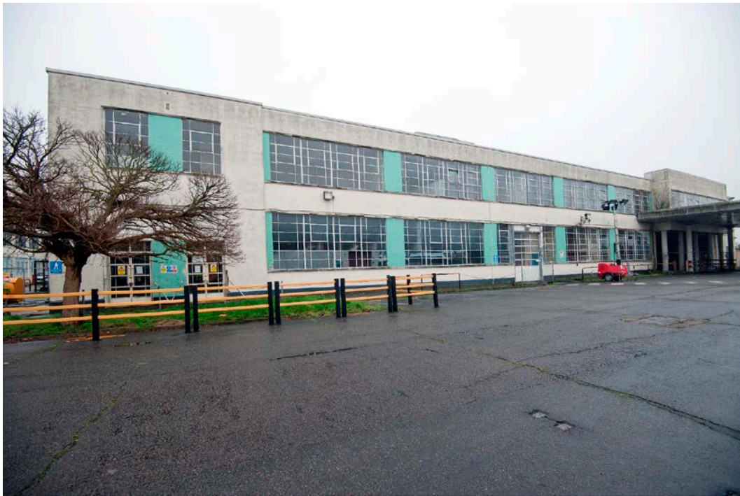
Fig 66 West elevation of the Former Canteen, looking south-east
