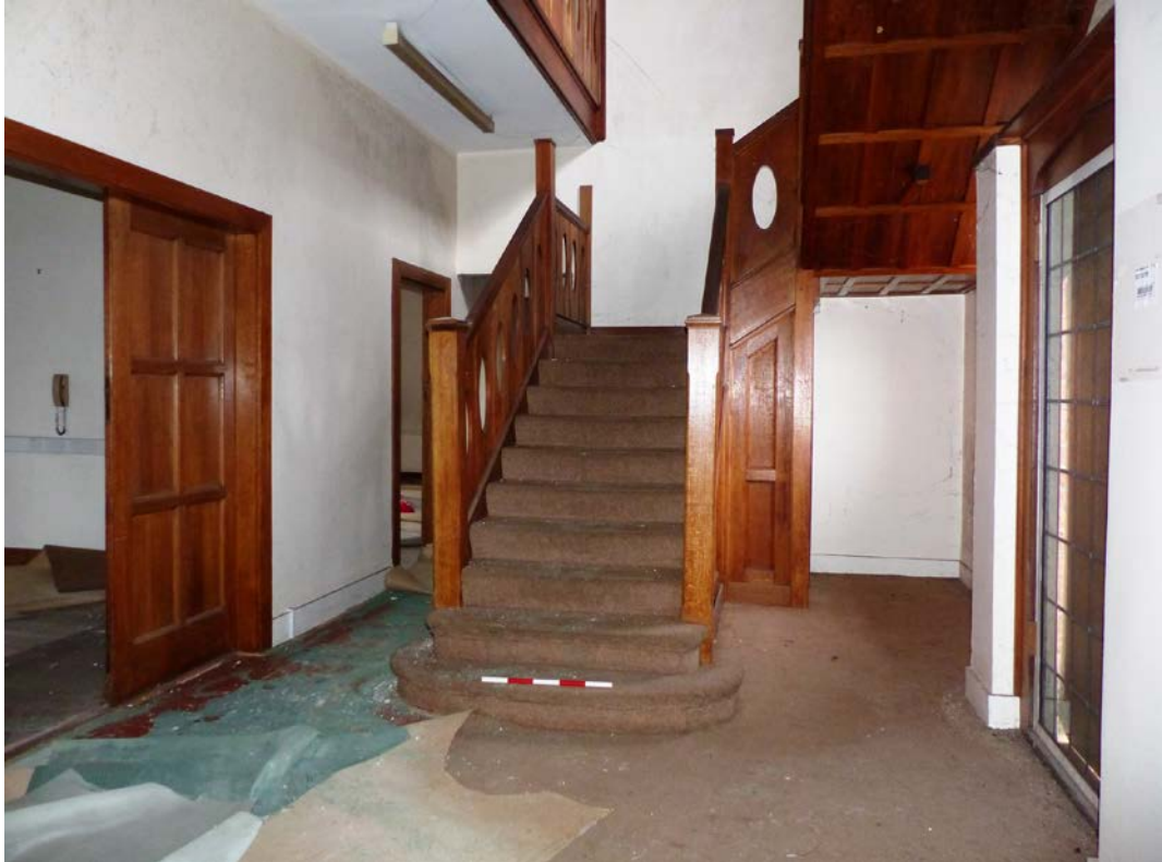
Fig 93 The entrance hall and staircase on the ground floor, looking south-west
