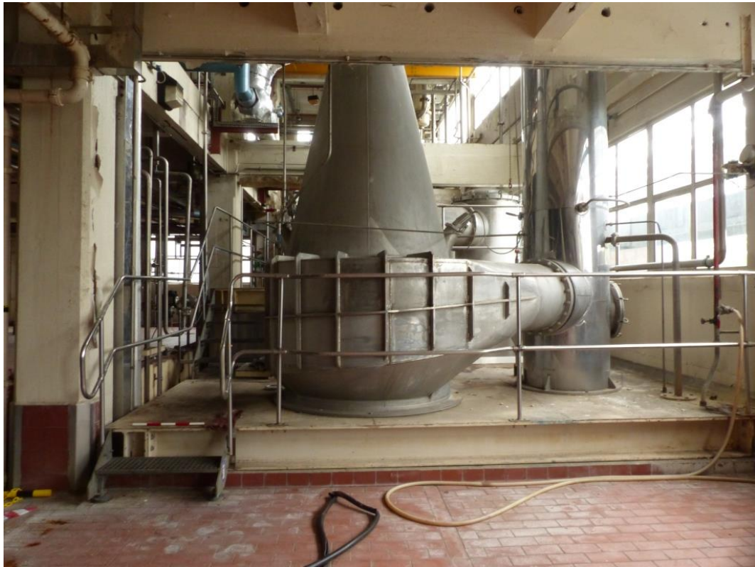
Fig 51 Room 1F49 looking west
