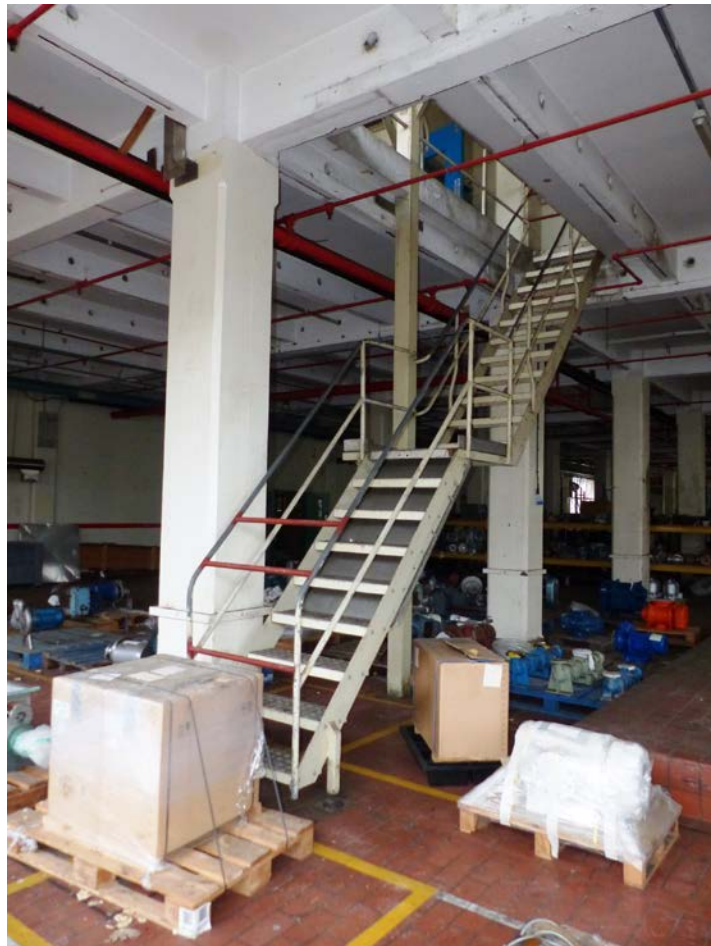
Fig 32 A staircase from GF1 provided access up to the first floor, looking north-
