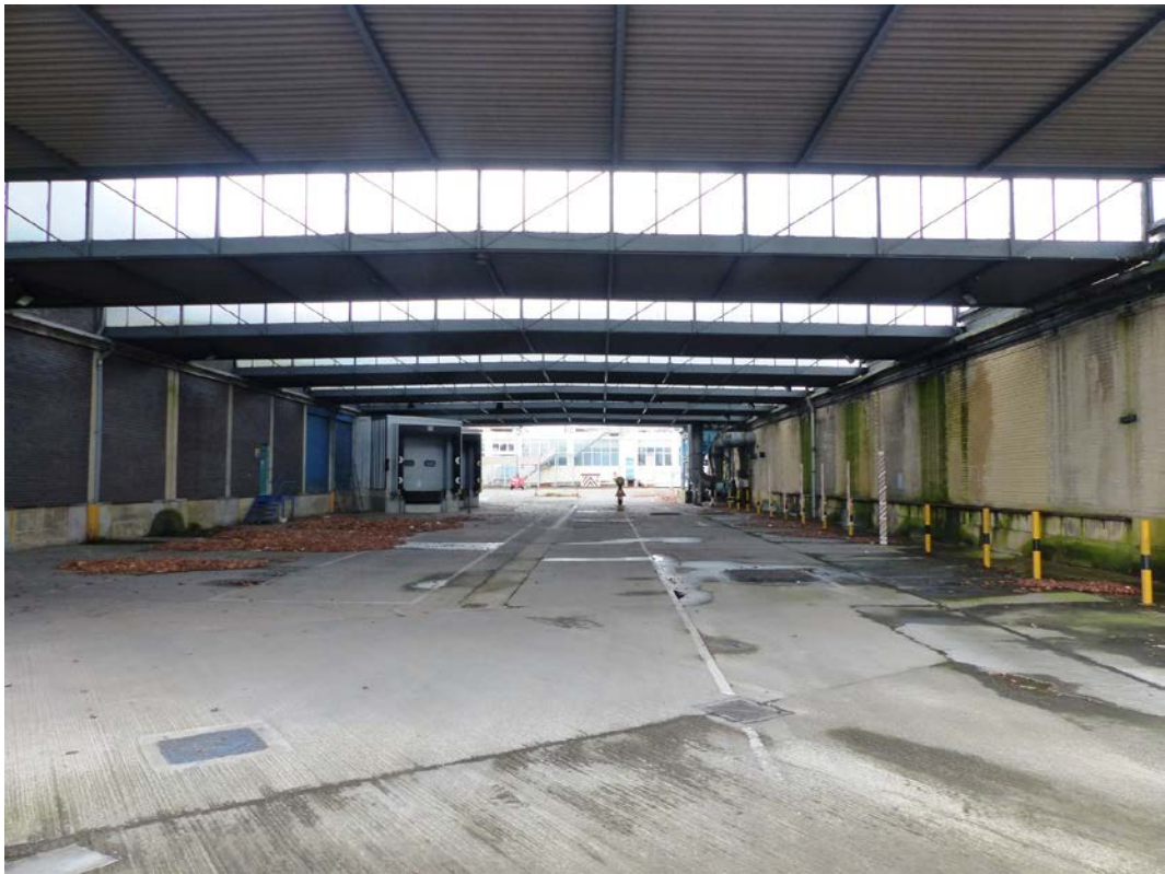
Fig 145 Loading bay with modern steel canopy between the two large factory buildings in the north-east corner of the site.
