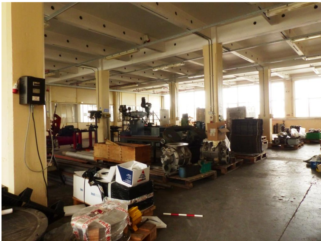
Fig 52 Room 1F61, machine storage looking north-east
