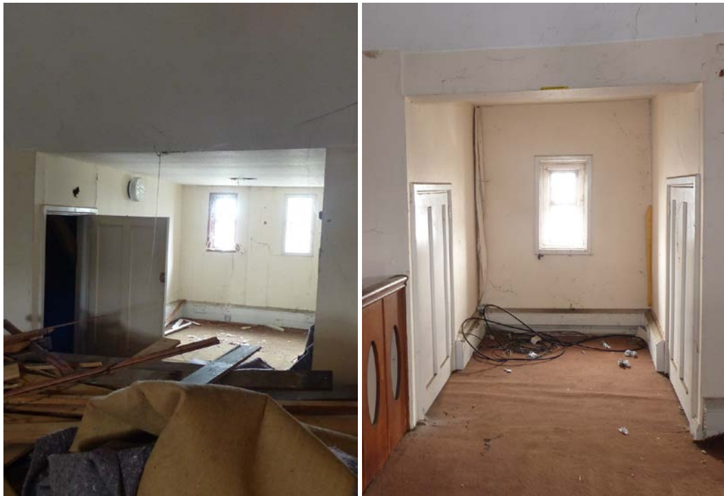
Fig 113 South (left) and northern (right) alcoves in 2F1
