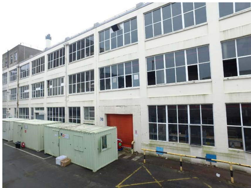
Fig 19 Central section of the west elevation
