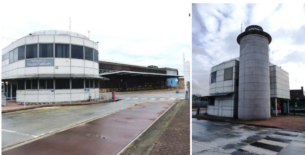
Fig 140 Entrance gatehouse and security office building. Note weighbridge installed in the road (left), view from the north (right)
