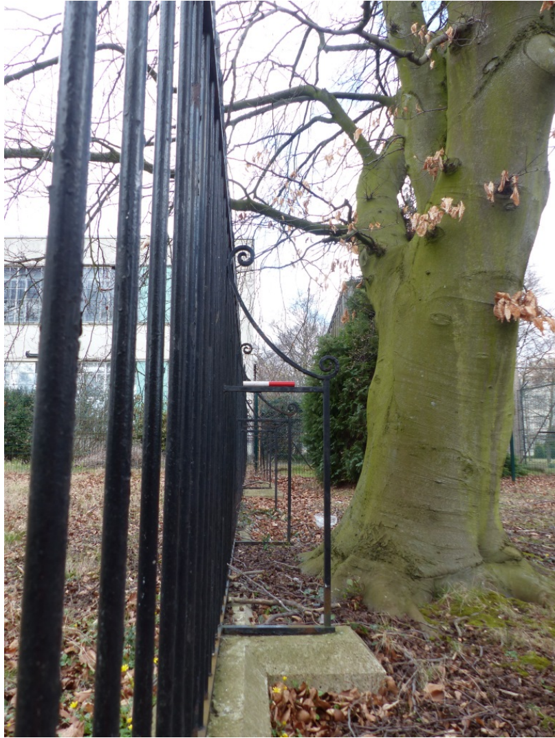
Fig 127 Scrolled outriggers, looking north
