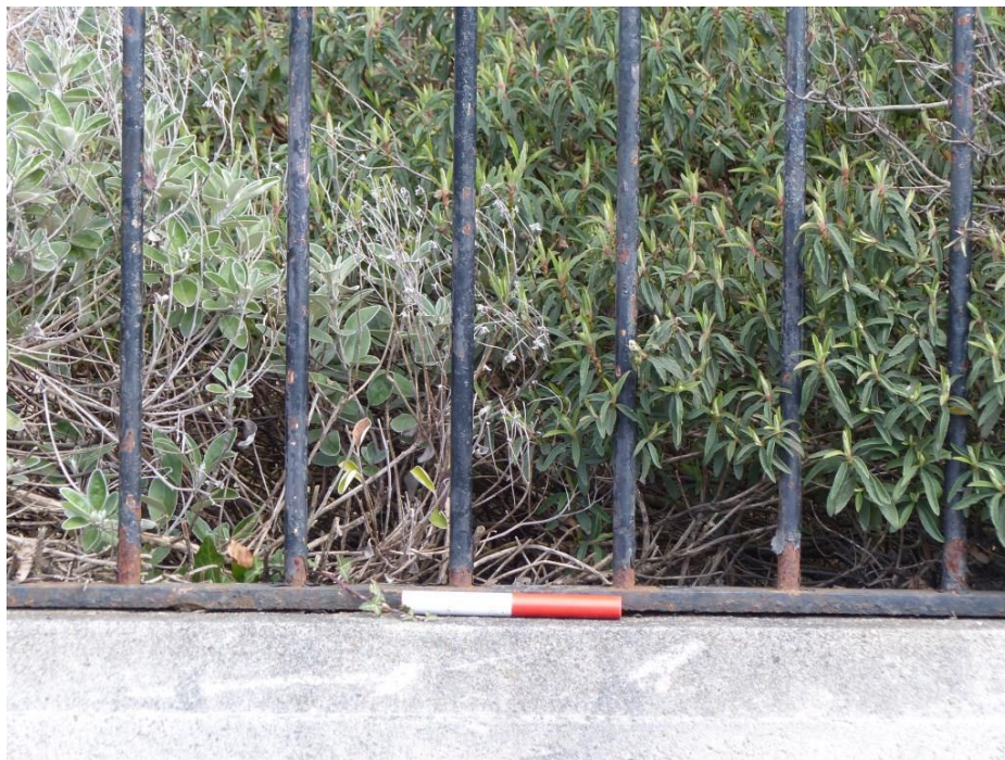
Fig 130 Railing Type B frame rail detail, looking north
