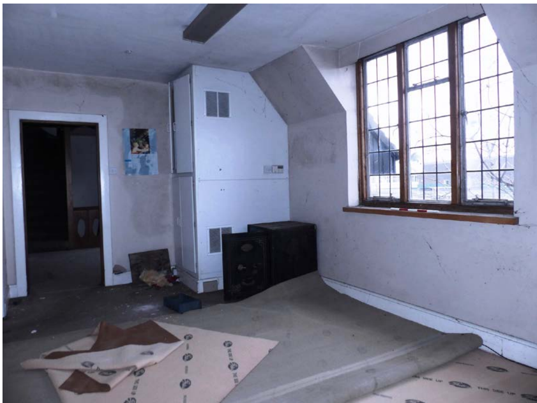
Fig 108 North-east corner bedroom on the first floor (1F2), looking north-west
