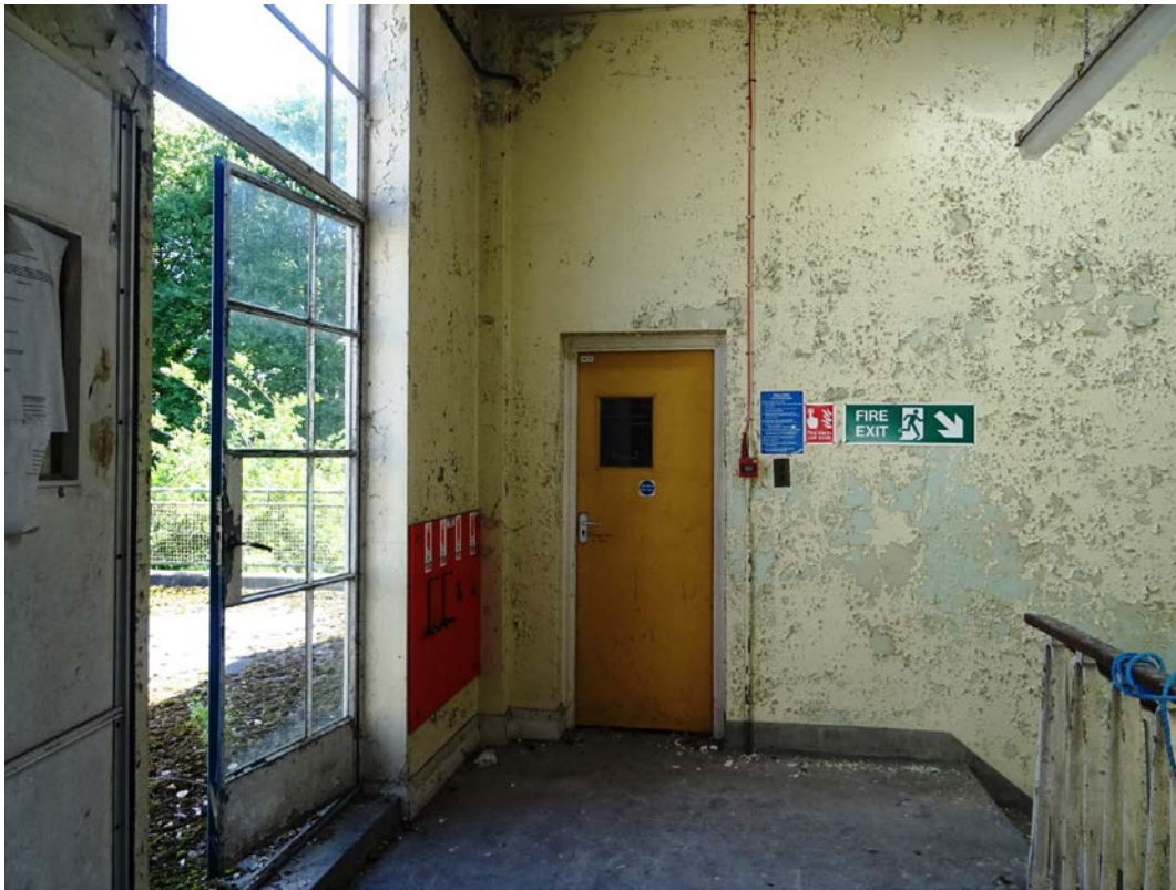
Fig 75 First floor landing at the south-east corner stairwell, looking east
