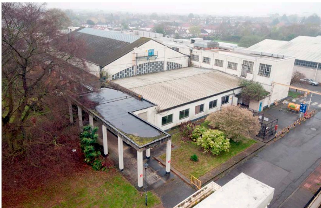
Fig 64 Former canteen building, view from the Main Factory roof, looking south-west
