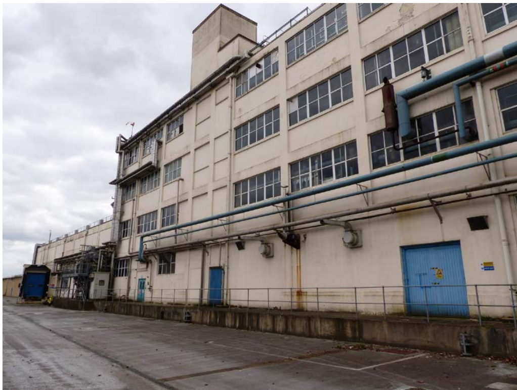
Fig 26 East end of the north elevation of the factory building
