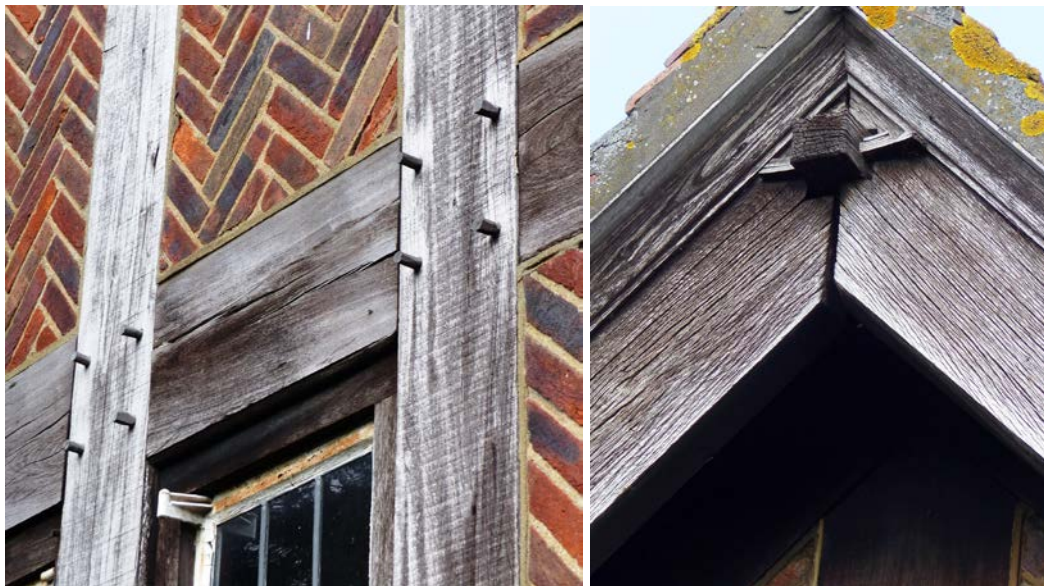
Fig 90 Projecting out wooden pegs and wedge lock
