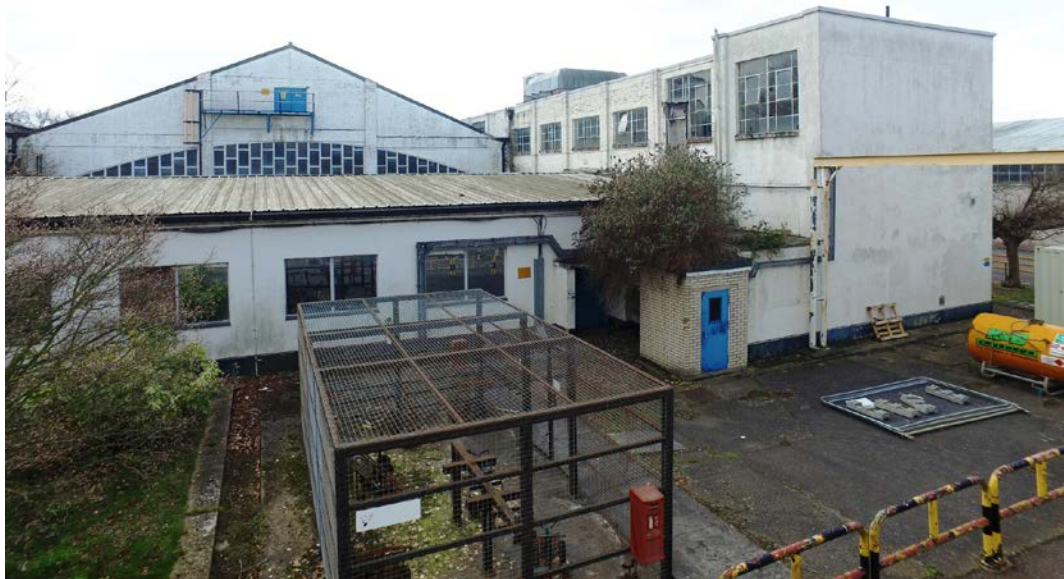
Fig 68 West end of the north elevation, looking south-west
