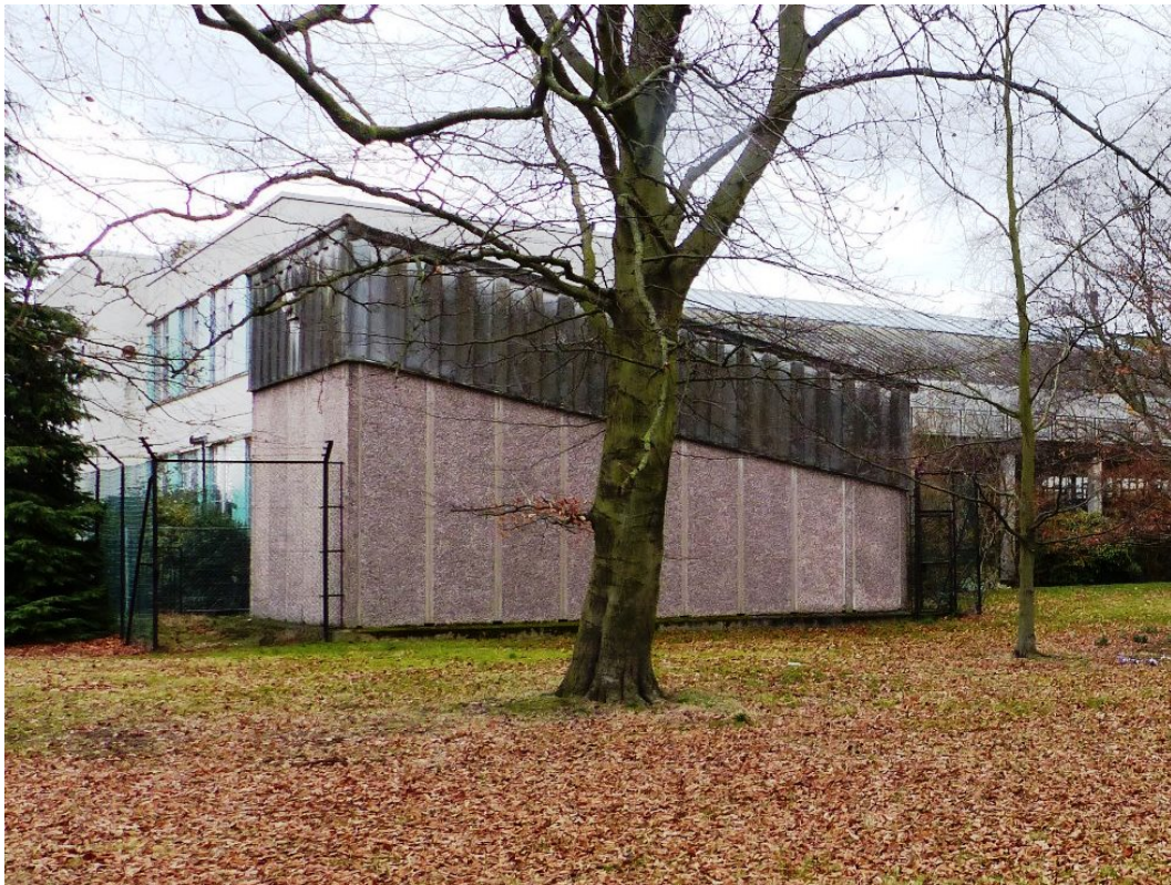
Fig 143 Squash court next to the former canteen building, looking north-west
