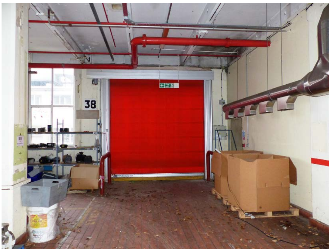
Fig 33 Loading bay at the south-west corner of GF1
