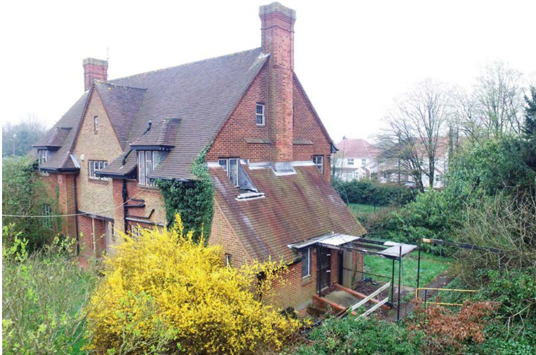
Fig 87 North and west facing elevation of the Lodge, looking south-east
