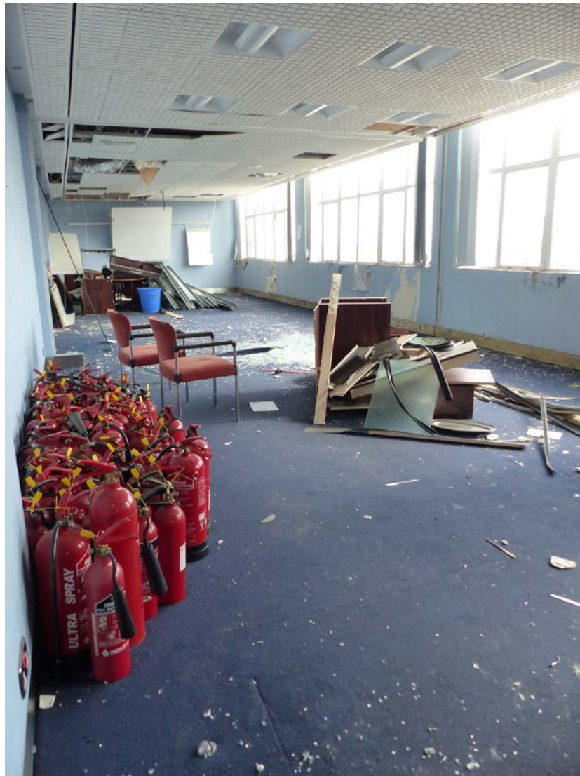
Fig 53 Interior of the board room on the second floor, looking north-east
