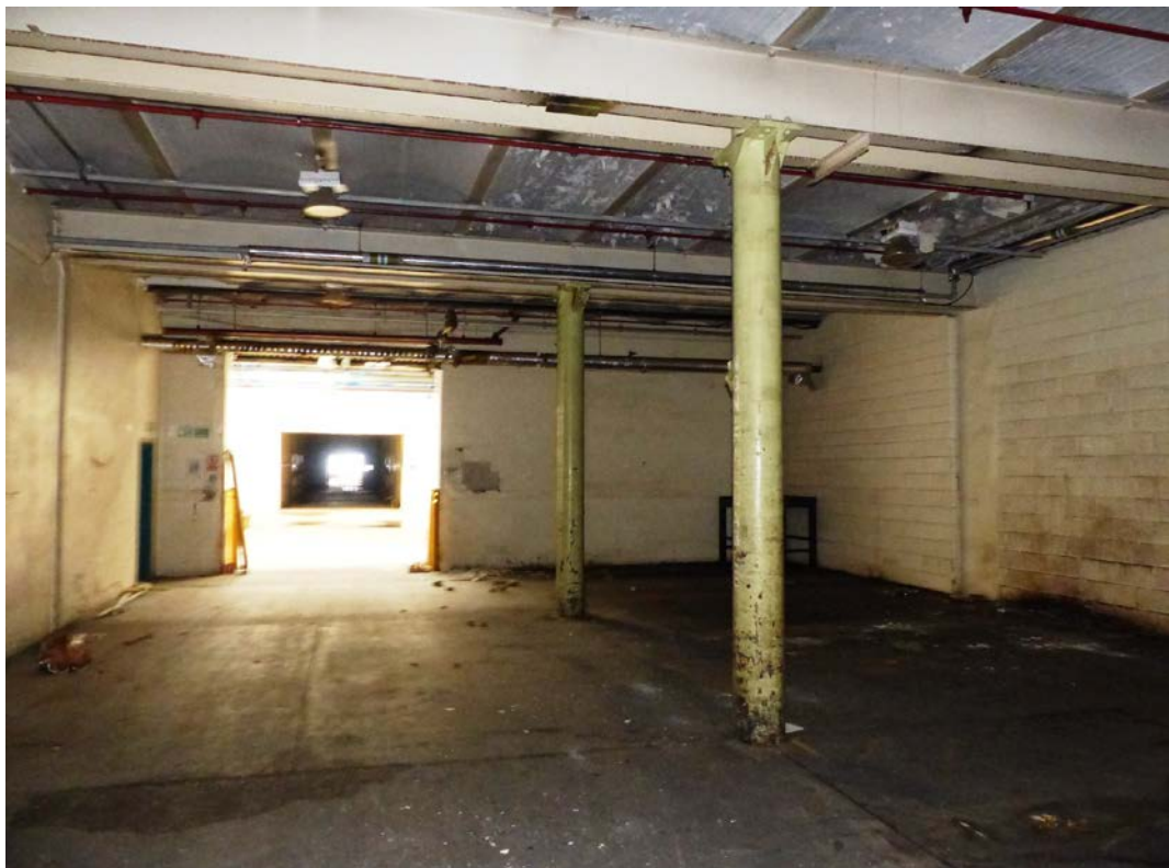
Fig 38 Interior of GF20, looking east
