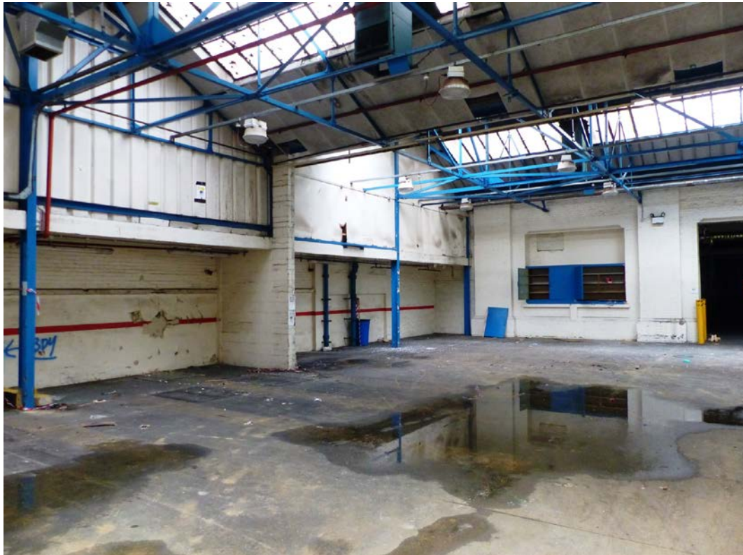
Fig 39 Interior of GF25
