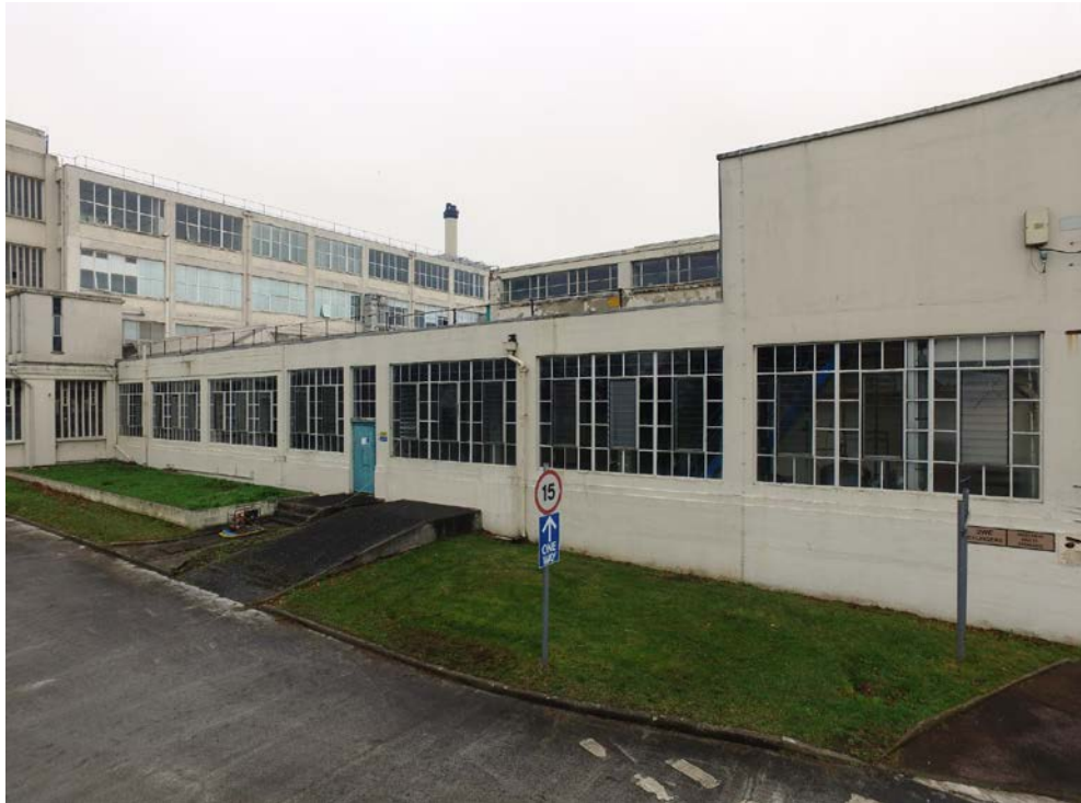
Fig 17 Single storey east section of the south elevation
