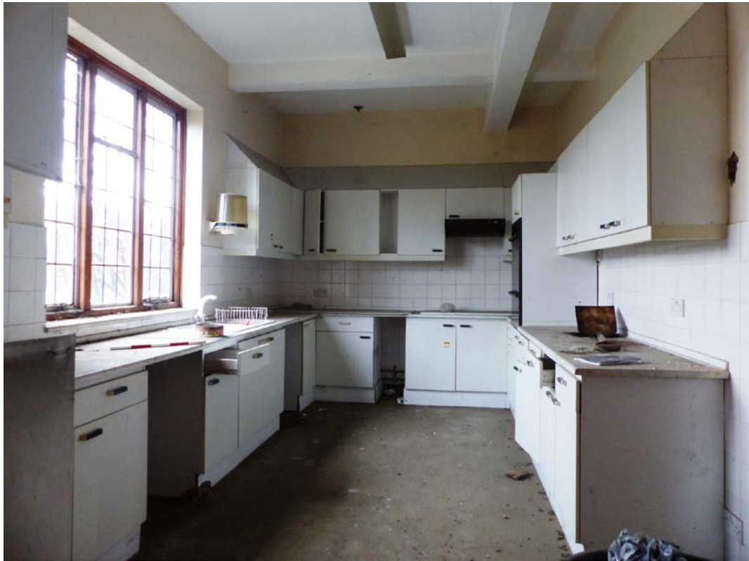
Fig 100 Interior of the kitchen (G4), looking east
