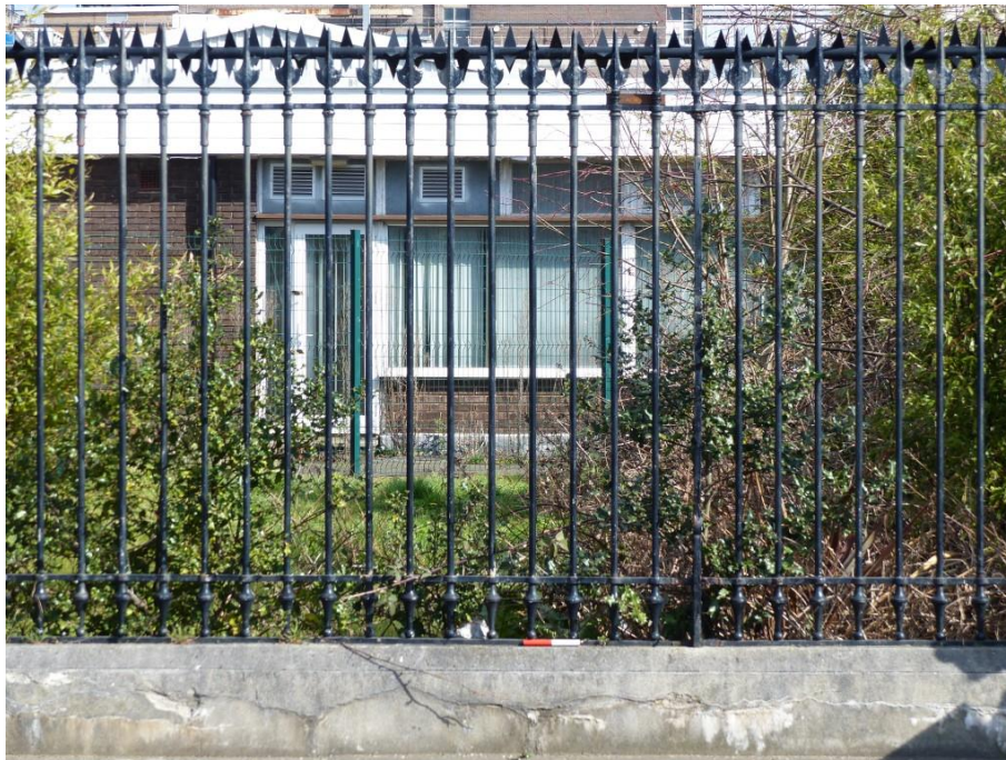
Fig 125 Railing Type A, looking north
