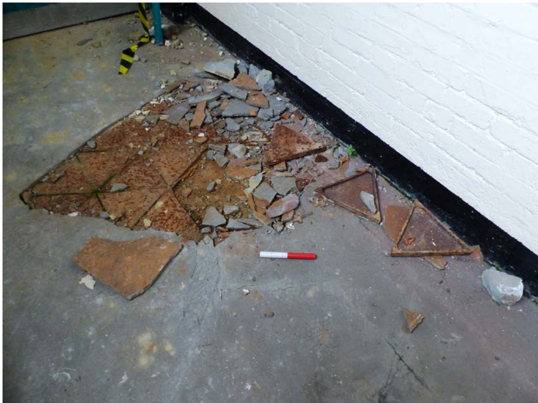
Fig 36 Steel triangular blocks formed the forklift route
