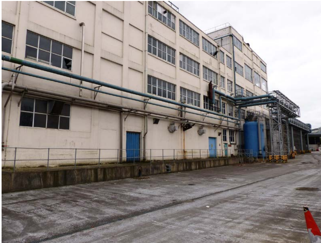
Fig 25 West end of the north facing rear elevation of the factory building
