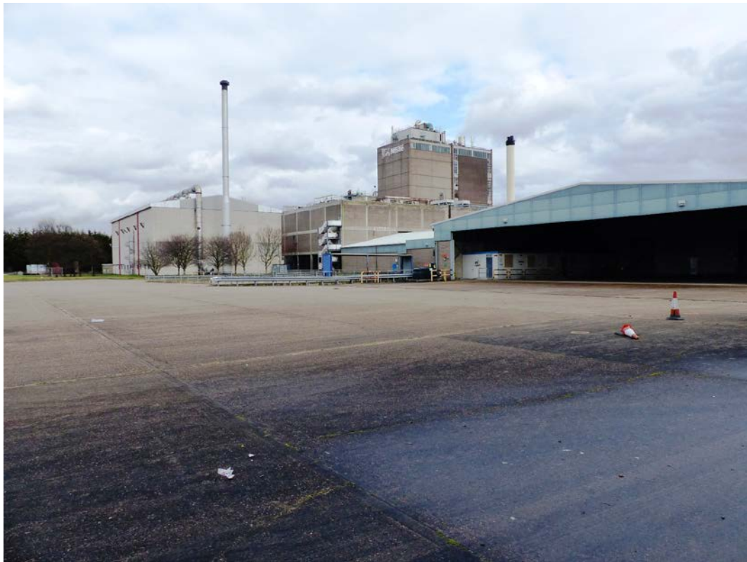
Fig 151 Large concrete surfaced car park at the west end of the site, looking north-east
