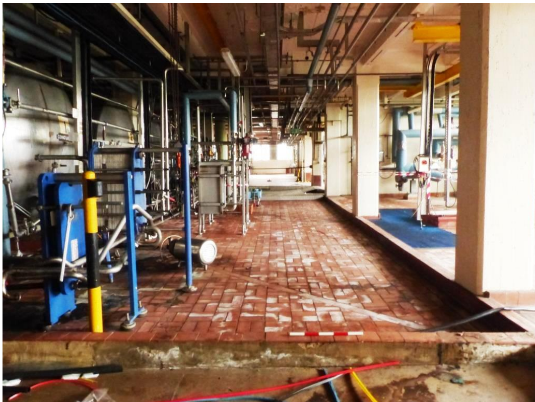
Fig 50 Room 1F49 looking west
