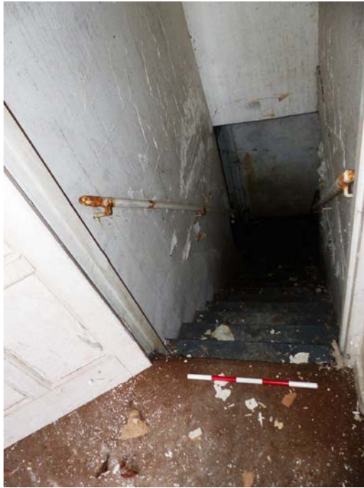
Fig 102 Staircase leading to the basement
