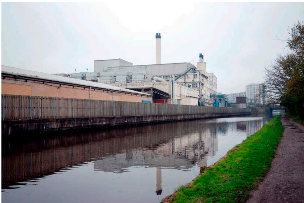
Fig 152 The factory buildings as seen from the canal path
