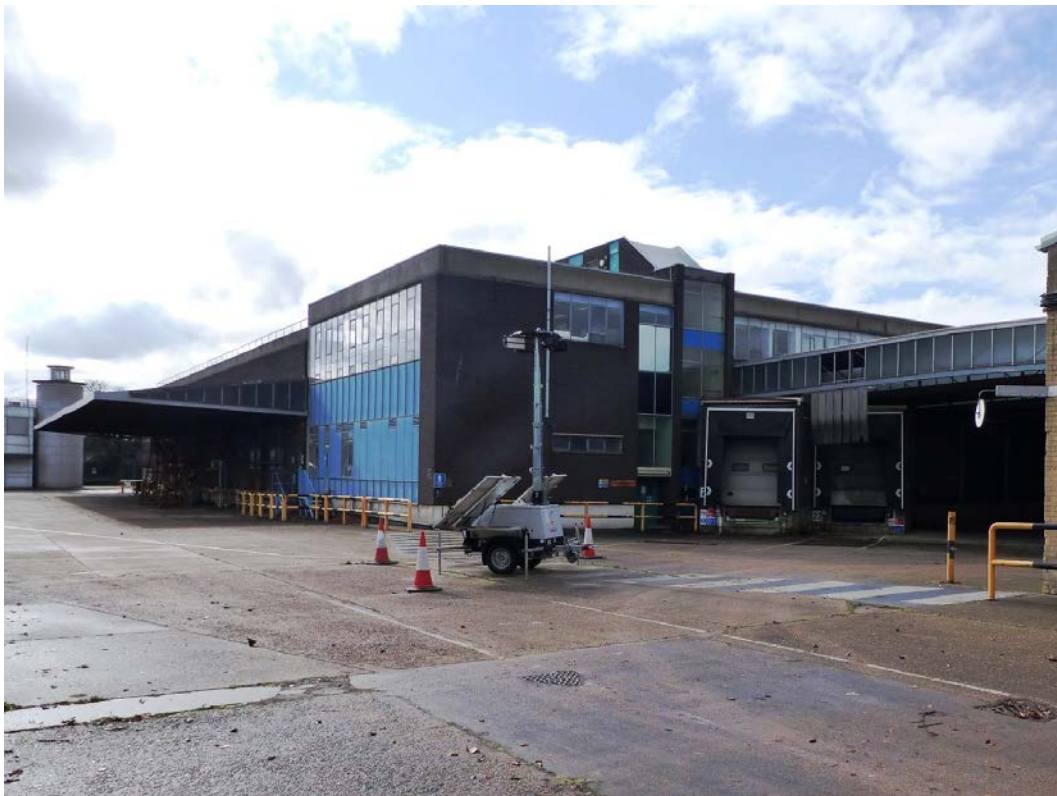
Fig 144 Later added factory building located on the east side of the site with a cantilevered canopy, looking south
