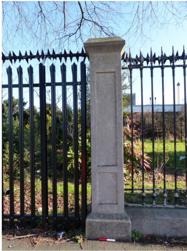
Fig 136 Post Type A, looking north
