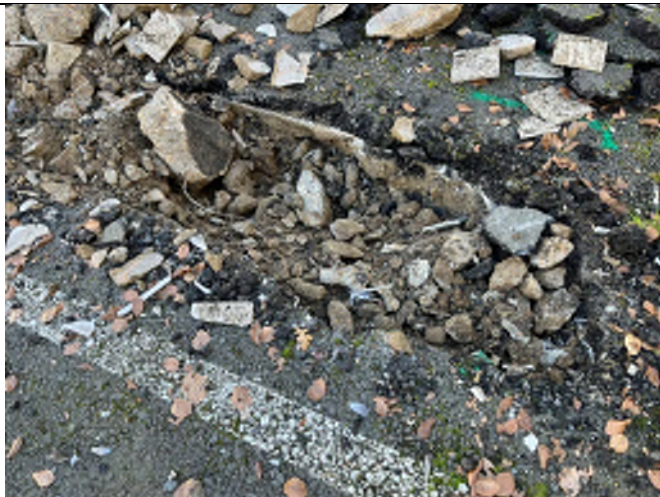
TP203 breaking out of hardstanding
