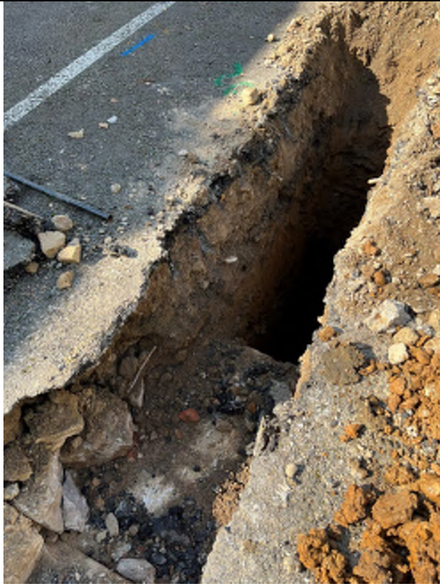
TP202 complete trial pit
