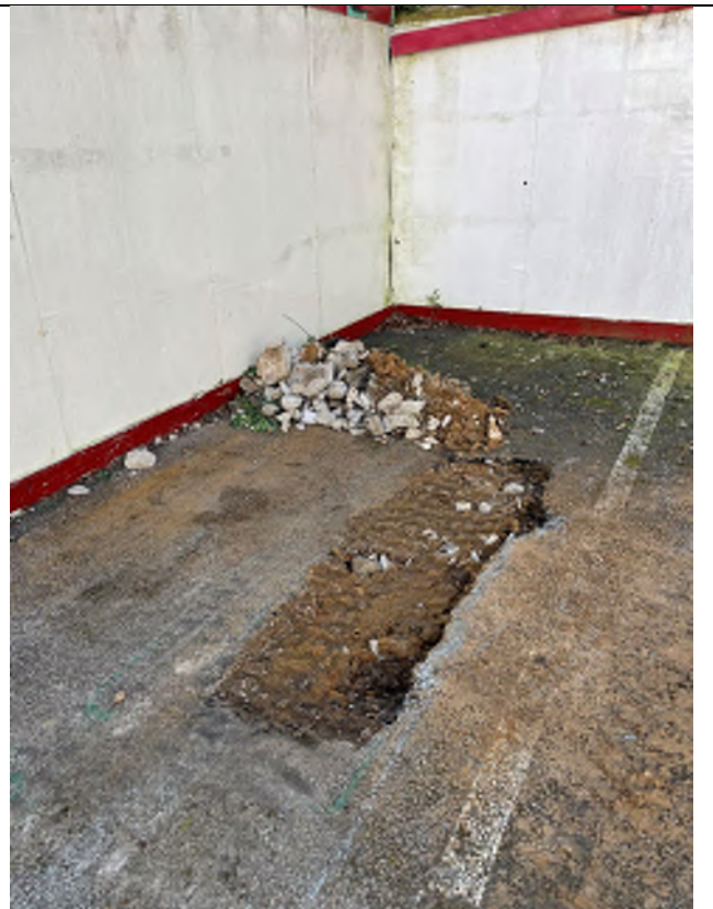
Trial pit reinstatement
