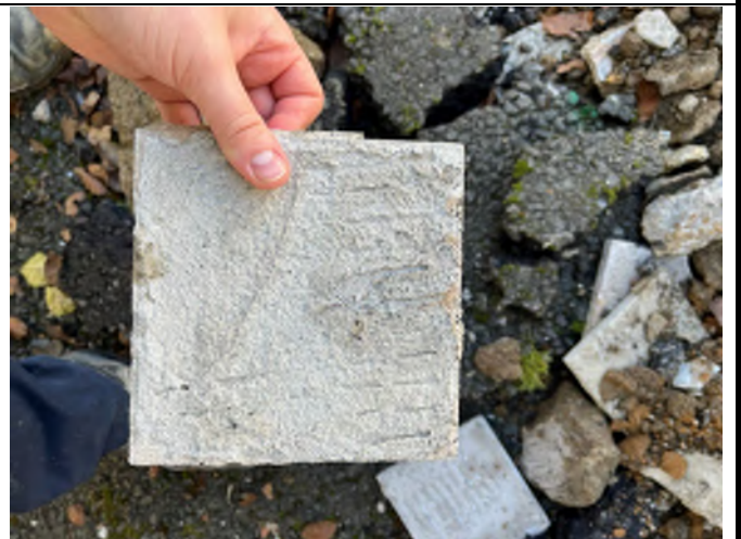
TP203 tiling found immediately below hardstanding
