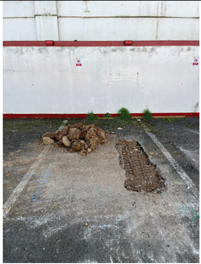
Trial pit reinstatement
