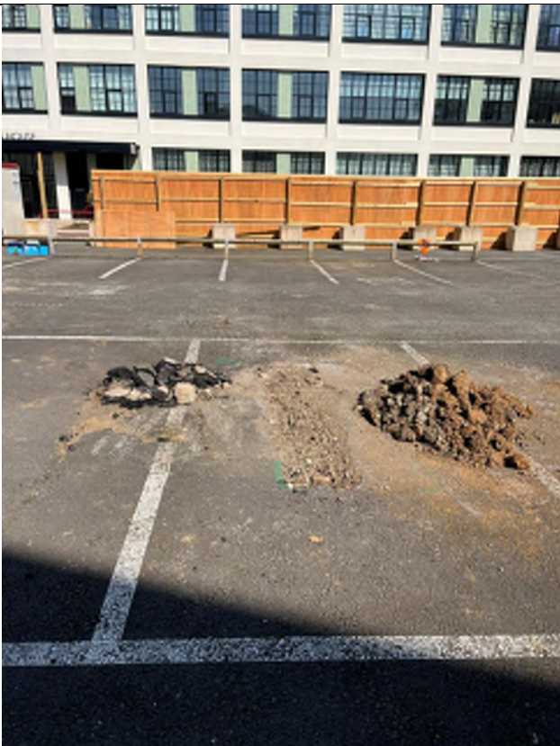
Trial pit reinstatement
