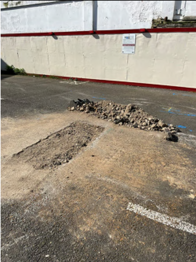
Trial pit reinstatement
