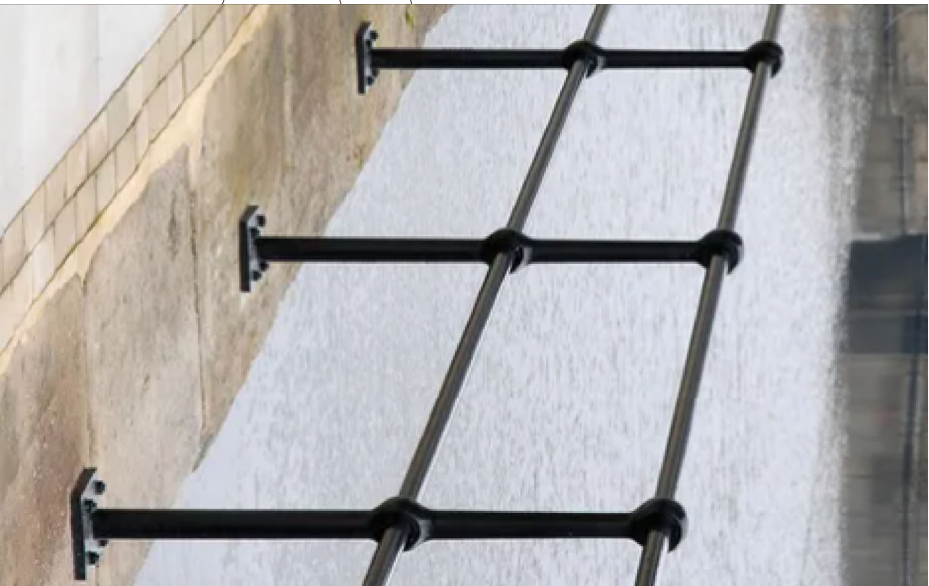
25m LONG x 1.1m HIGH WITH MID RAIL BLACK HANDRAIL TO PROVIDE A PEDESTRIAN BARRIER TO THE TRAFFIC ISLAND AND BARRIER SYSTEM. HANDRAIL TO MATCH CANAL PROTECTION HANDRAIL.
