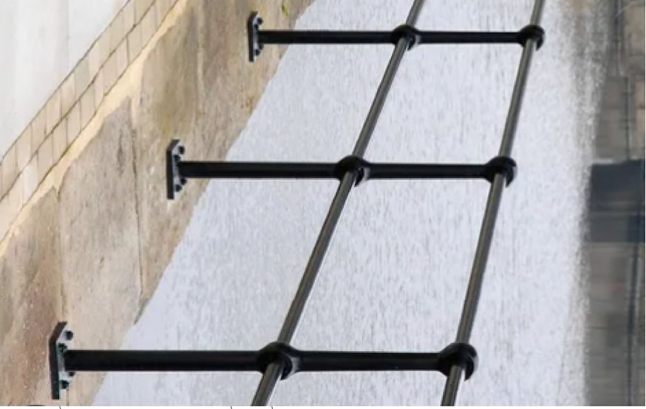
6.5m LONG x 1.1m HIGH WITH MID RAIL BLACK HANDRAIL TO PROVIDE A PEDESTRIAN BARRIER TO THE TRAFFIC ISLAND AND BARRIER SYSTEM. HANDRAIL TO MATCH CANAL PROTECTION HANDRAIL.
