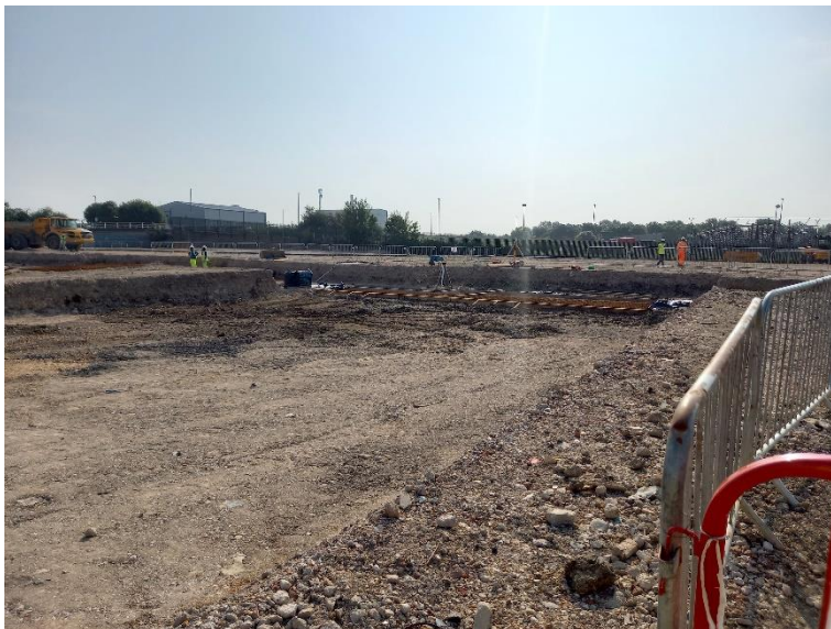
Excavation for loading dock to units 2 and 3.
