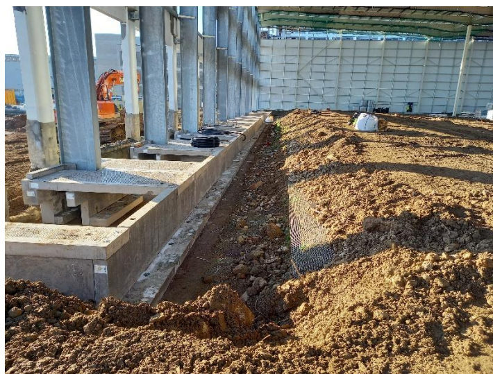
Unit 4 – excavations behind retained façade.
