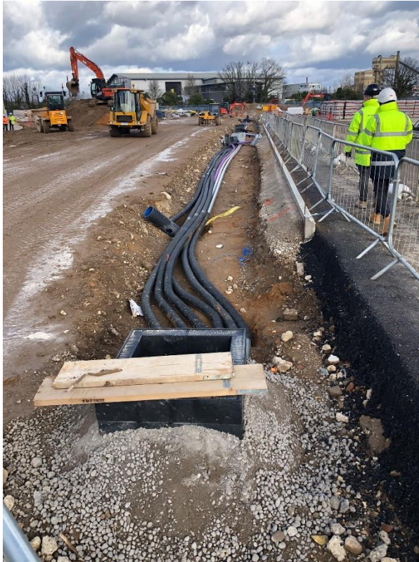
Utility installation below estate road.
