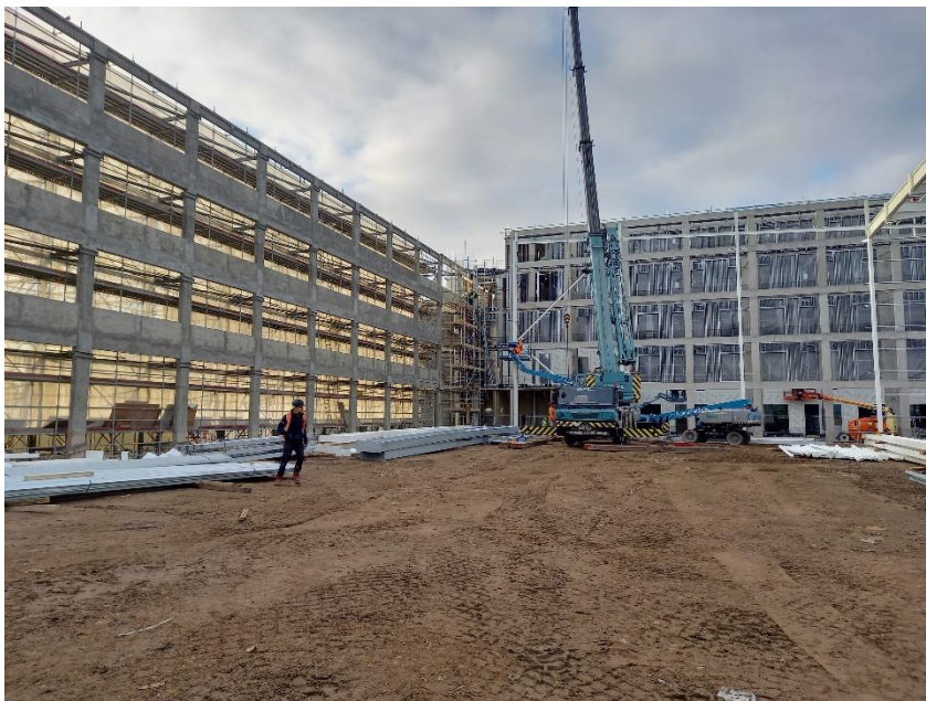
Unit 4 behind retained facade
