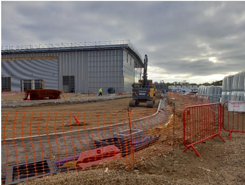
Estate road construction (with unit 3 in background)
