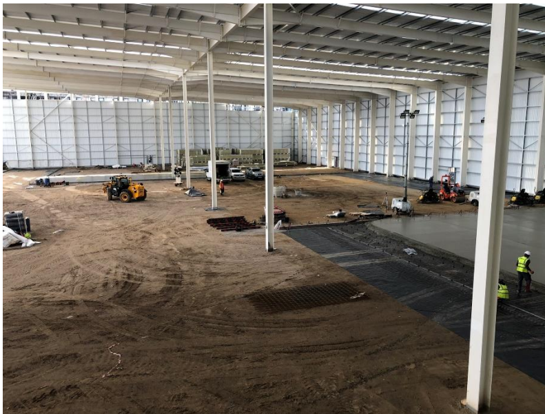
Unit 4 – floor slab installation
