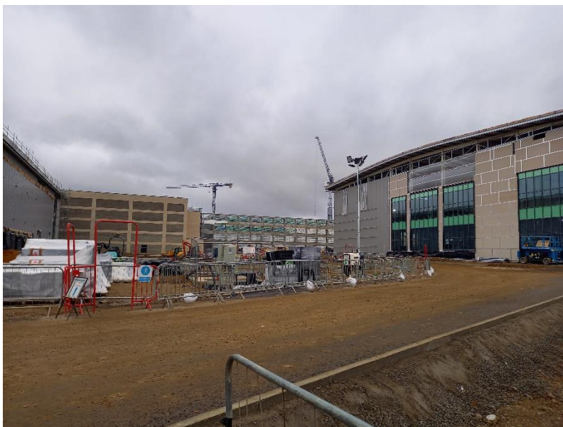
General site view: unit 1 to left; unit 4 centre; units 2/3 to right
