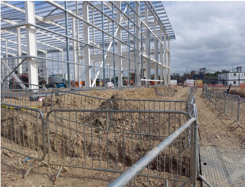
Excavation for loading dock to units 4.
