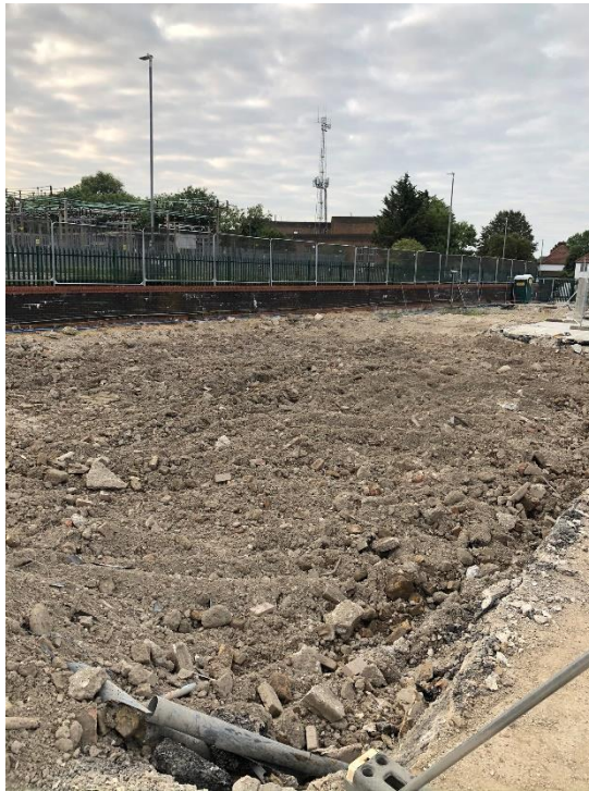
Removal of remnant hard surfacing on northern boundary
