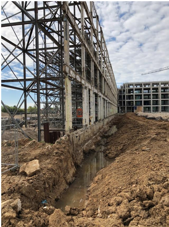
Excavations in front of Unit 4 retained facade
