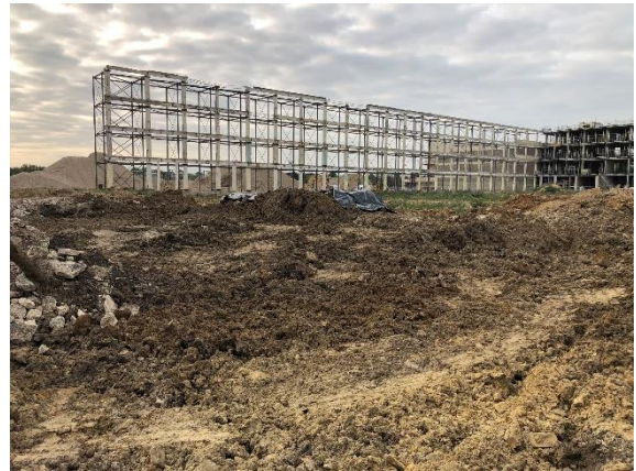
Ongoing earthworks for Unit 4
