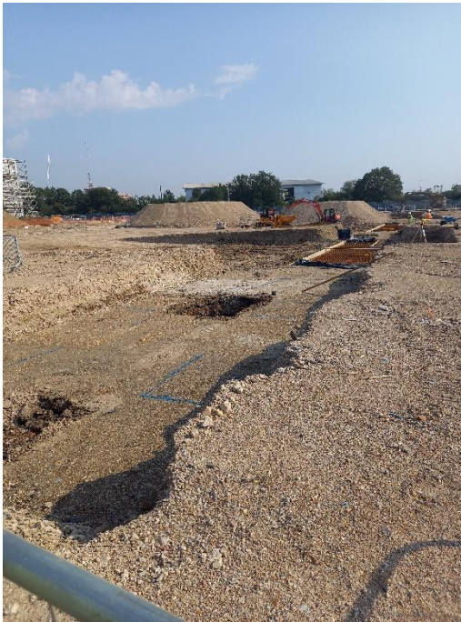
Foundation excavations for units 2 and 3.
