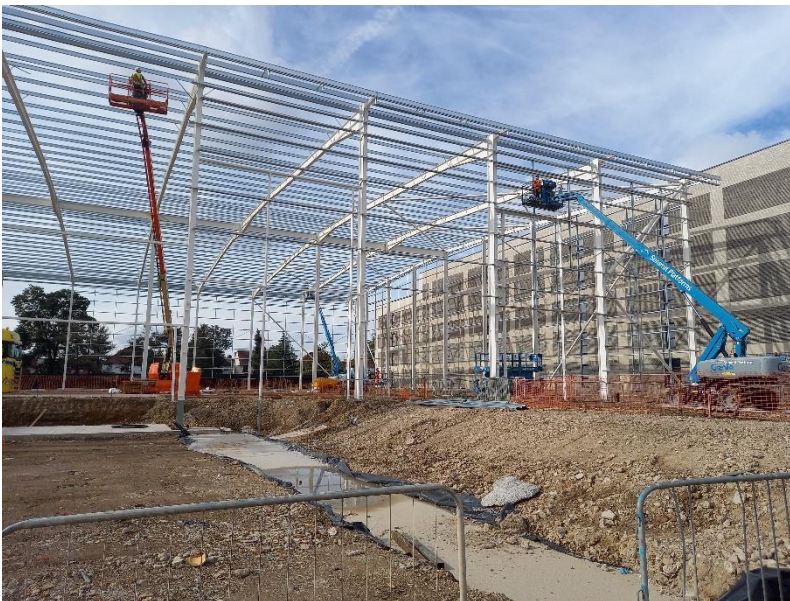
Excavation for loading dock to unit 1.
