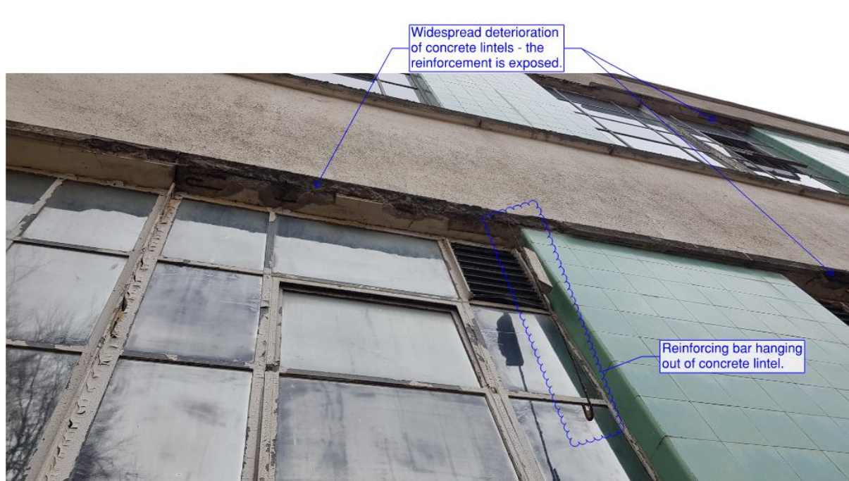
Figure 2: Image of south elevation showing lintel deterioration
