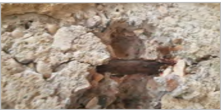
P8b: BAR EXPOSED AT BREAKOUT B/O C
