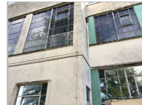
P1e: VERTICAL CRACK TO EXTERNAL COLUMN AB
