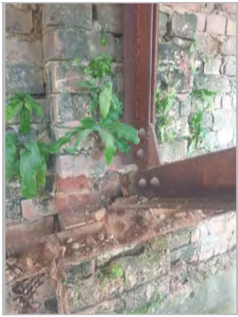
P11a: BOTTOM CONNECTION OF TRUSS K3
