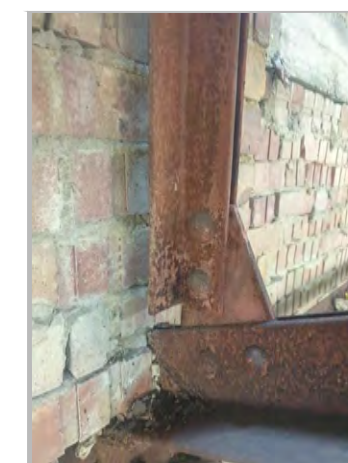
P21b: BOTTOM CONNECTION OF TRUSS G10
