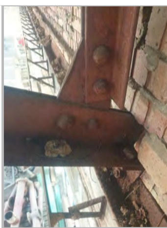
P24a: BOTTOM CONNECTION OF TRUSS H10
