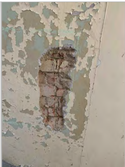
P1g: CRACK INVESTIGATION - SURVEY AREA RR4
