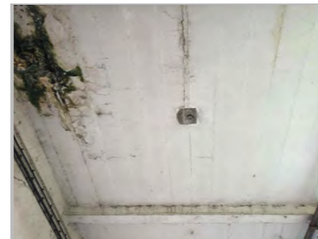
P1d: WATER SEEPAGE, CRACK AND MOSS GROWTH - GRID Q-P/10-11
