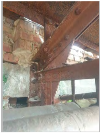
P11b: TOP CONNECTION AT TRUSS K3
