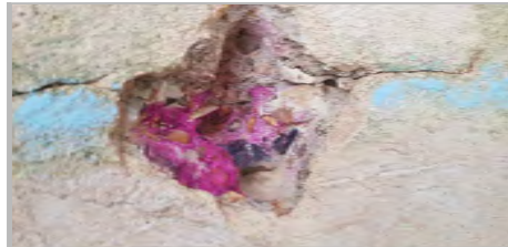
P11b: BAR EXPOSED AT BREAKOUT B/O D
