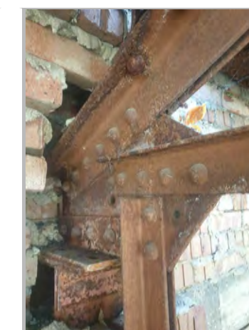
P21c: TOP CONNECTION AT TRUSS G10
