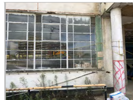
P1k: SPALLING TO WINDOW STRUCTURE AT WESTERN FACE OF BUILDING
