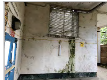
P1g: CRACK AND WATER INGRESS TO WALL R/10-11
