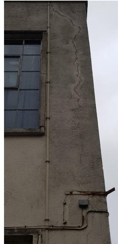
Photo 11: Crack through render on south-west corner of building
