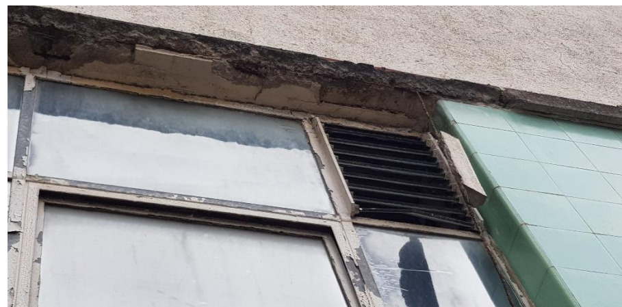
Photo 14: Façade lintel spalling with reinforcement dislodged.
