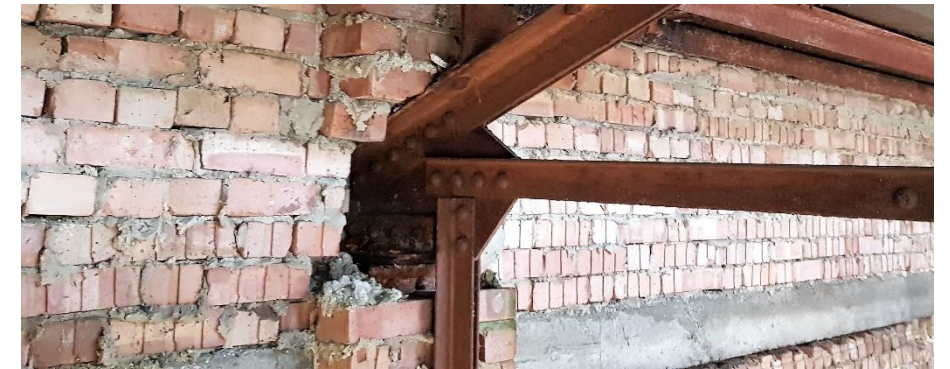
Photo 6: Canteen hall truss embedded in brickwork.
