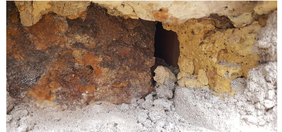
Photo 12: Steel column exposed within brick encasement.
