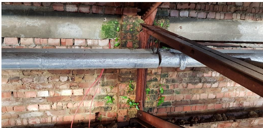
Photo 7: Roof truss embedment into brickwork under box gutter.
