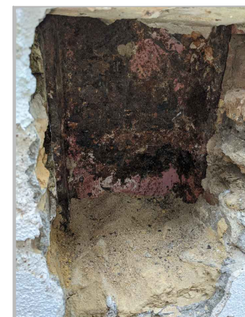
P1m: CL4 CLOSER VIEW OF COLUMN FLANGES WEB
