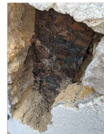
P1n: CL4 CLOSER VIEW OF COLUMN FLANGE
