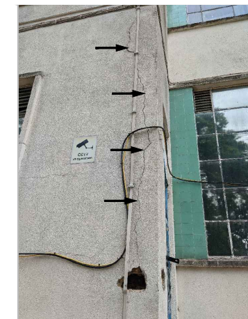
P1g: CL3 COLUMN EXPOSURE AND CRACKING
