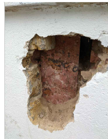
P1a: CL1 COLUMN EXPOSURE
