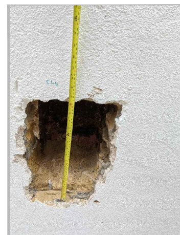
P1l: CL4 EXPOSURE TO COLUMN FLANGE AND WEB
