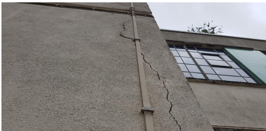
Photo 13: Crack through render on south elevation
