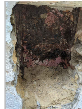
P1m: CL4 CLOSER VIEW OF COLUMN FLANGES WEB
