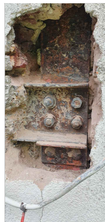
P2c: B2 BEAM TO COLUMN CONNECTION EXPOSURE
