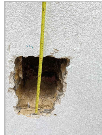
P1l: CL4 EXPOSURE TO COLUMN FLANGE AND WEB
