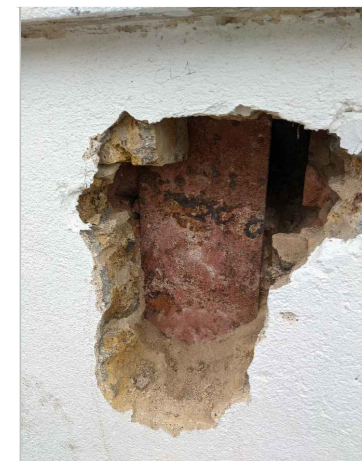
P1a: CL1 COLUMN EXPOSURE
