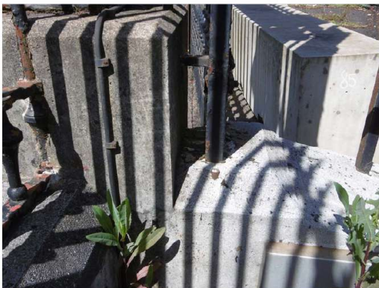
Fig 12: Western gate corner post with accompanying concrete support
