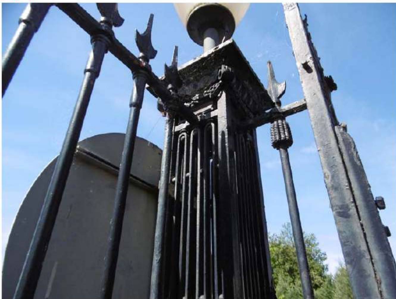
Fig 13: Western gate corner post with lamp and decorative detail, looking west
