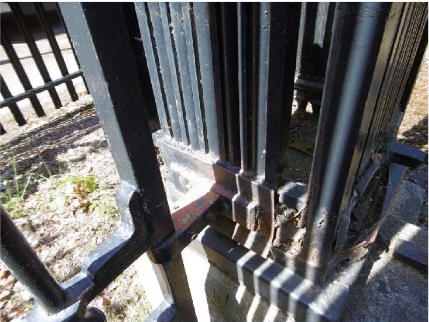
Fig 3: Central gate corner looking south, exposed metal frame in concrete base
