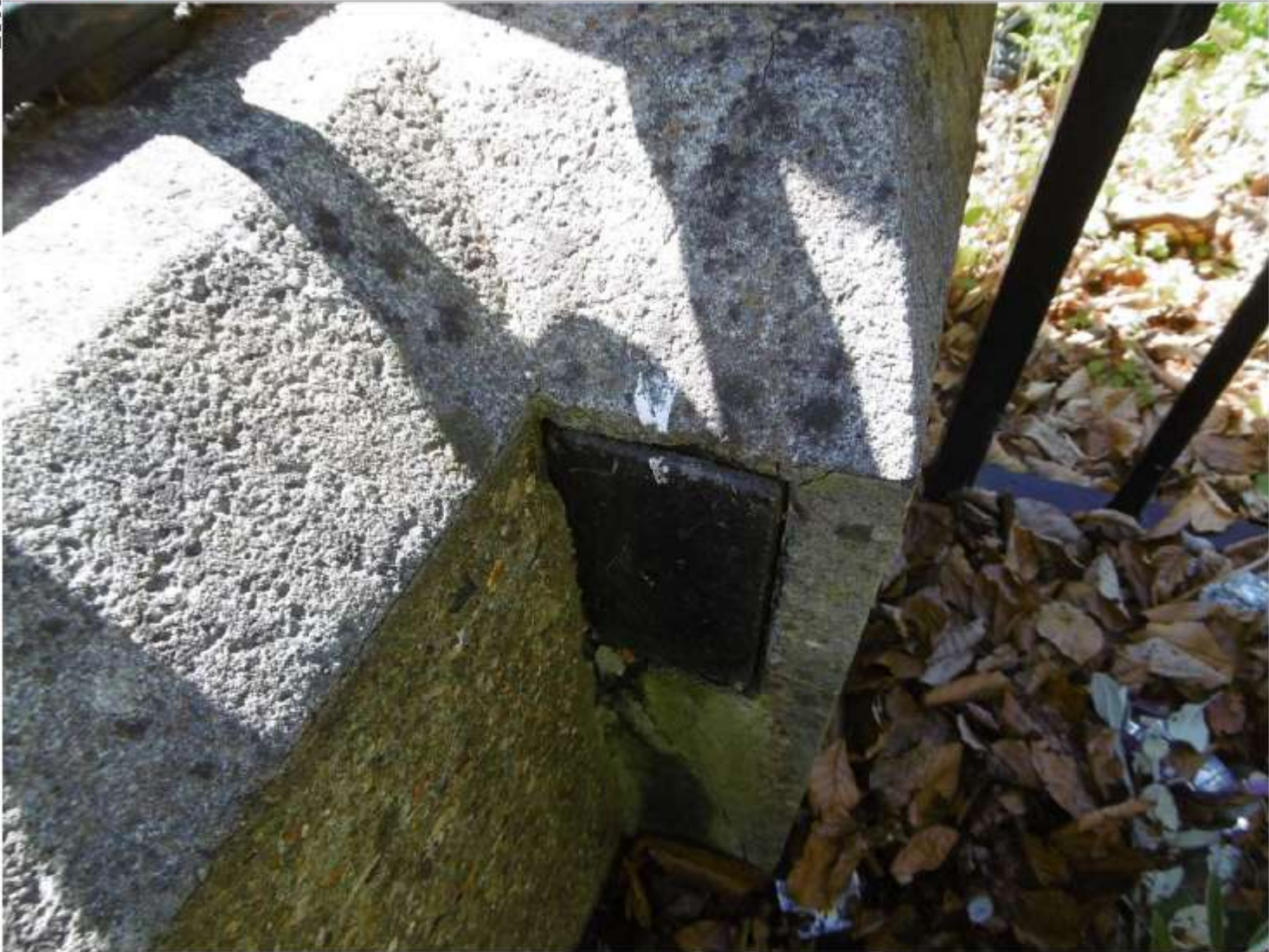
Fig 3: Central gate corner looking south, exposed metal frame in concrete base
