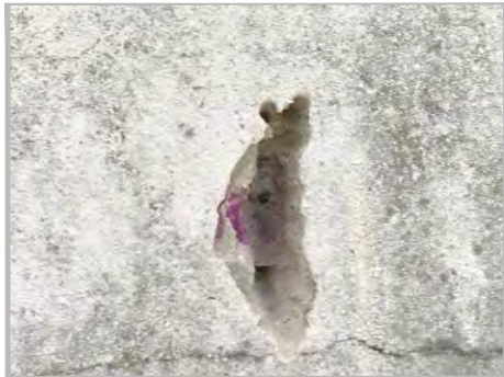
P8b: CLOSE UP VIEW OF BEAM C/10-11
