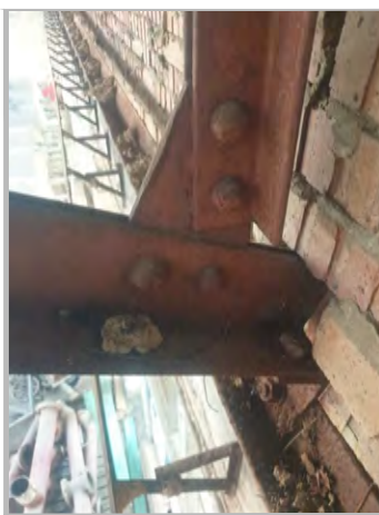
P24a: BOTTOM CONNECTION OF TRUSS H10
