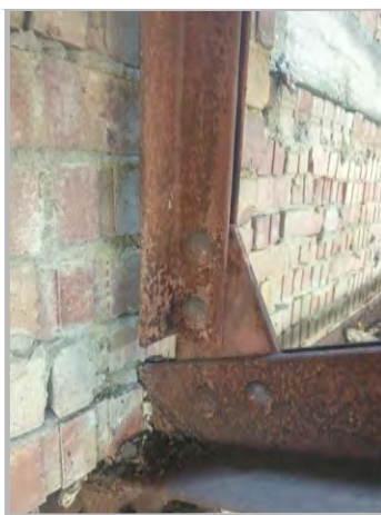
P21b: BOTTOM CONNECTION OF TRUSS G10
