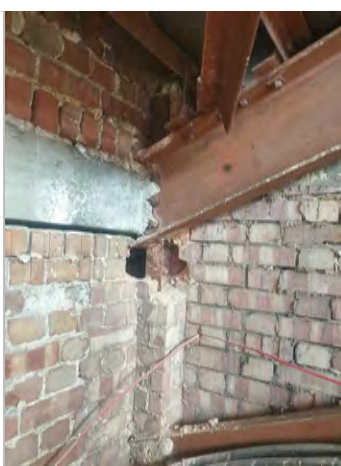
P2a: TRUSS D3 END CONNECTION
