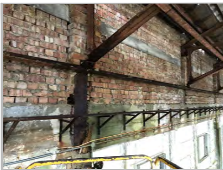
P5a: TRANSFER BEAM G-H/10
