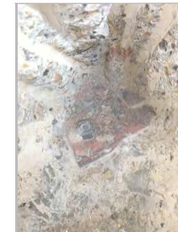
P2b: CLOSE UP VIEW OF BASE PLATE AT BOTTOM OF TRIAL PIT TP1
