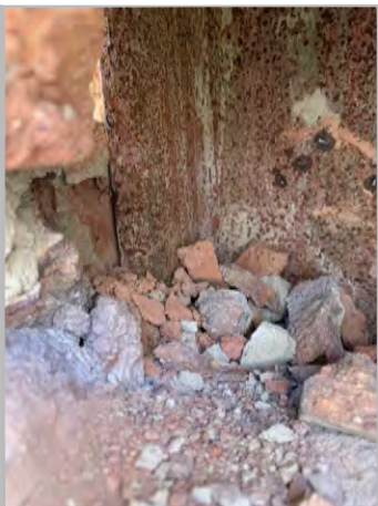
P23b: CLOSE UP VIEW OF COLUMN Q3
