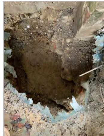
P8b: LOOKING DOWN AT FOUNDATION AT BASE OF TRIAL PIT TP3
