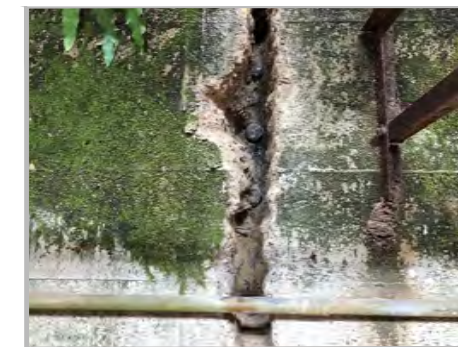
P11c: CLOSE UP VIEW OF BOTTOM OF TRANSFER BEAM K3
