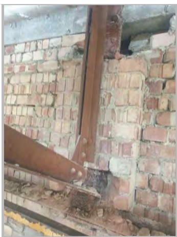
P8a: BOTTOM CONNECTION OF TRUSS J3
