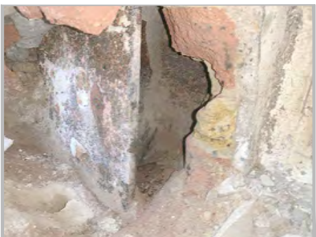
P11b: CLOSE UP VIEW OF COLUMN E10
