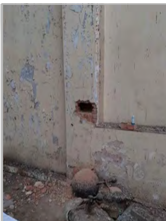
P7a: COLUMN C8
