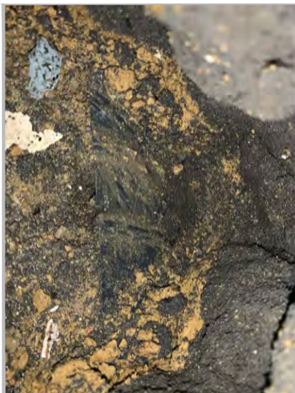
P1h: CRACK INVESTIGATION - SURVEY AREA RR9
