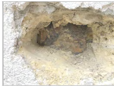
P2b: CLOSE UP VIEW OF COLUMN A5
