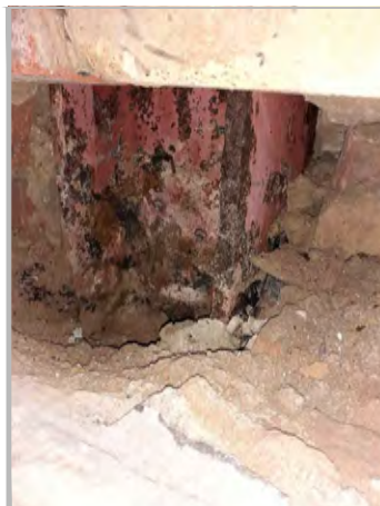
P8b: CLOSE UP VIEW OF COLUMN C10
