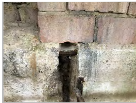
P8b: CLOSE UP VIEW OF TRANSFER BEAM J-K/3
