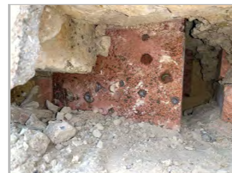
P19b: CLOSE UP VIEW OF COLUMN L1
