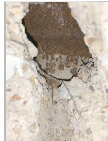
P5b: CLOSE UP VIEW OF PRIMARY BEAM E/1-3
