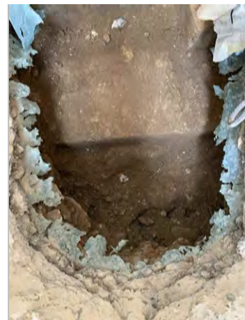
P5b: LOOKING DOWN AT FOUNDATION AT BASE OF TRIAL PIT TP2
