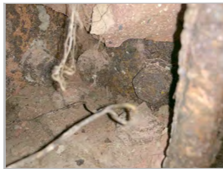
P5b: CLOSE UP VIEW OF TRANSFER BEAM G-H/10
