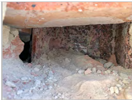
P26b: CLOSE UP VIEW OF COLUMN S3
