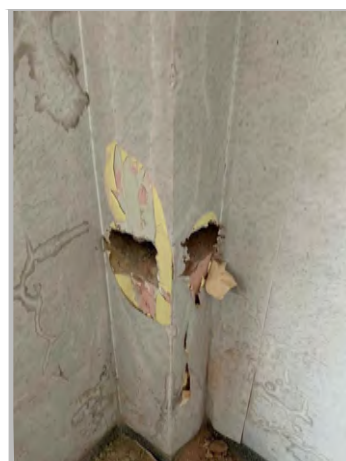
P4a: COLUMN C1
