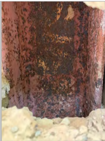
P22b: CLOSE UP VIEW OF COLUMN N11
