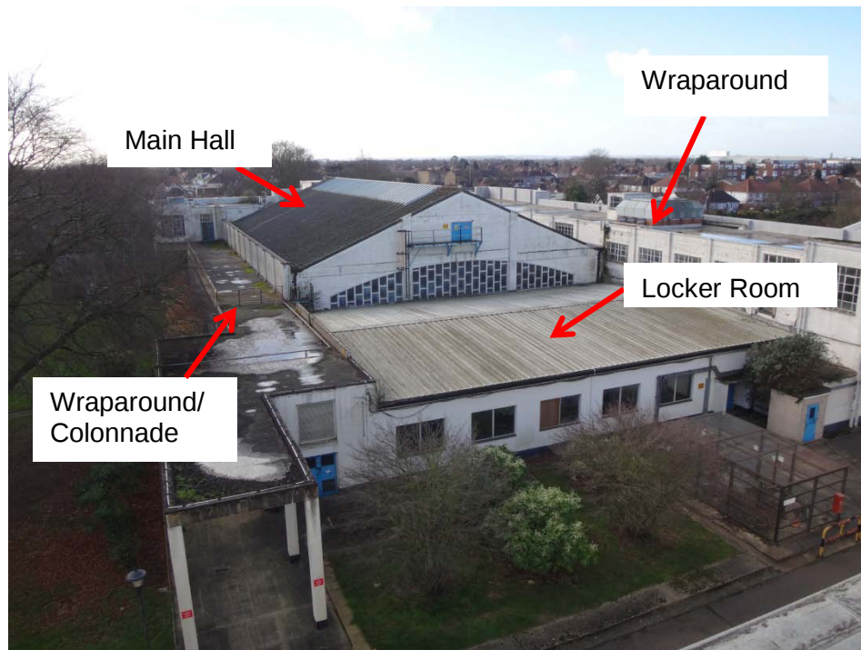
Aerial view of the former canteen building showing the northern elevation and various portions of the building
