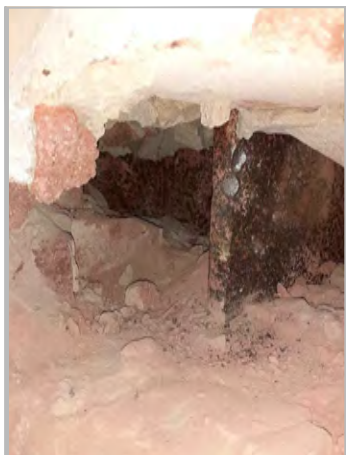
P6b: CLOSE UP VIEW OF COLUMN C3
