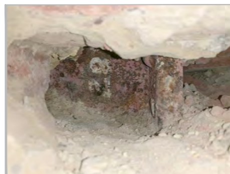
P4b: CLOSE UP VIEW OF COLUMN C1
