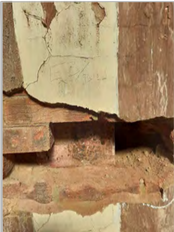
P10b: CLOSE UP VIEW OF COLUMN E3
