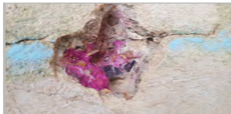
P11b: BAR EXPOSED AT BREAKOUT B/O D
