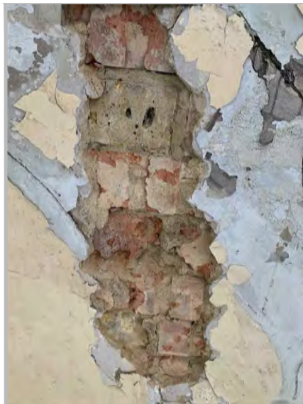
P1a: DPC INVESTIGATION - SURVEY AREA RR2
