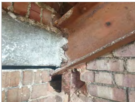
P2b: CLOSER VIEW OF TOP CONNECTION AT TRUSS D3
