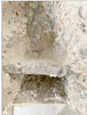
P6b: CLOSE UP VIEW OF PRIMARY BEAM G/2-3
