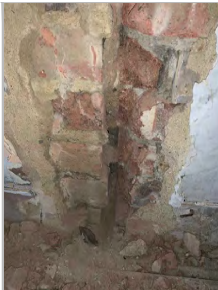
P1c: DPC INVESTIGATION - SURVEY AREA RR11
