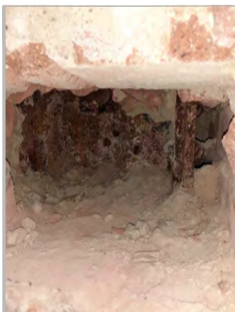
P7b: CLOSE UP VIEW OF COLUMN C8
