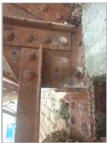
P8b: TOP CONNECTION AT TRUSS J3
