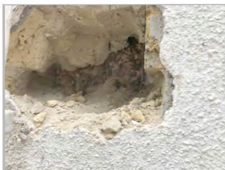
P3b: CLOSE UP VIEW OF COLUMN A12
