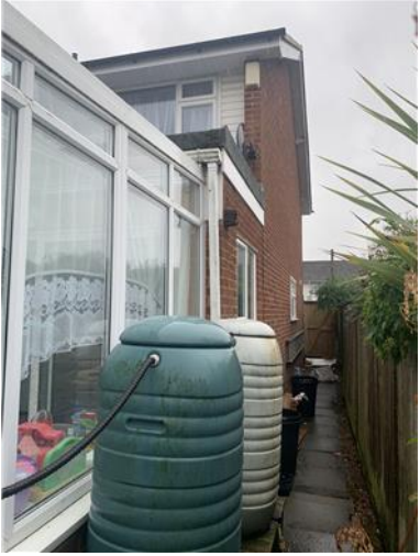
Views of the side alleyway
