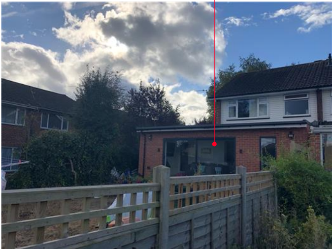
View from rear garden looking at the neighbour's recently built extension
