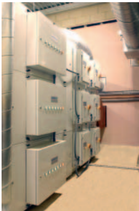
Six ESP and Three UV-C modules installed as an integrated system.
