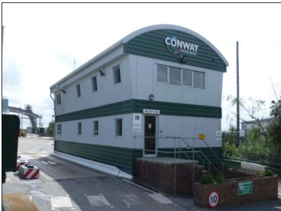
Figure 10.1: Erith Weighbridge Office
