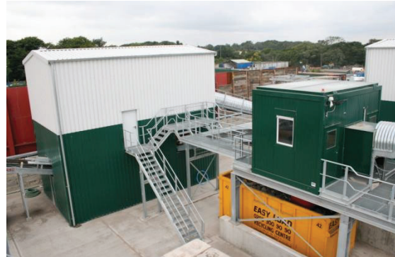
Arising fed into our static crusher housed in an acoustic silenced building
