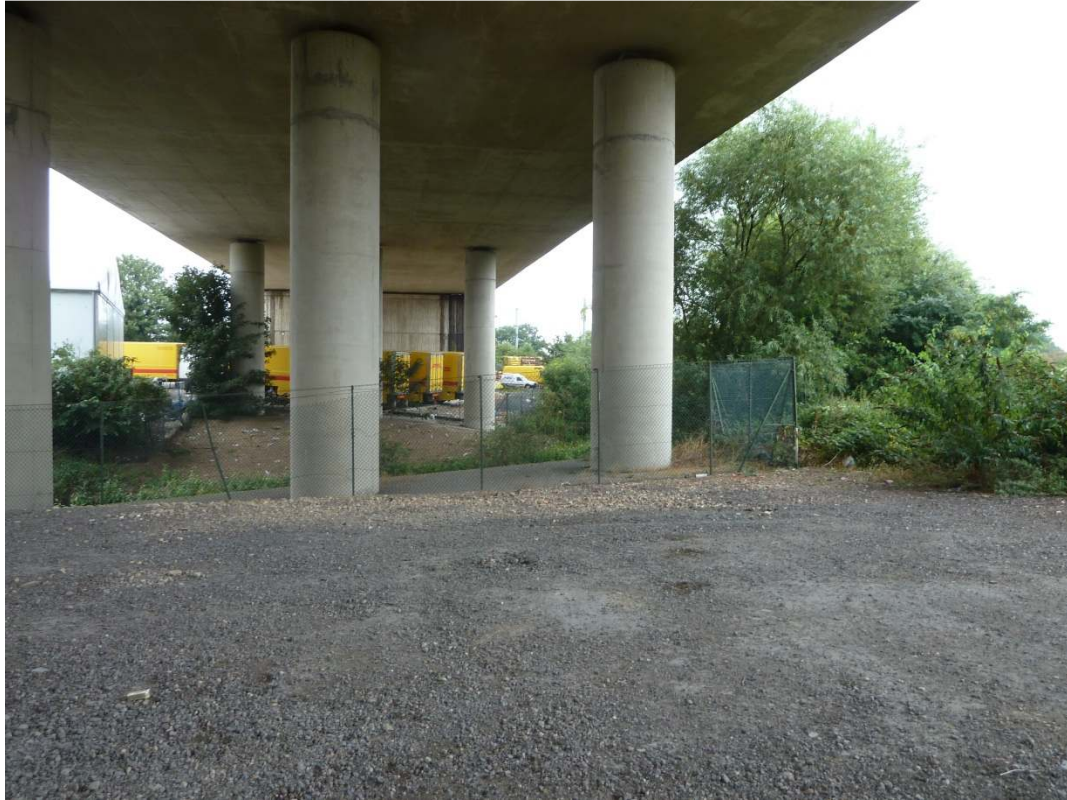
View of the proposed car parking area beneath the flyover looking north
