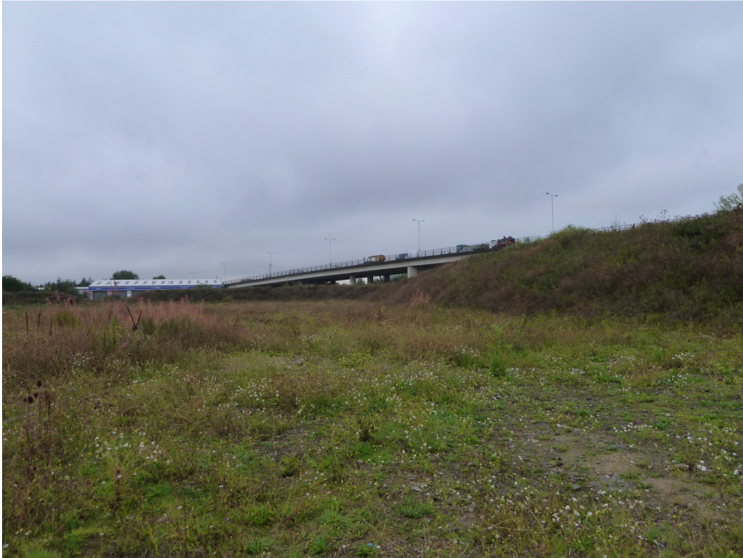
View across the site looking south
