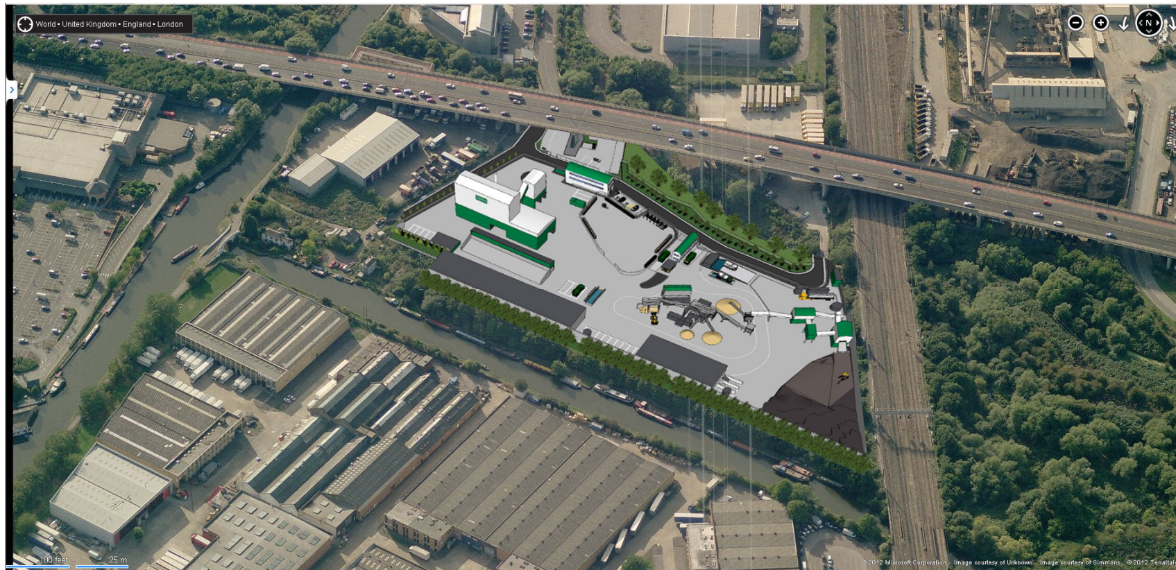
Aerial CGI view looking west
