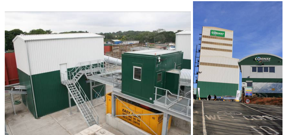
Fig 12 – Use of attenuation and enclosures at FM Conway existing sites
