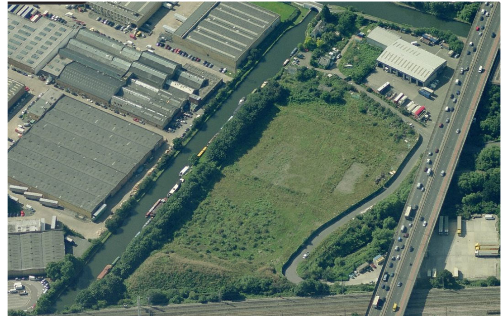
Fig 2 – Aerial View of the site from the north (approx. 5 years old)
