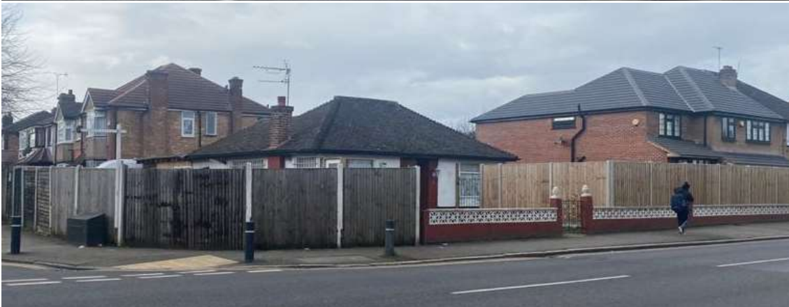
Photograph of existing bungalow looking south from North Hyde Road
