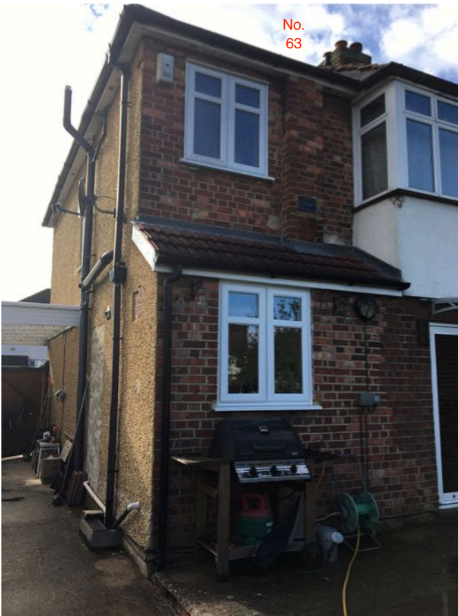
View of the side and rear elevation (detail)
