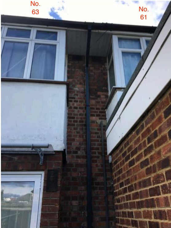
View of the rear elevation (detail)
