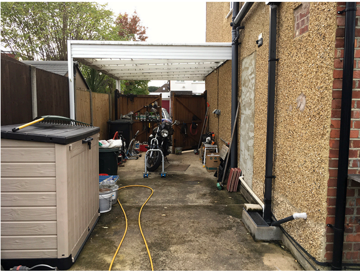
View of the canopy on the side
