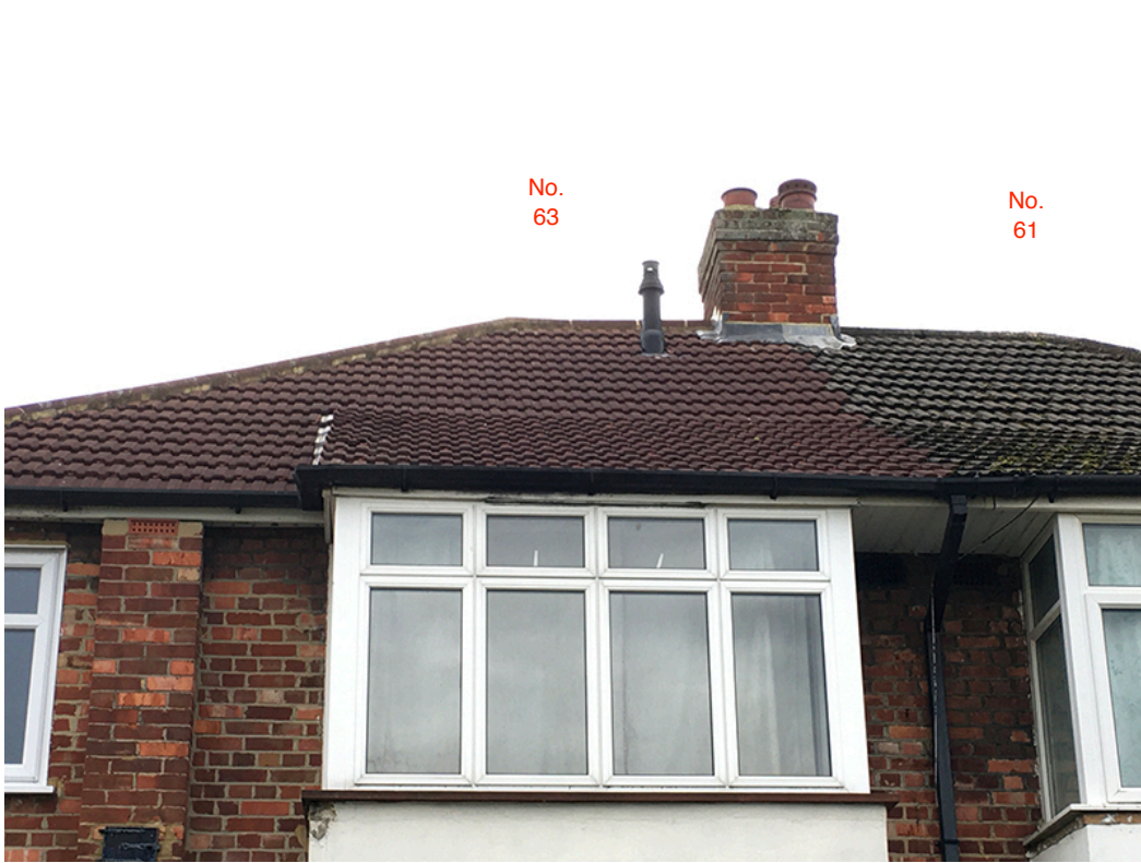
View of the rear elevation (detail)
