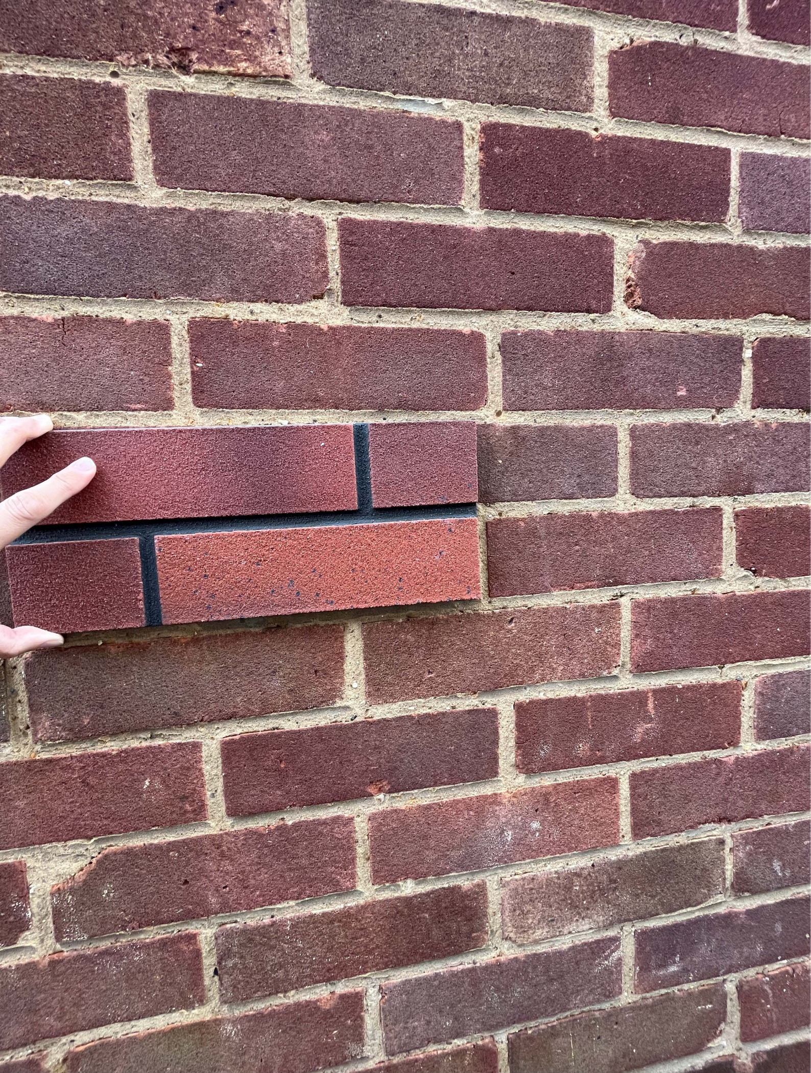
Bricks manufactured by Izoflex and the colour is 6073 Porto. In order to match the existing, the proposed mortar will be beige 205.
