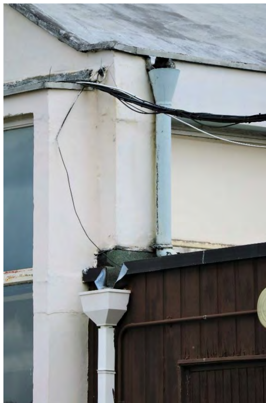
Fig 32 Detail showing the downpipes to the south-west of the structures
