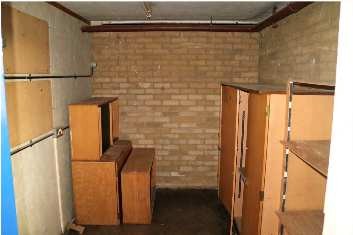
Fig 73 The storage room to the north of Building 5, looking north
