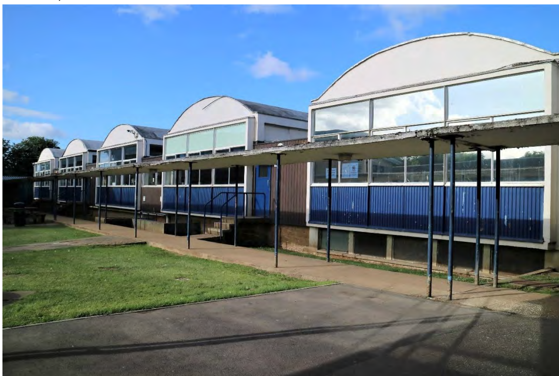
Fig 13 Block B, looking south-west
