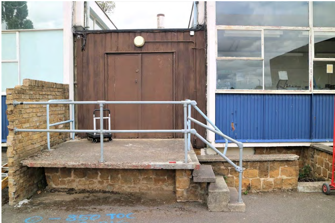
Fig 29 The low roofed partition with double doors between buildings 1 and 2, looking east
