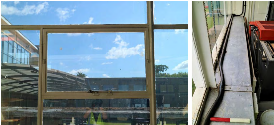
Fig 41 (Left) Detail of a pivoting window on the east elevation. (Right) Detail of an internal window sill
