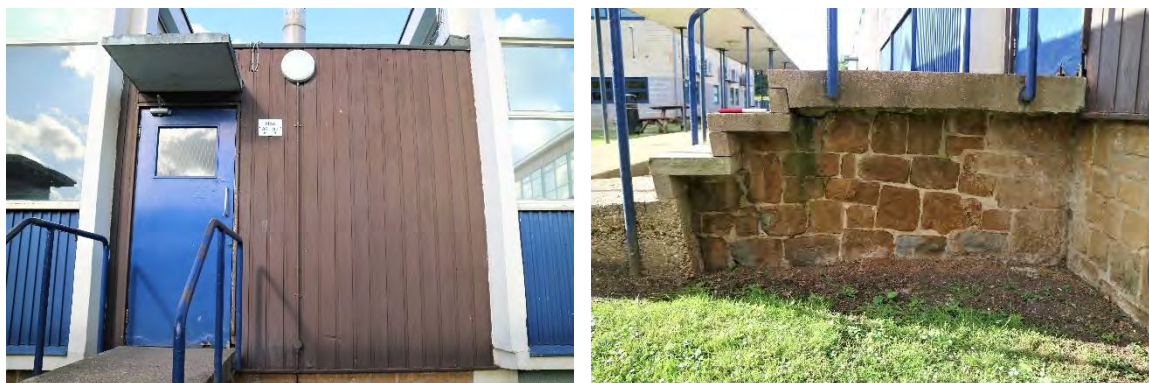
Fig 17 (Left) The low roofed timber clad partitions between each building, looking east. (Right) The stone and concrete steps which led to each door, looking south
