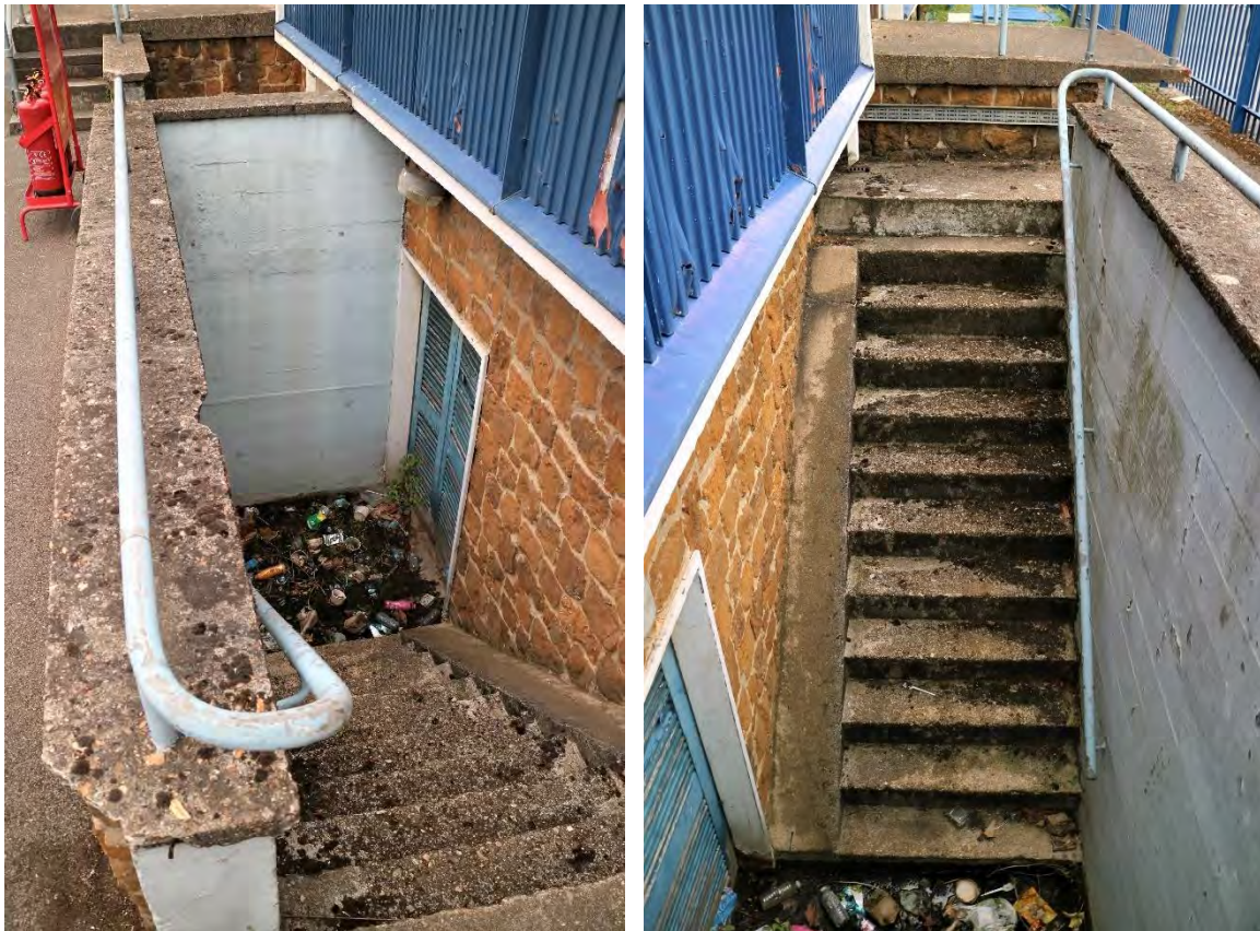
Fig 31 The basement access to the west of Building 2. (Left) Looking north. (Right) Looking south
