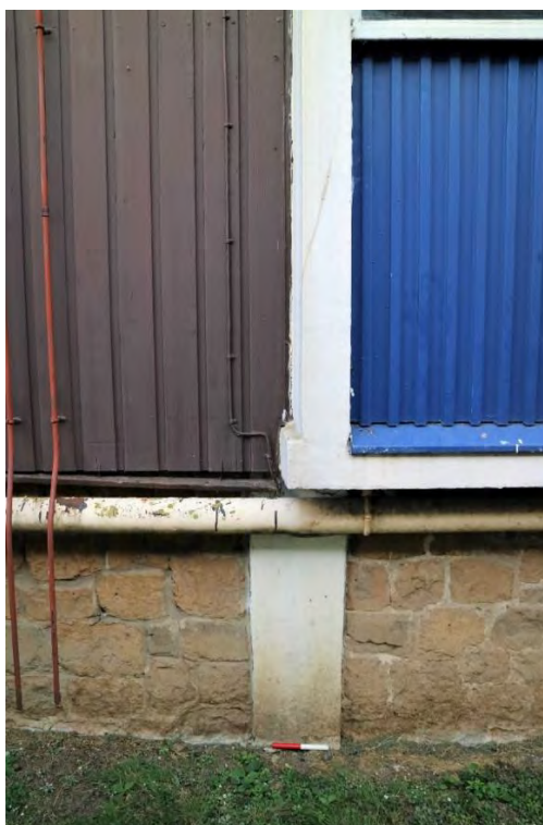
Fig 16 Detail showing the three types of cladding on the east elevation, looking west
