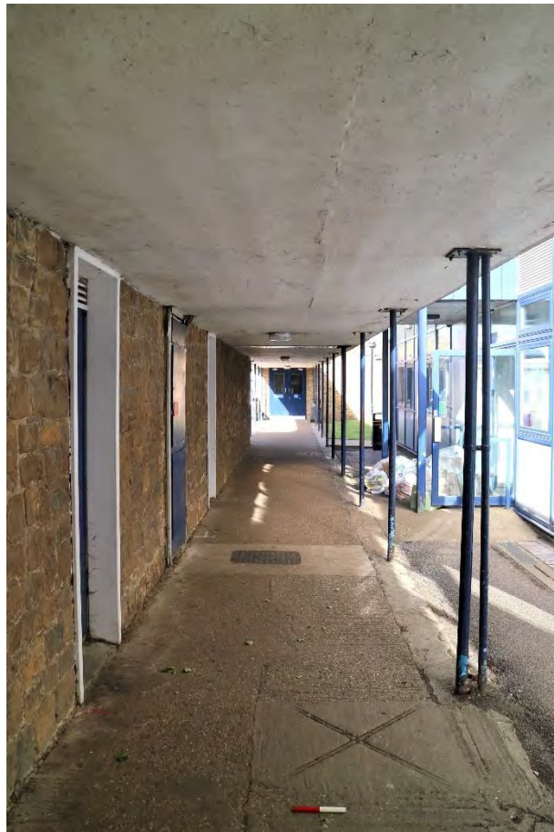
Fig 24 The path and awning which projected out from the north elevation, looking west
