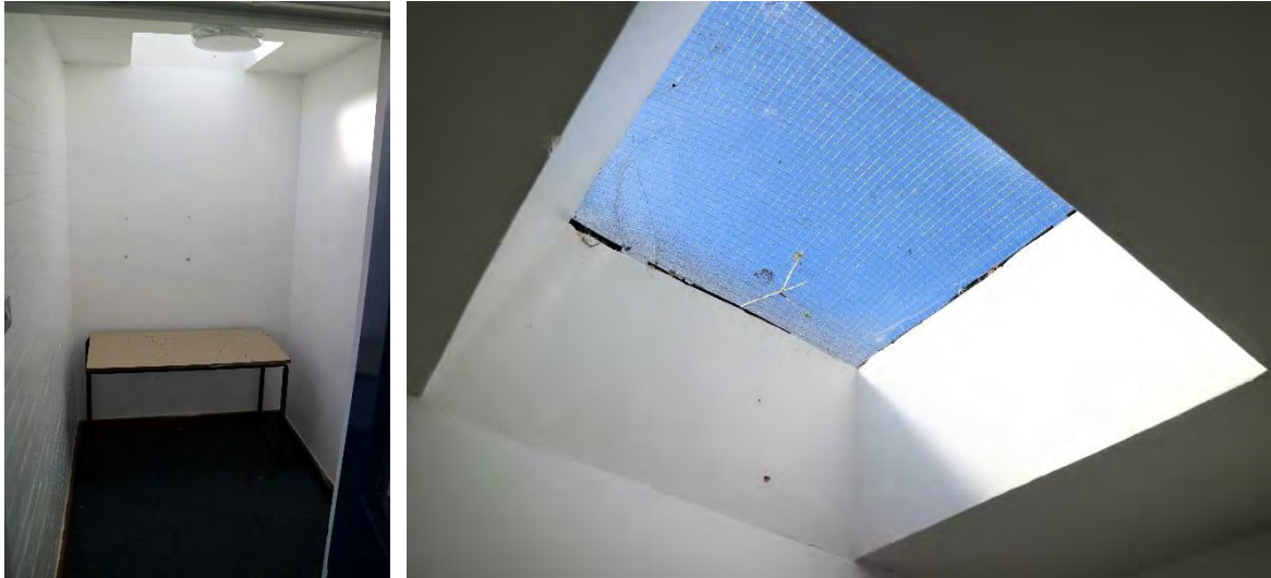
Fig 48 (Left) The office to the south-east of Building 1, looking south. (Right) Detail of the skylight above
