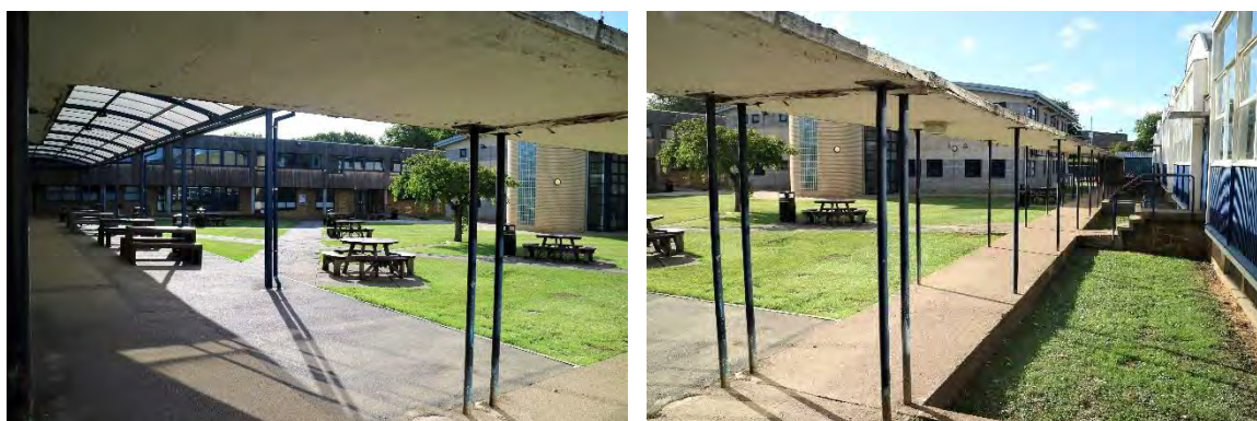
Fig 14 The courtyard to the south of Queensmead School. (Left) Looking south-east towards the classroom block also designed by YMR. (Right) Block B and its front to the courtyard, looking south
