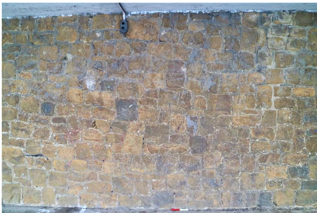
Fig 23 Detail showing the masonry cladding along the north elevation, looking south
