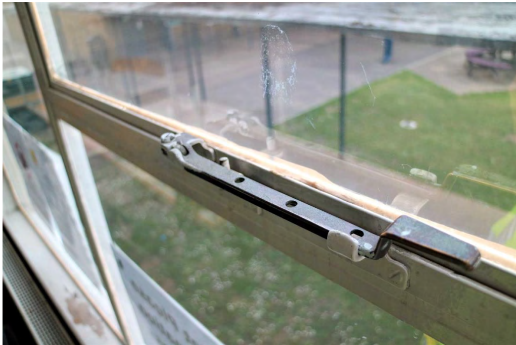
Fig 43 Detail of a window arm or catcher
