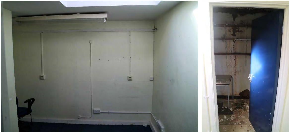
Fig 49 (Left) The office to the south of Building 1, looking south. (Right) A storage room, looking west
