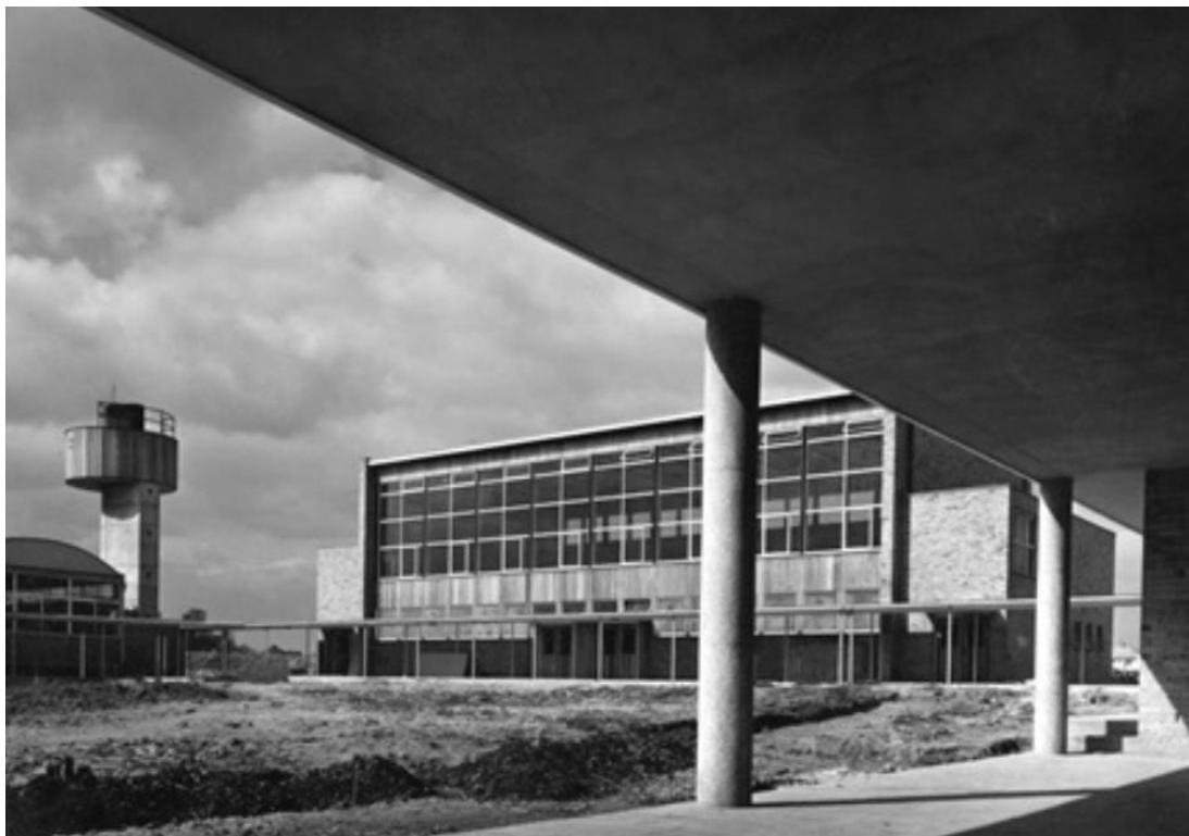
Fig 12 The gymnasium in 1953, looking north-west. Image: RIBA44280 RIBA Architecture
