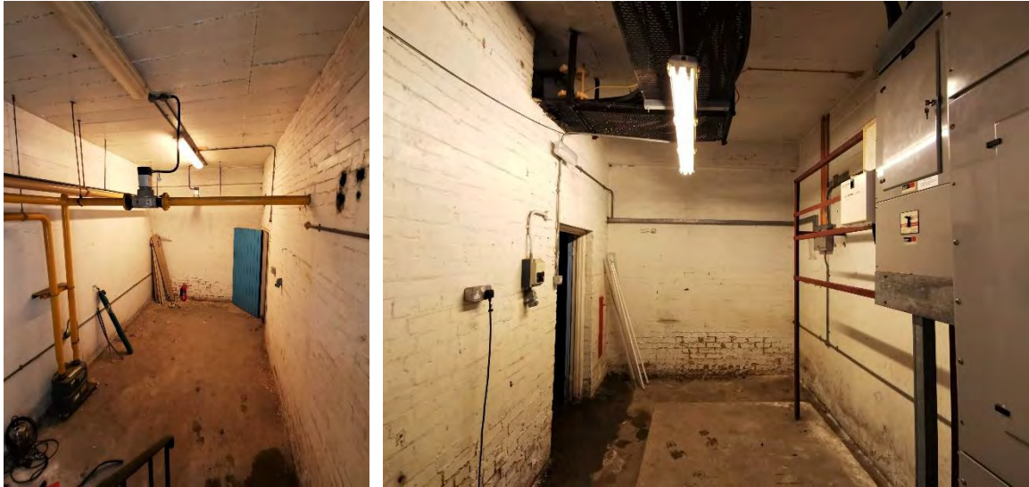
Fig 37 (Left) The eastern corridor, looking west. (Right) The western corridor, looking east
