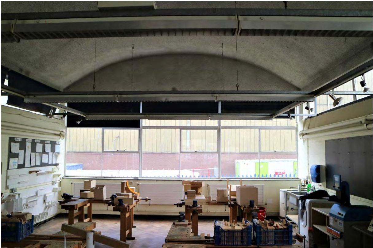
Fig 70 Building 5, looking west
