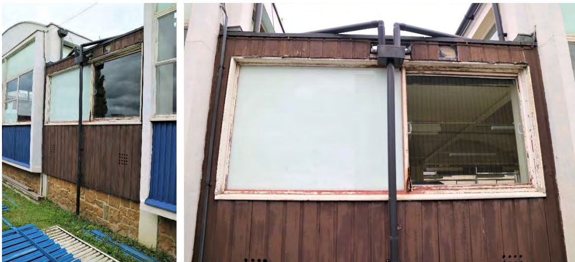
Fig 30 The partition between buildings 3 and 4. (Left) Looking north-east. (Right) Looking east
