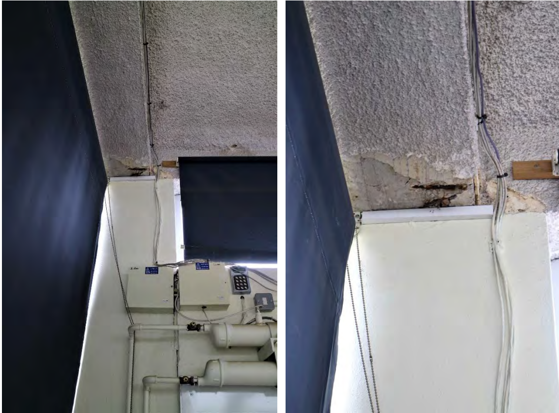
Fig 40 Detail shots of an exposed reinforced concrete beam
