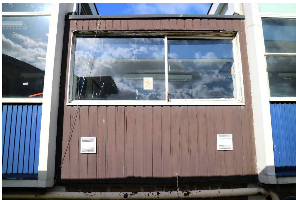
Fig 18 The adjoining partitions between buildings 2 and 3, looking west
