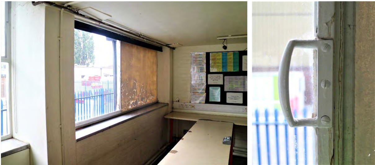
Fig 68 (Left) Sliding window to the north-west of Building 4, looking north-west. (Right) Detail of handle
