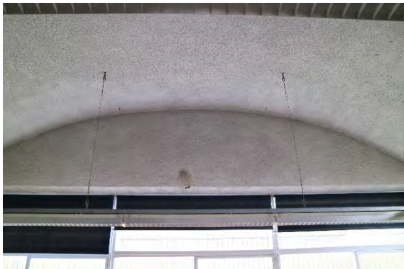
Fig 39 Detail shots of the sound proof cement render ceiling
