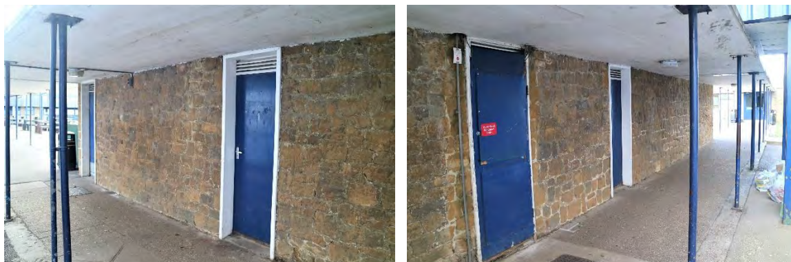
Fig 22 The north elevation. (Left) Looking south-east. (Right) Looking south-west
