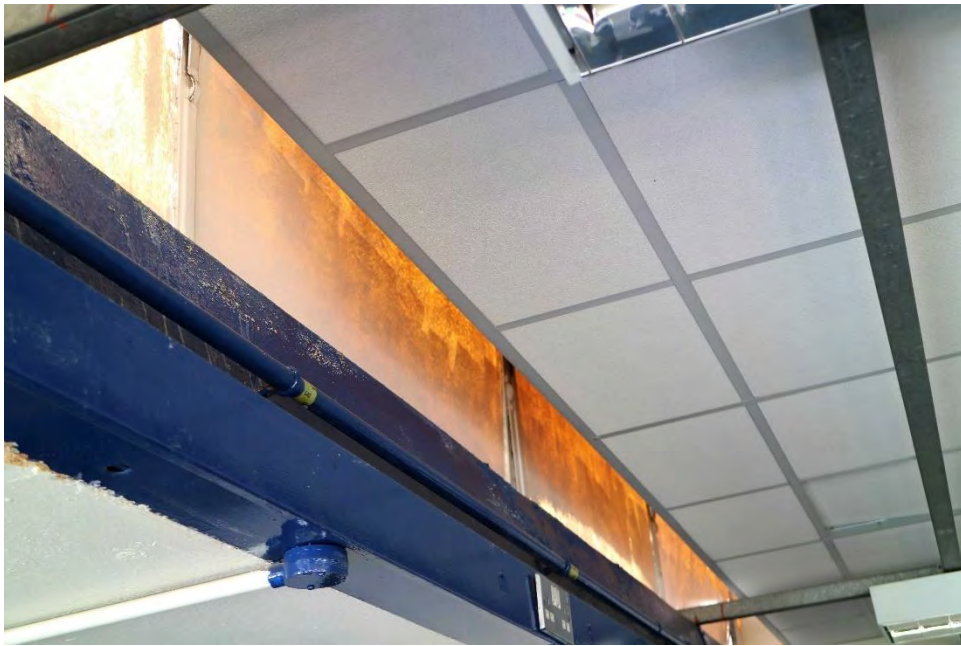
Fig 53 The southern crittall window of Building 2, looking south-west
