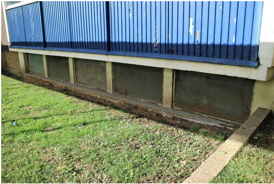
Fig 19 The basement windows underneath Building 1, looking south-west
