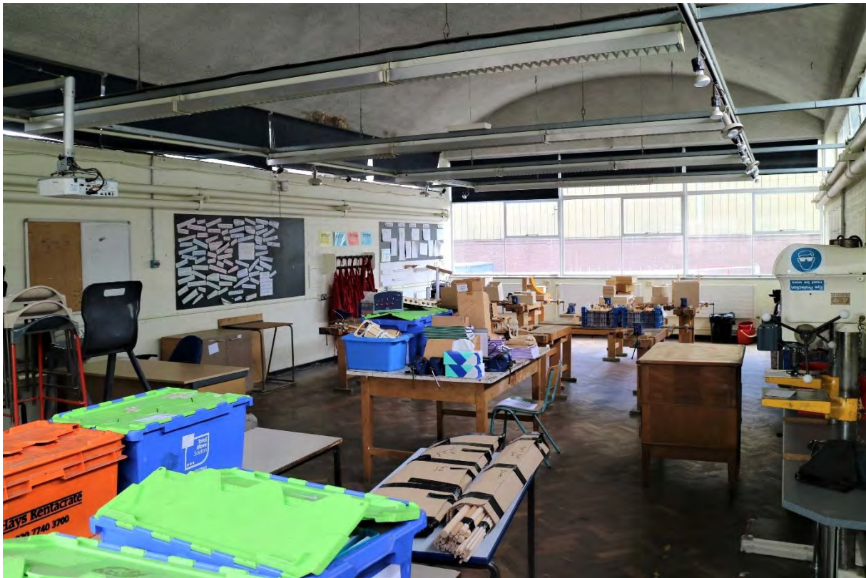
Fig 72 Building 5, looking south-west
