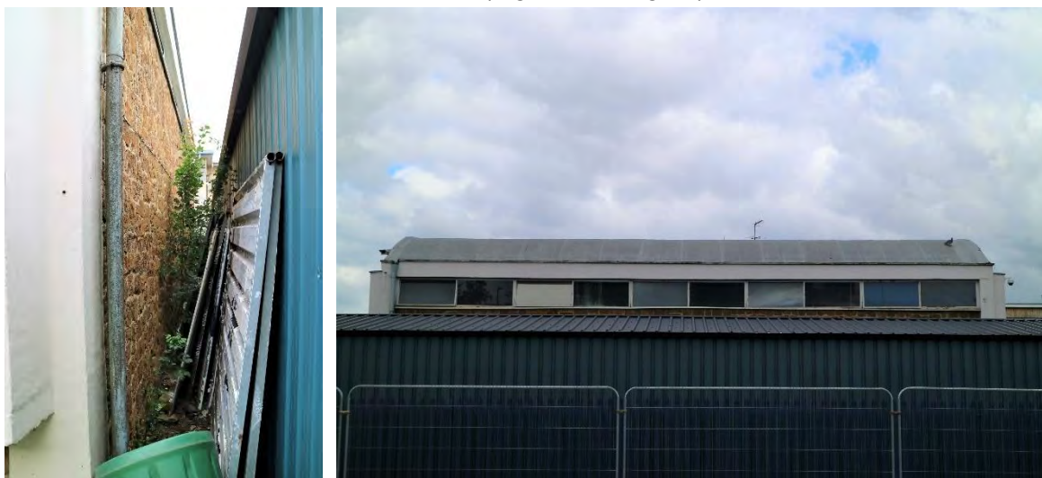
Fig 33 The south elevation. (Left) Looking east. (Right) Looking north
