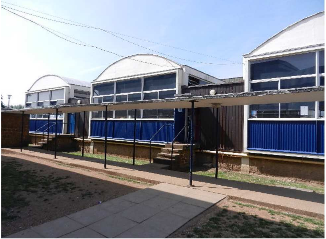
Existing Eastern Elevation of Block B.
