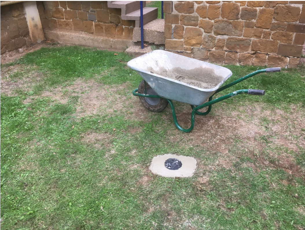
Plate 5. Installation of WS2
