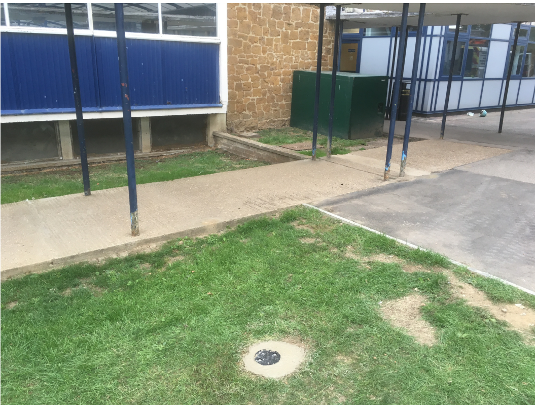
Plate 6. Installation of WS1
