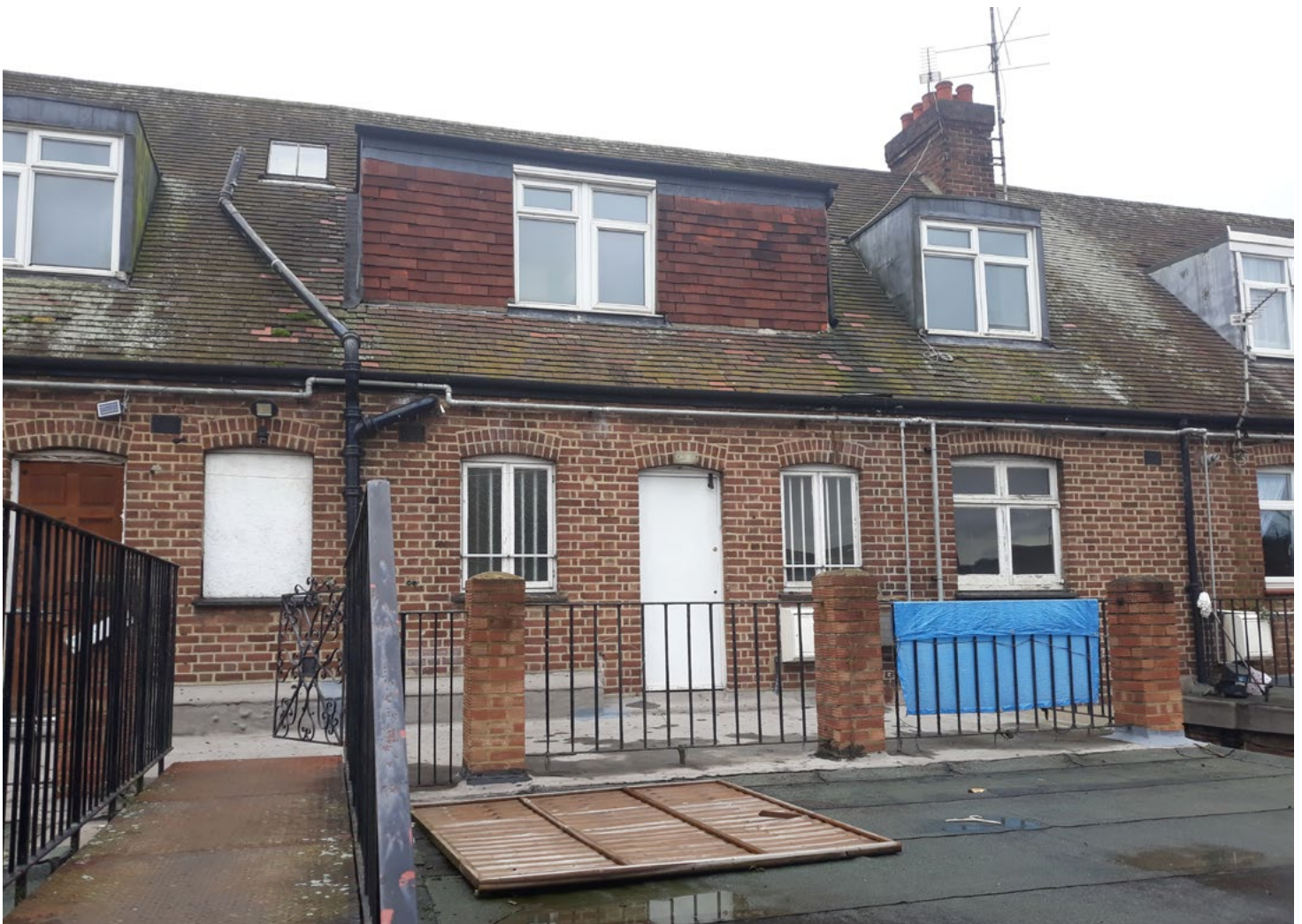
Photo of existing rear elevation showing the two existing dormers and the terrace above ground floor shops.
